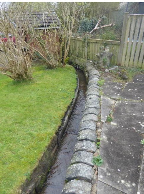
Vertical stone lined channel looking east.
