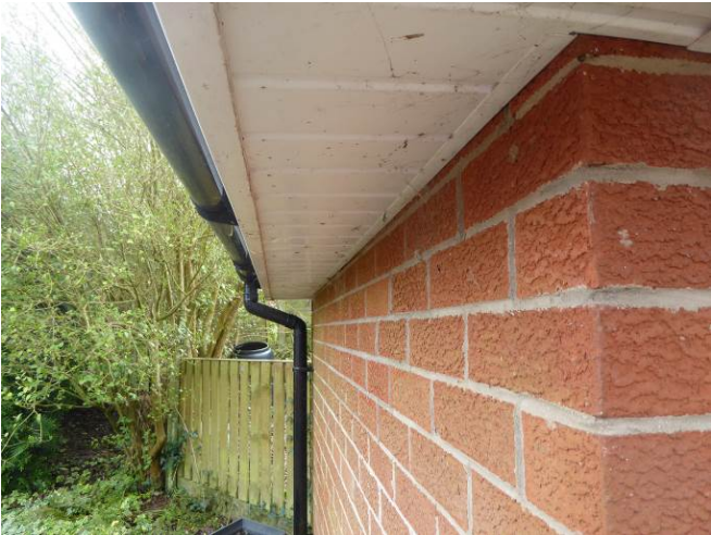
Detached outbuilding showing tight fitted soffits to brickwork.
