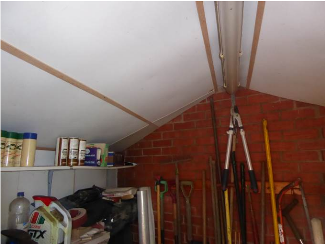
Detached outbuilding showing boarded roof below concrete tiles.
