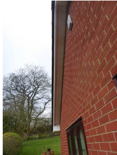
Bungalow, showing southern gable elevation, soffits are tight to the brickwork.
