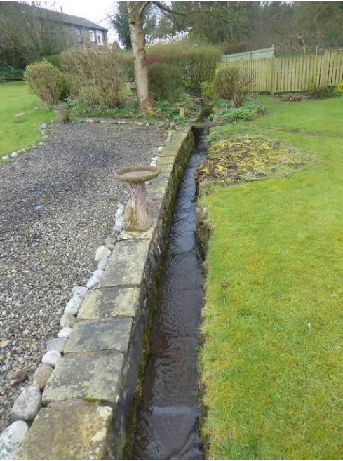
Vertical stone lined channel looking west.
