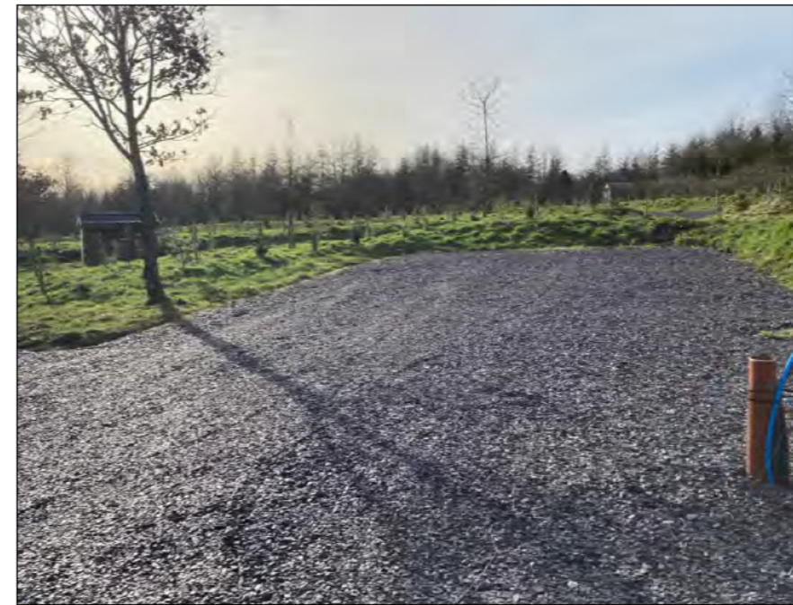
Photograph showing unoccupied caravan pitch with FOUL only pop up
