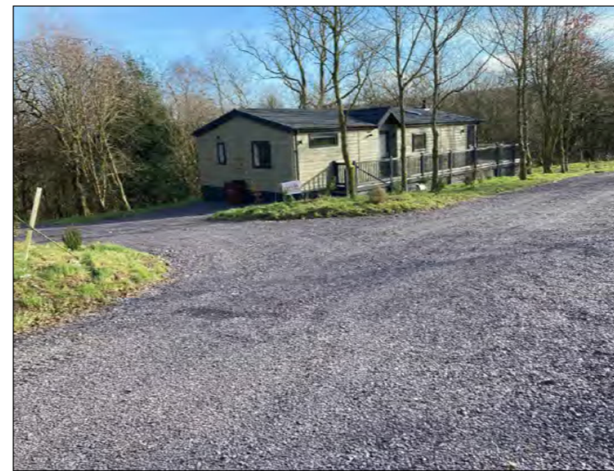
Photograph showing unbound gravel access track
