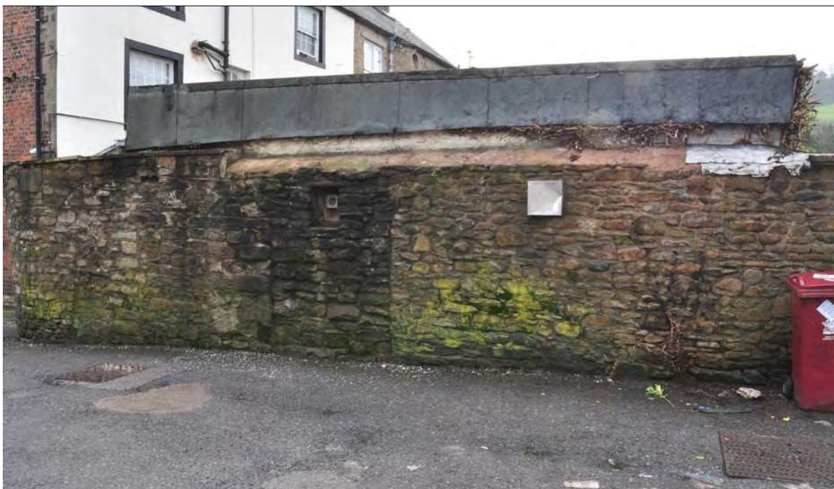
Photo 2: North wall, with blocked opening to be retained. Note unsightly felt roof covering and mortar coping. (Photo taken Feb 2021)
