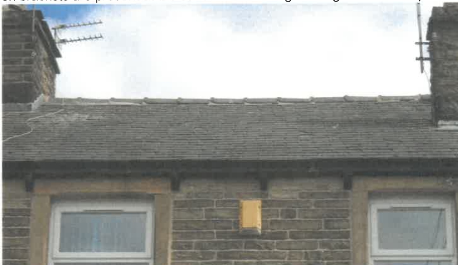
Main roof front pitch
