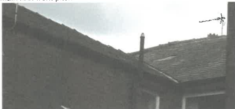
Rear roof pitch and outrigger
