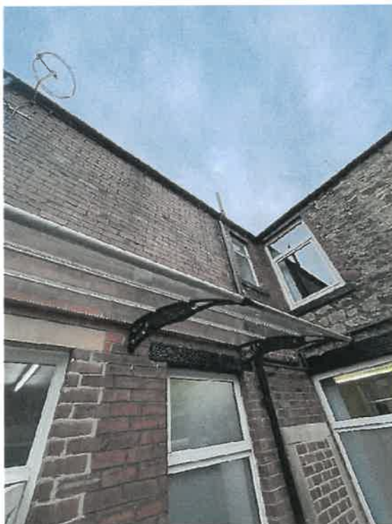
Rear two storey element is constructed in facing brick and is assumed to have been constructed as part of the original build. Various alterations have been made with regards new and bricked up existing window openings, along with a modern canopy.
