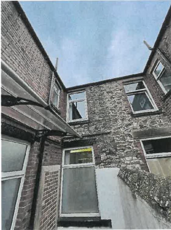
Rear Elevation constructed in stone and brick. Windows white upvc.
