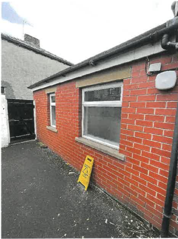
Rear single storey element appears to be more modern. With more recent looking facing brick.
