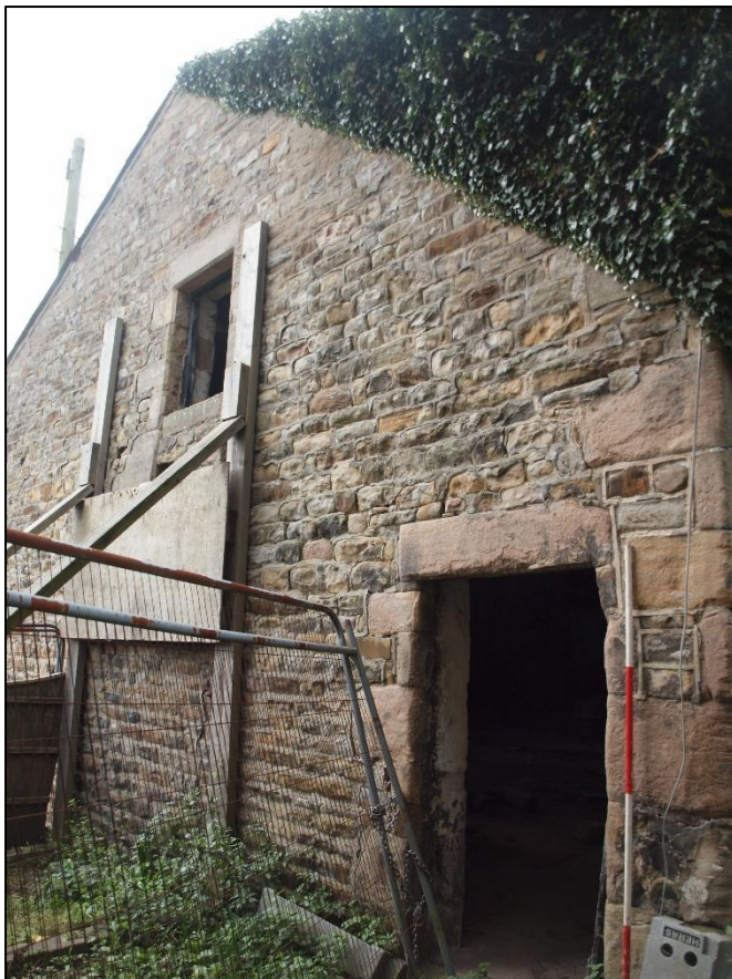
Plate 18: Gable showing northern doorway
