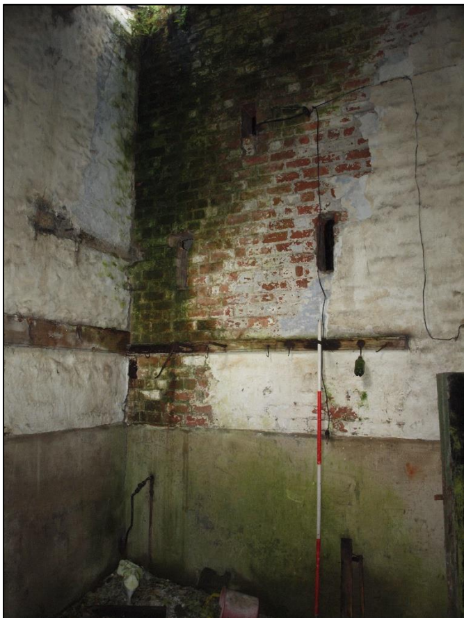
Plate 80: Inserted brick wall with ventilation slots to first floor
