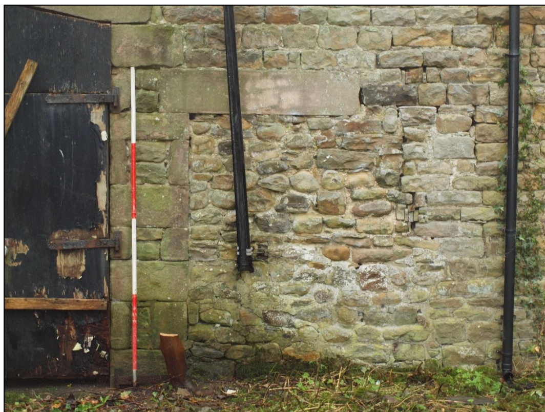
Plate 26: Detail of blocked doorway
