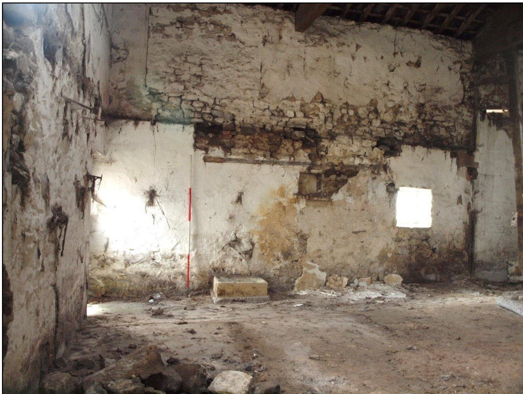
Plate 46: Eastern end of south wall showing blocked first floor window and ground floor niche
