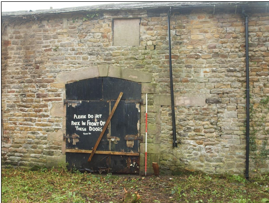
Plate 24: Barn door with pitching eye over and blocked doorway to the right
