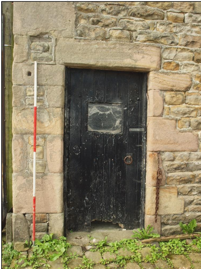
Plate 16: Doorway to southern end of gable
