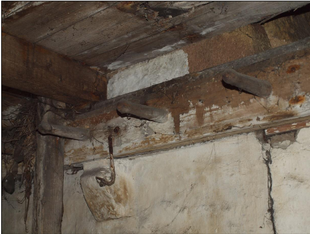
Plate 71: Timber beam along east wall with timber pegs and iron hooks
