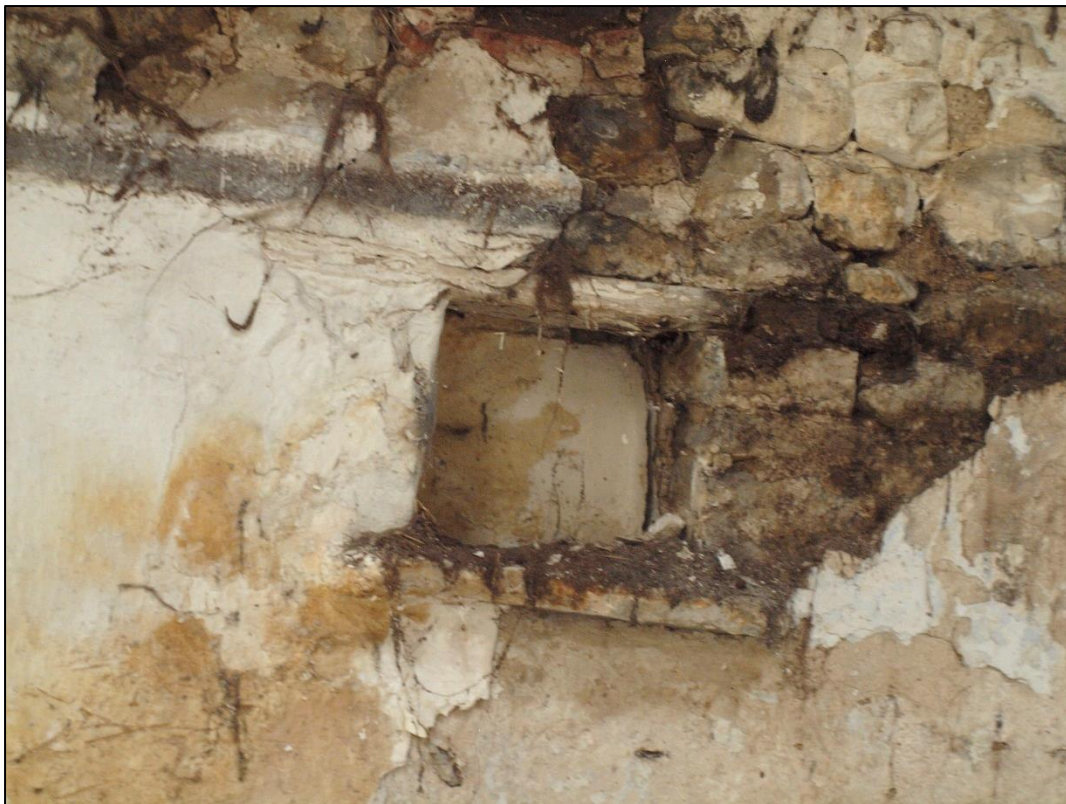
Plate 48: Detail of niche
