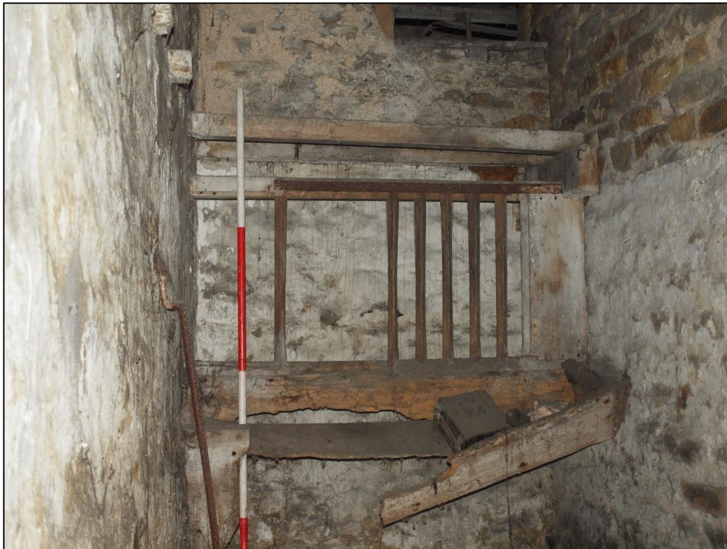
Plate 65: Detail of timber feeding trough
