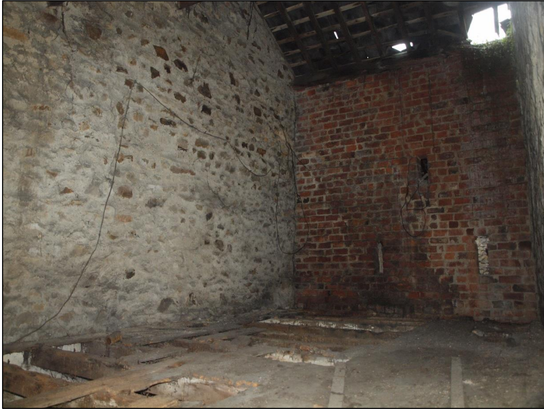
Plate 75: First floor of extension showing brick wall to the north
