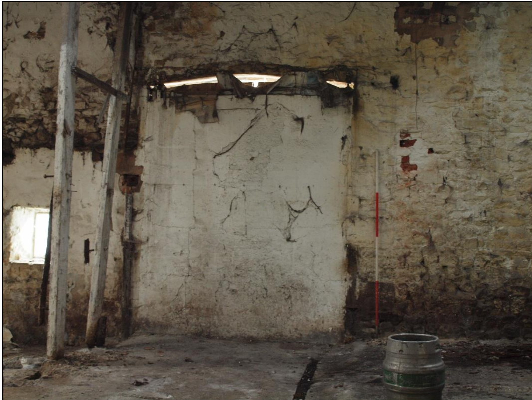
Plate 51: Southern barn door blocked with concrete block
