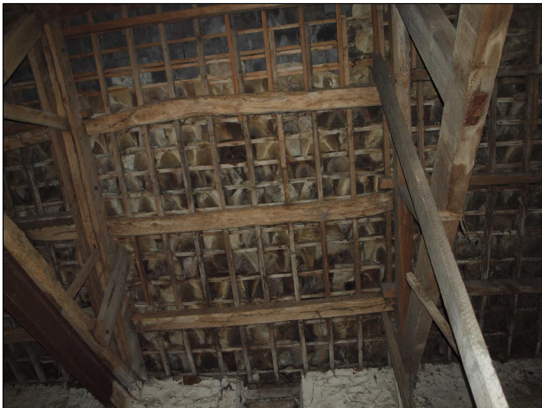
Plate 63: Roof showing remaining hand cut purlins
