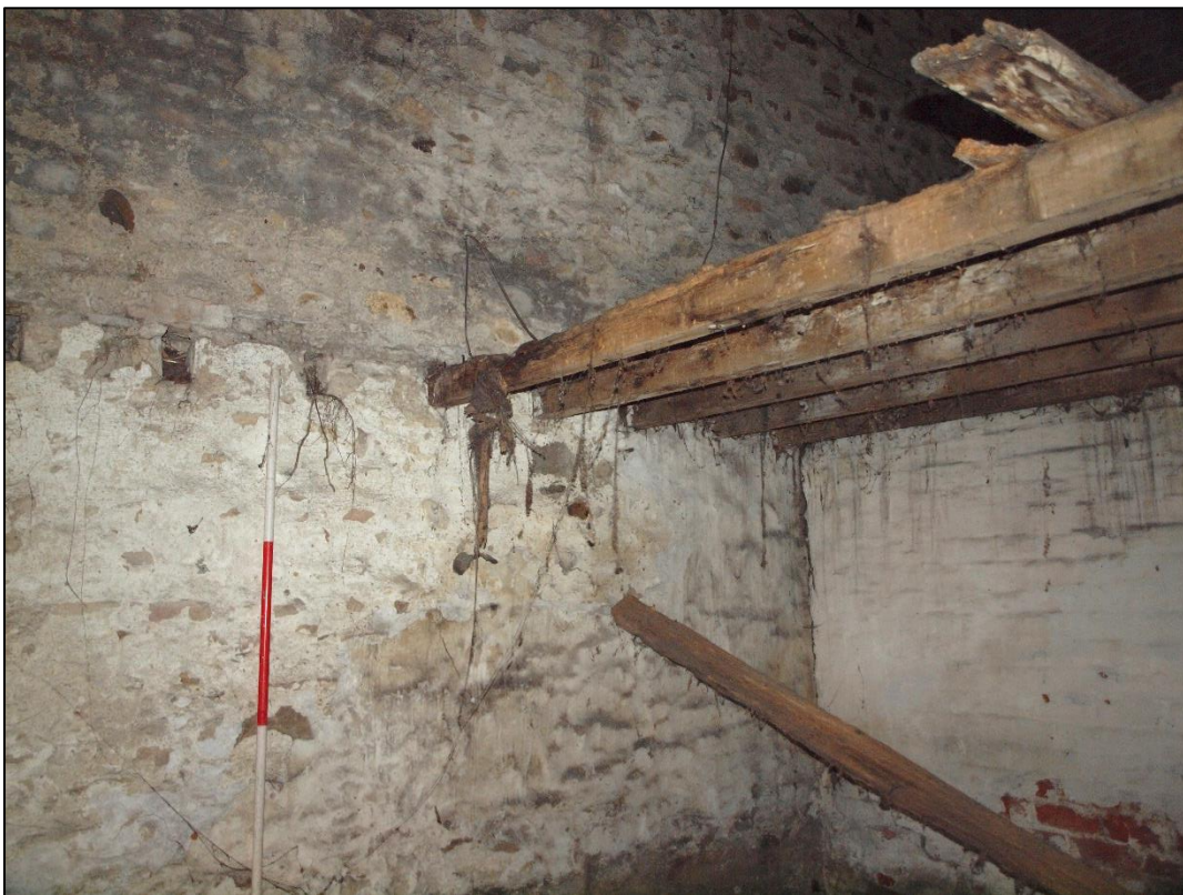
Plate 72: Joist holes and remaining first floor
