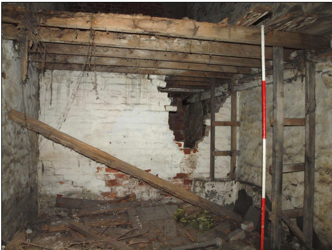
Plate 68: Southern room of west extension
