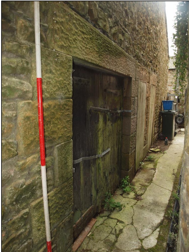
Plate 37: Wide loading doorway at northern end
