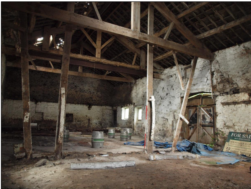
Plate 40: General shot of interior looking west
