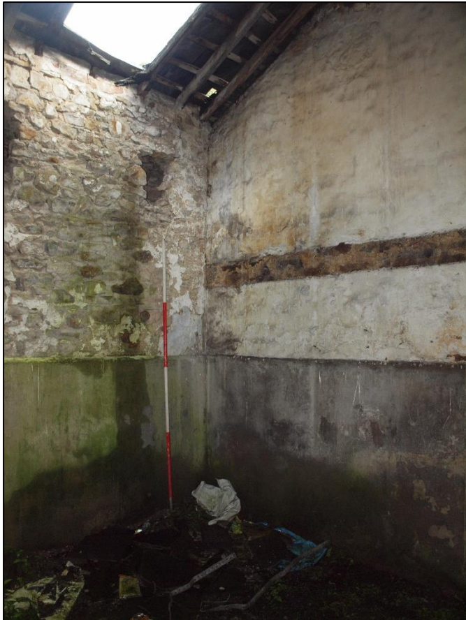
Plate 79: Cement render with whitewashed brick over
