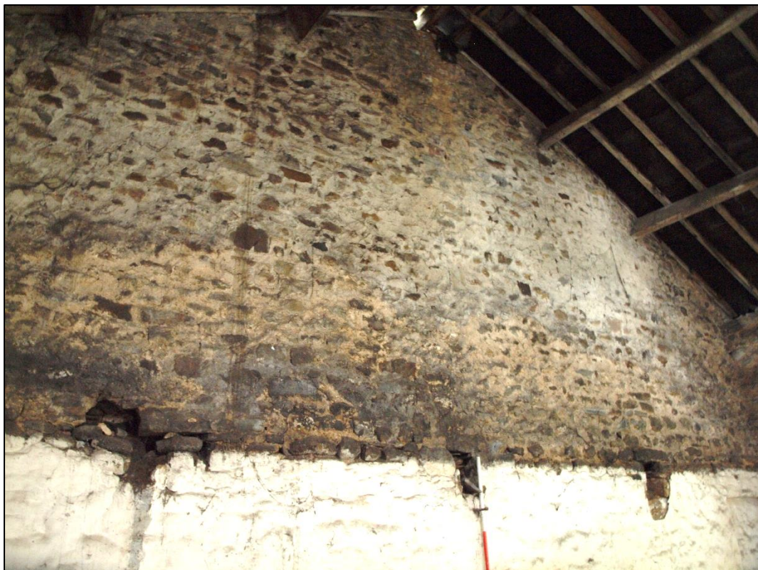
Plate 59: Detail of removed first floor joist holes an first floor of gable
