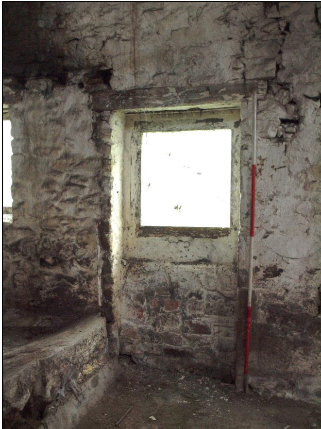
Plate 55: Blocked doorway with window inserted
