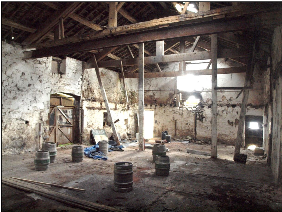
Plate 42: General shot of interior looking east
