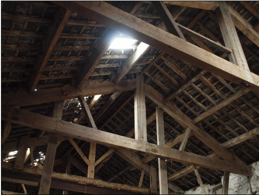
Plate 41: King post trusses
