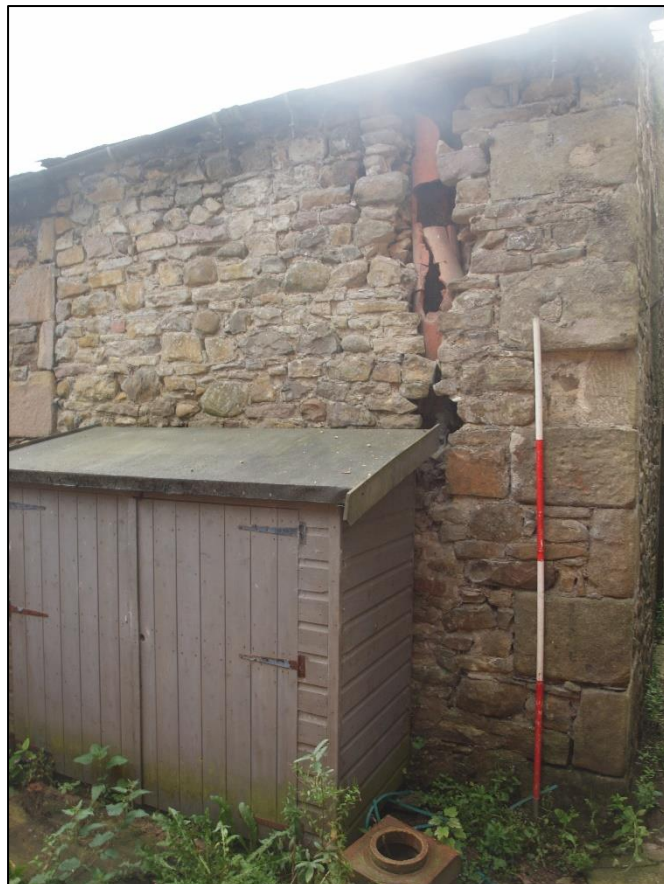
Plate 32: North elevation of extension
