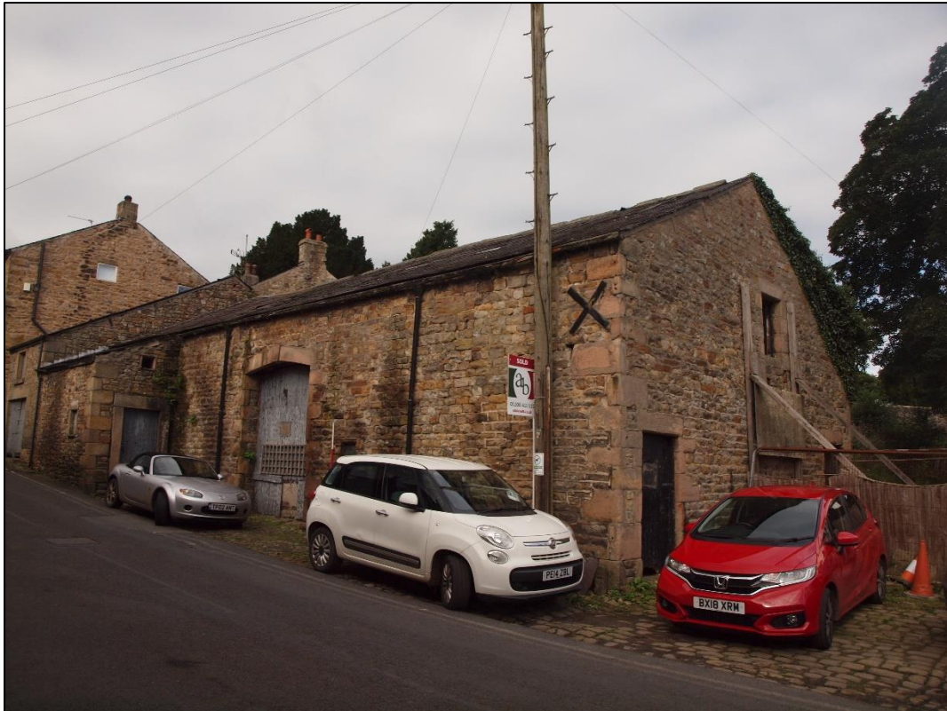
Plate 1: General shot of south elevation from Talbot Street
