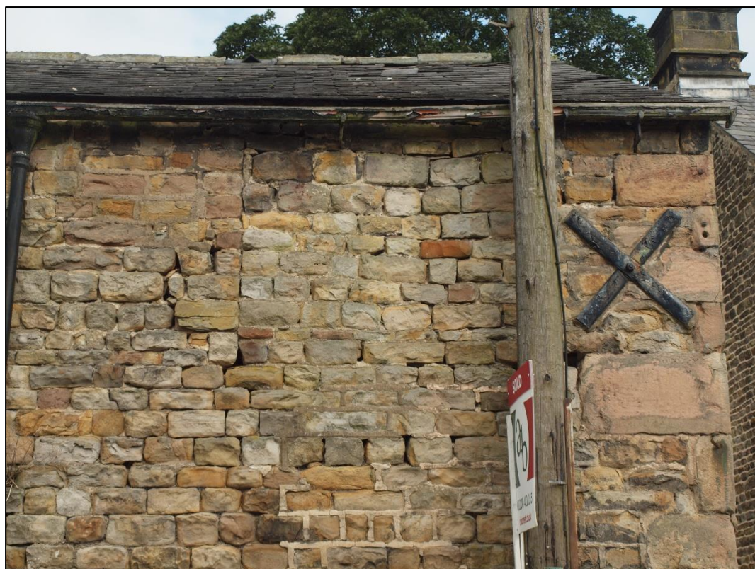
Plate 14: Blocked window at first floor level
