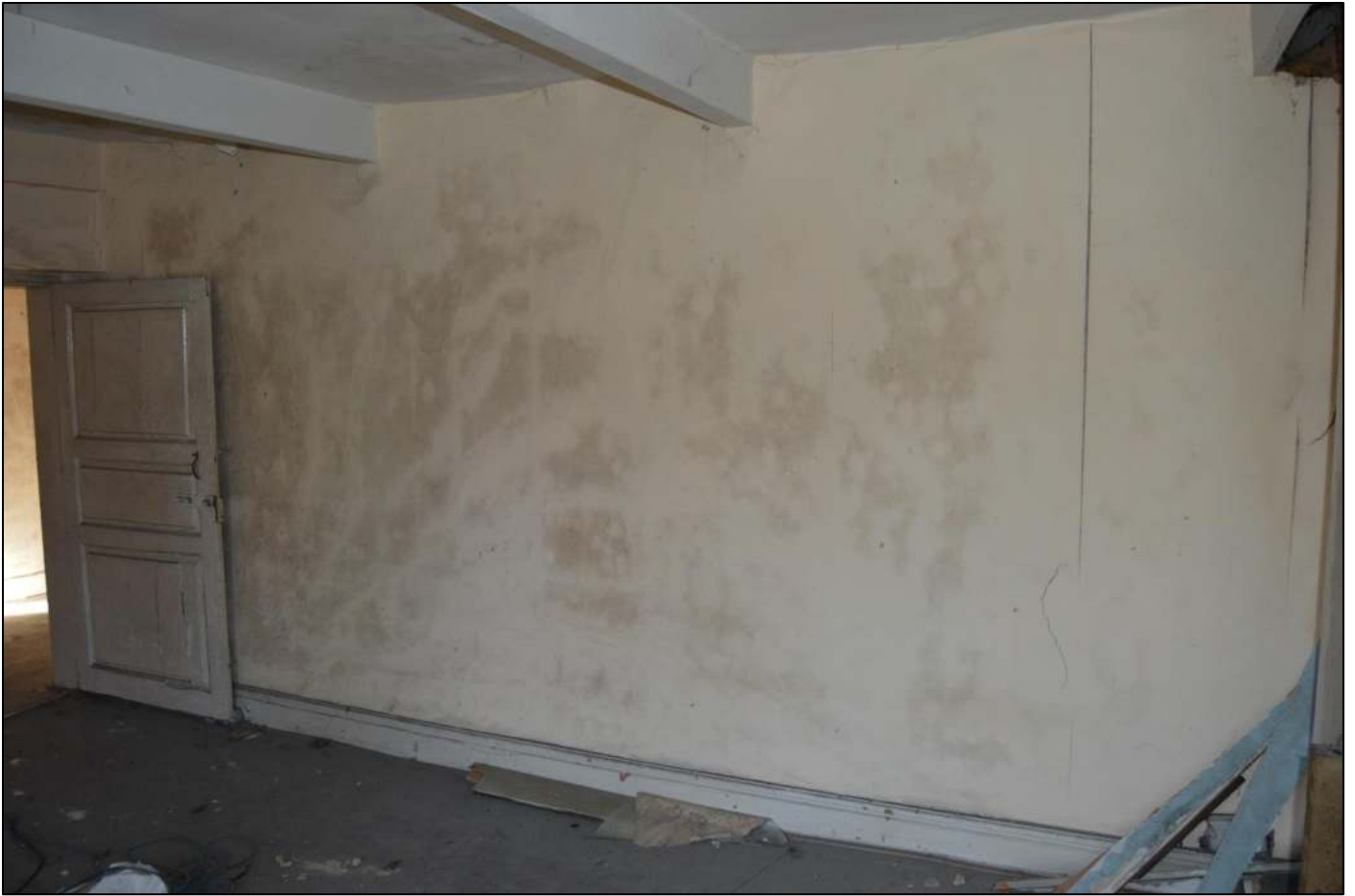
PL57: View north west within the first-floor east unit.
