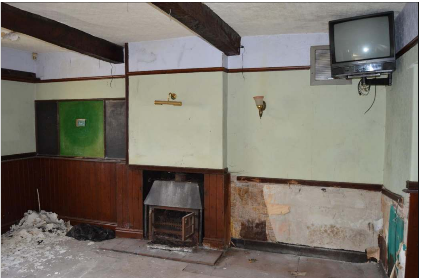
PLI 8: View south west within the ground floor south unit.
