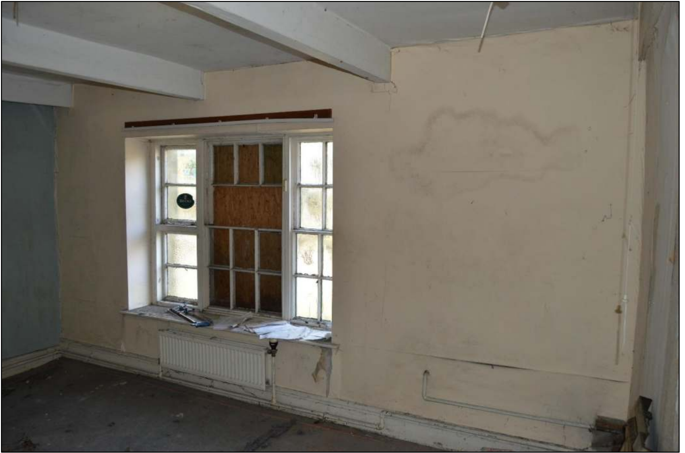
PL59: View north west within the first-floor west unit.
