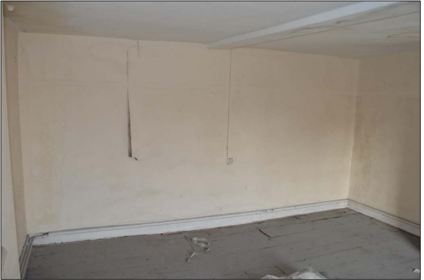
PL49: View north east within the first-floor south unit.
