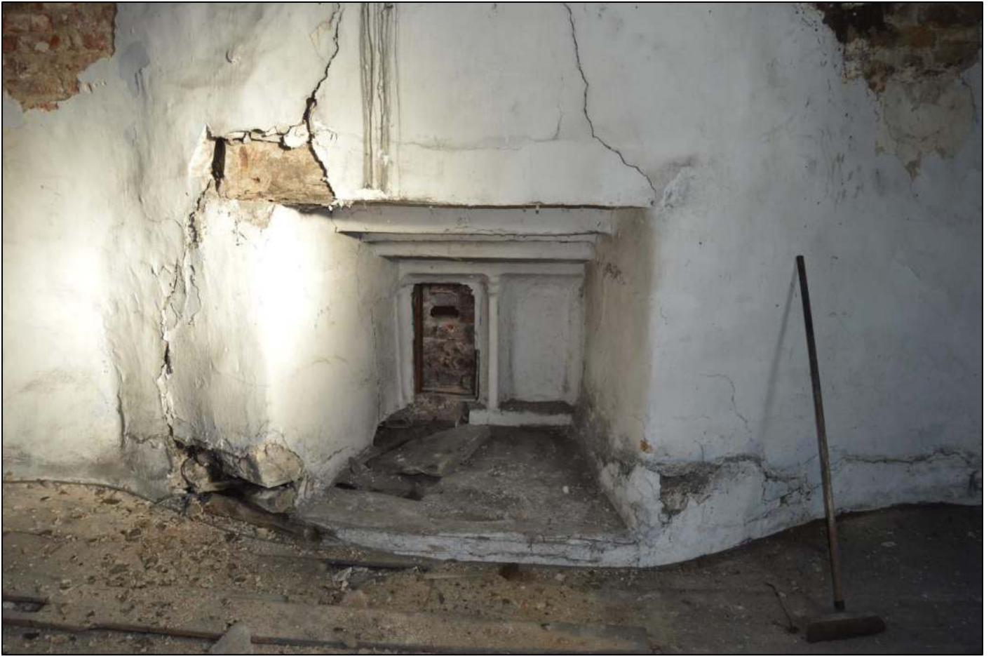
PL67: View of blocked up 17 th century mullion window to the north east wall of the attic.
