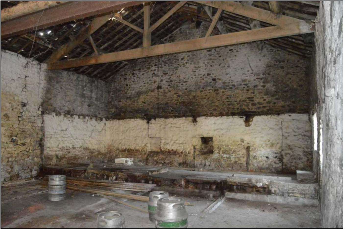
PL85: View of the barn interior from the north west.
