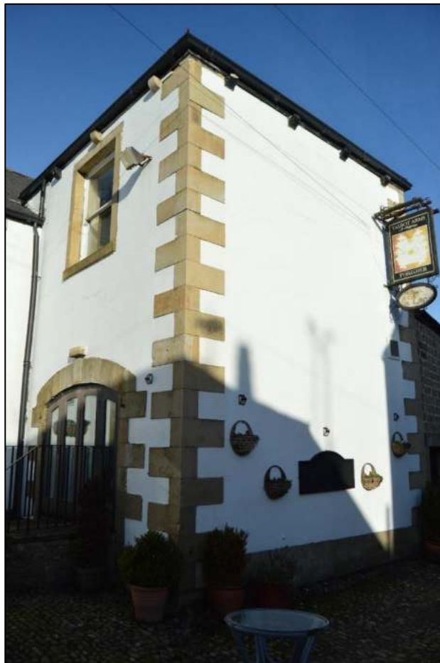
PL04: View of the 19 th century coach house addition from Talbot Street.
