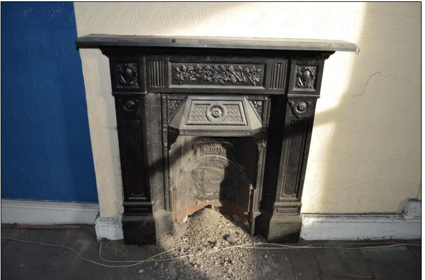
PL56: View of the fireplace to the first-floor east unit.
