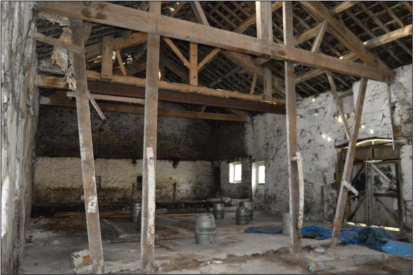
PL83: View of the barn interior from the north east.
