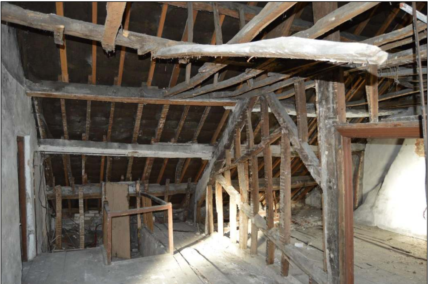
PL66: View north west from the attic landing.
