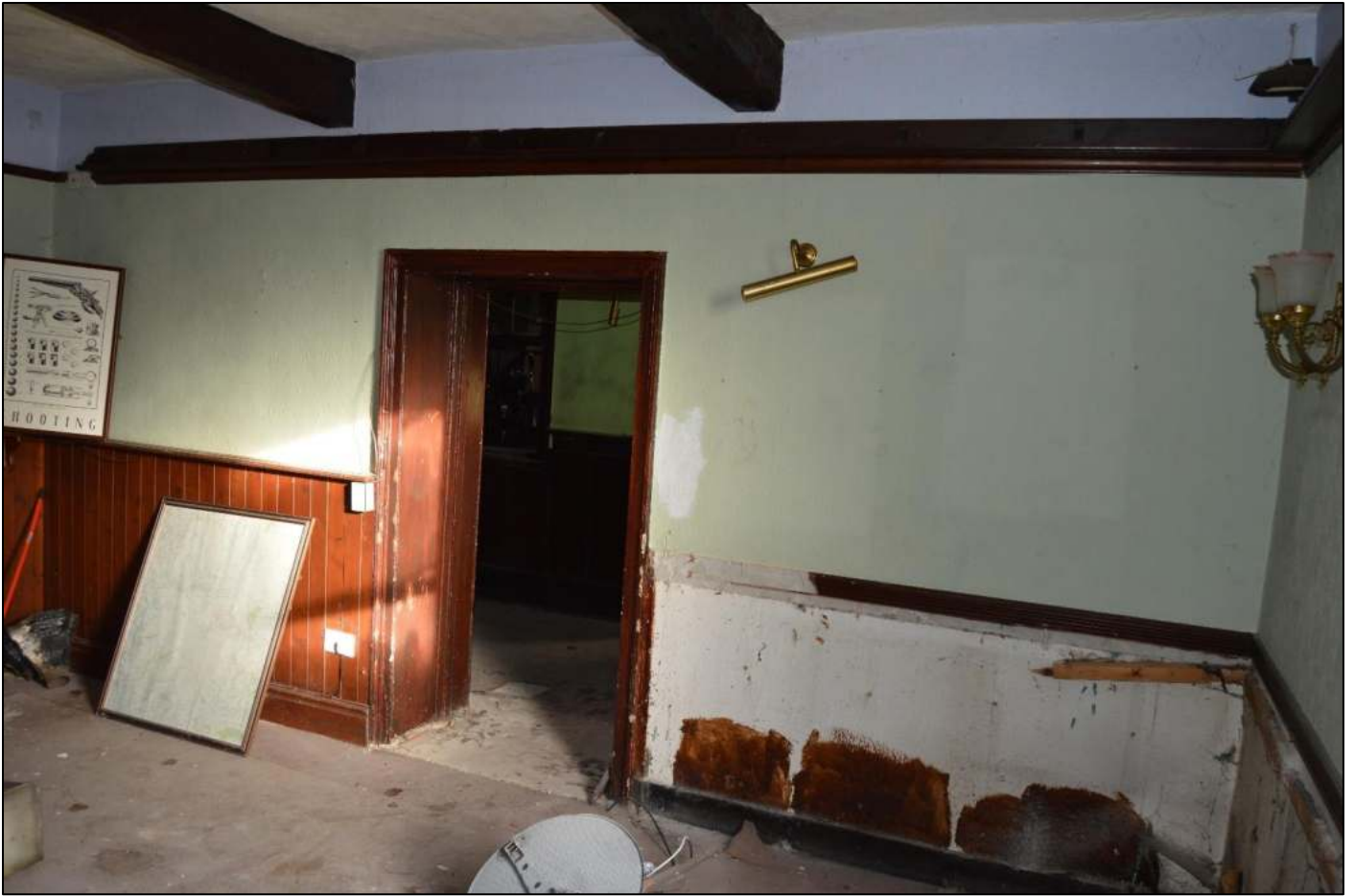
PL19: View north east within the ground floor south unit.
