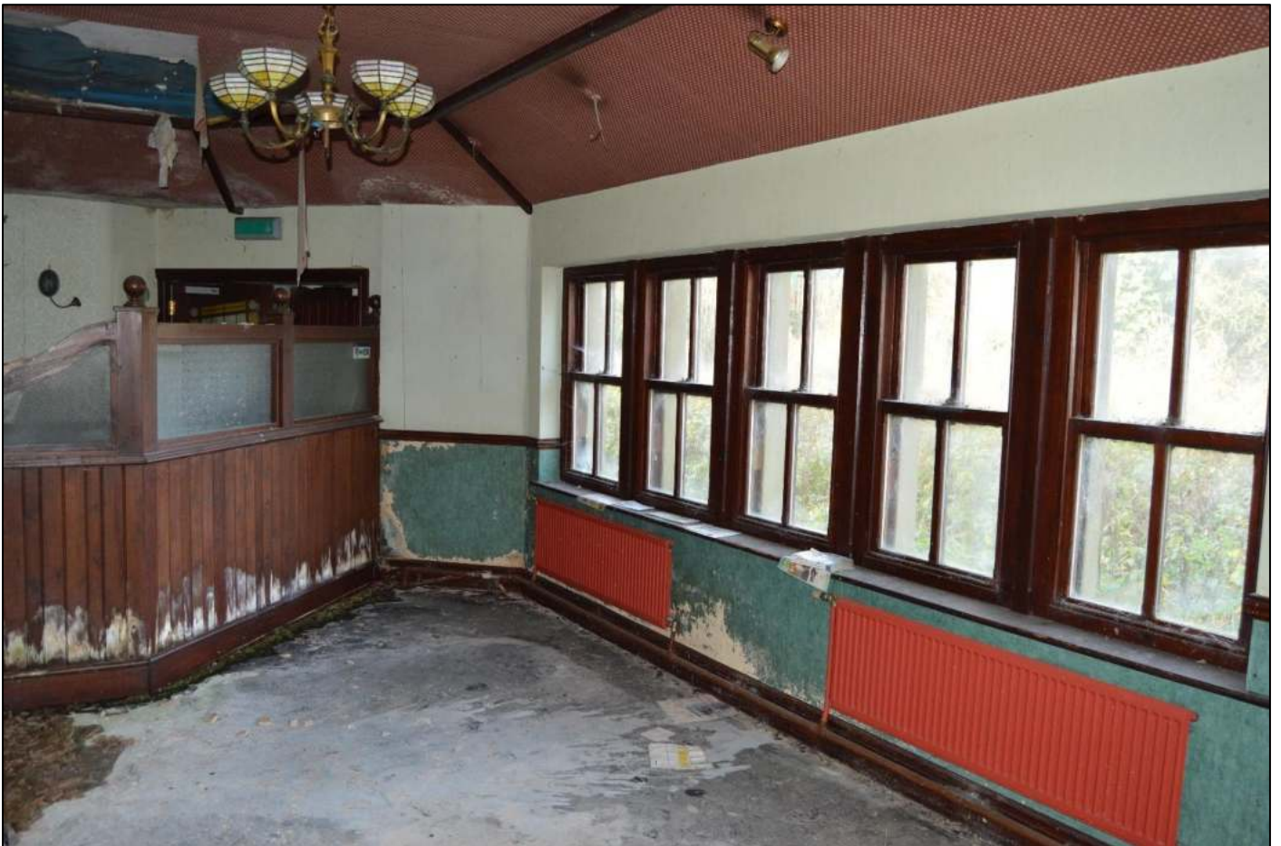
PL32: View south west within the rear extension.
