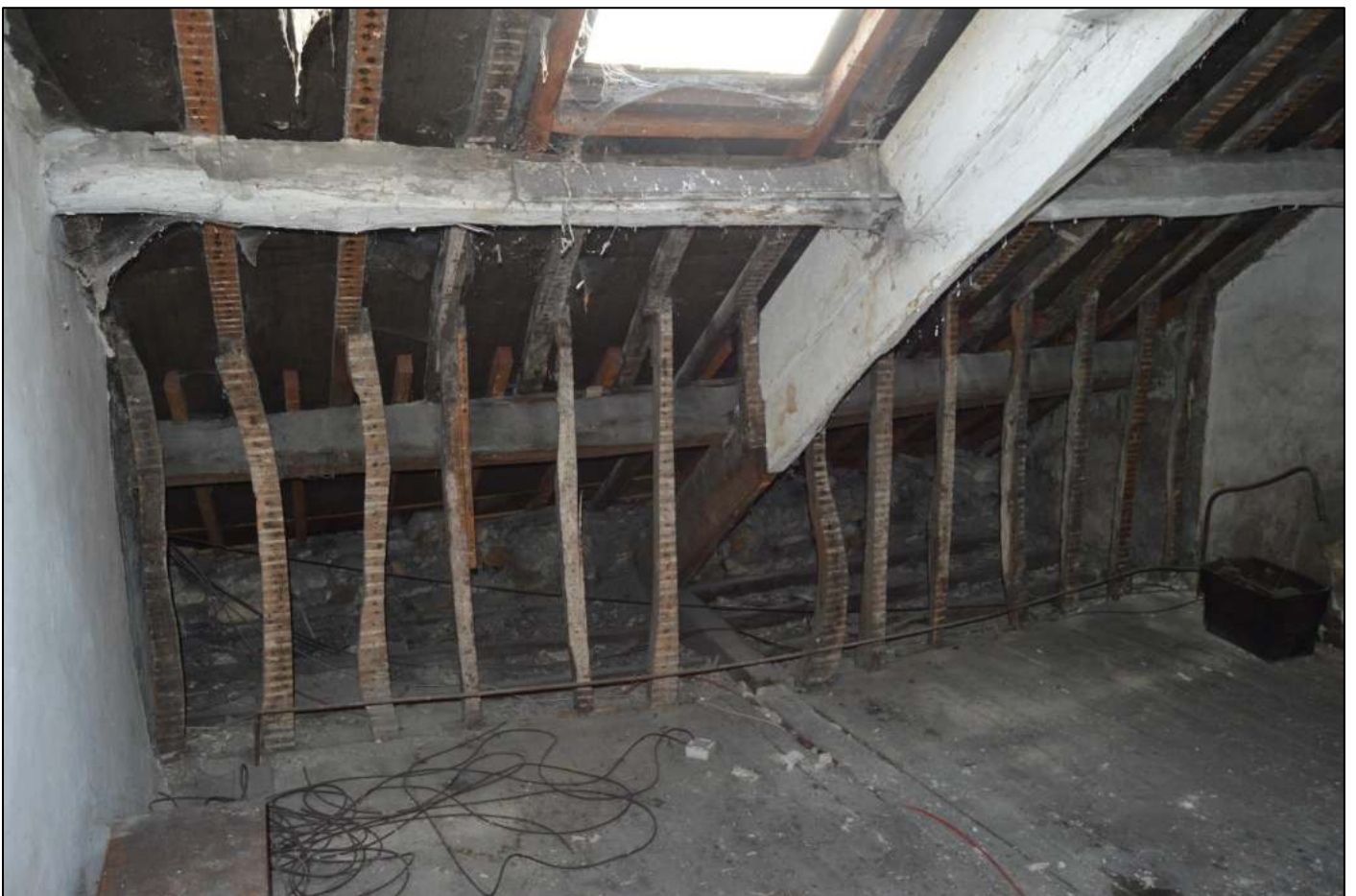
PL70: View south east within the south unit of the attic.
