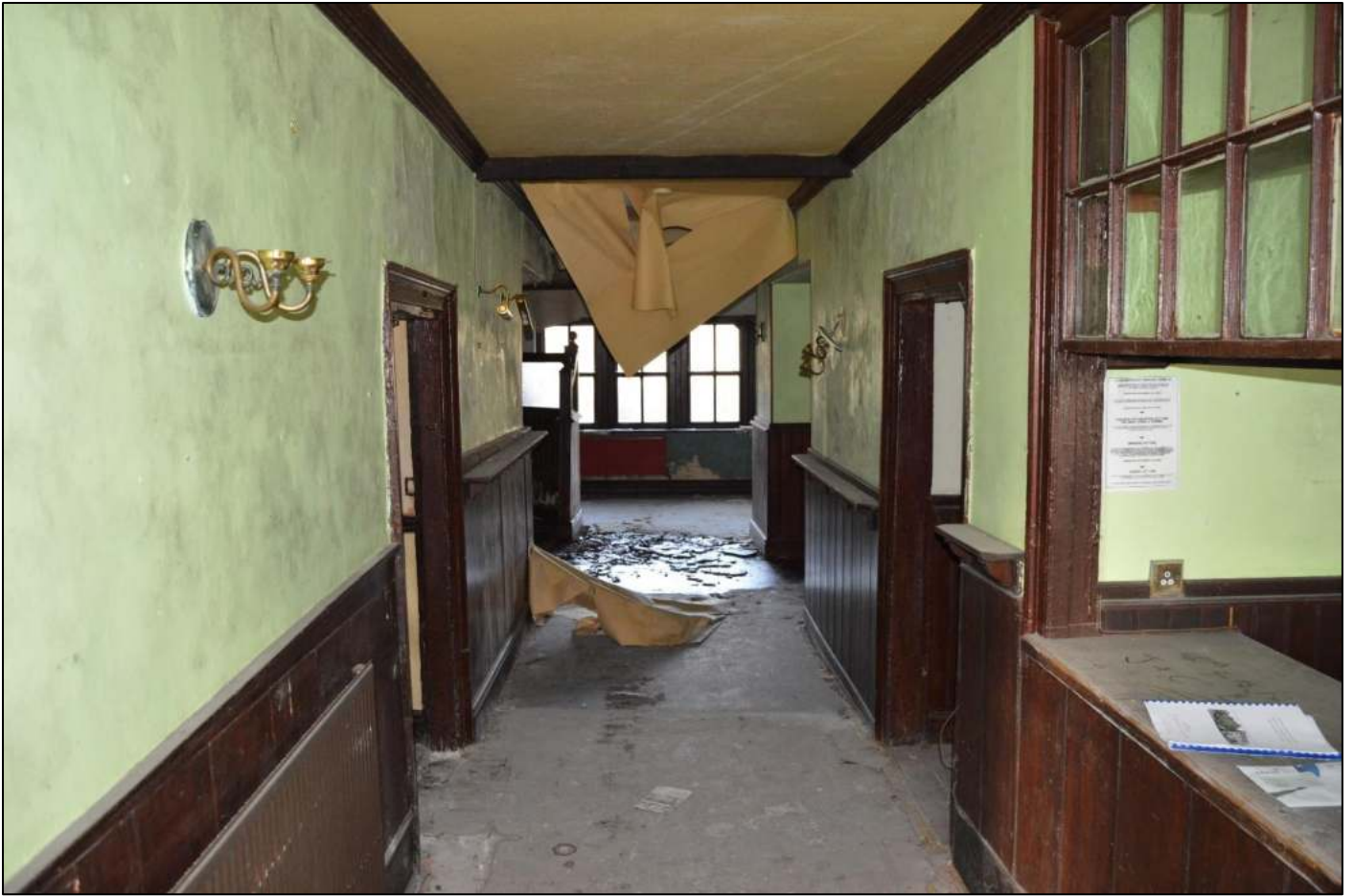
PL25: View north west along the central ground floor passage.
