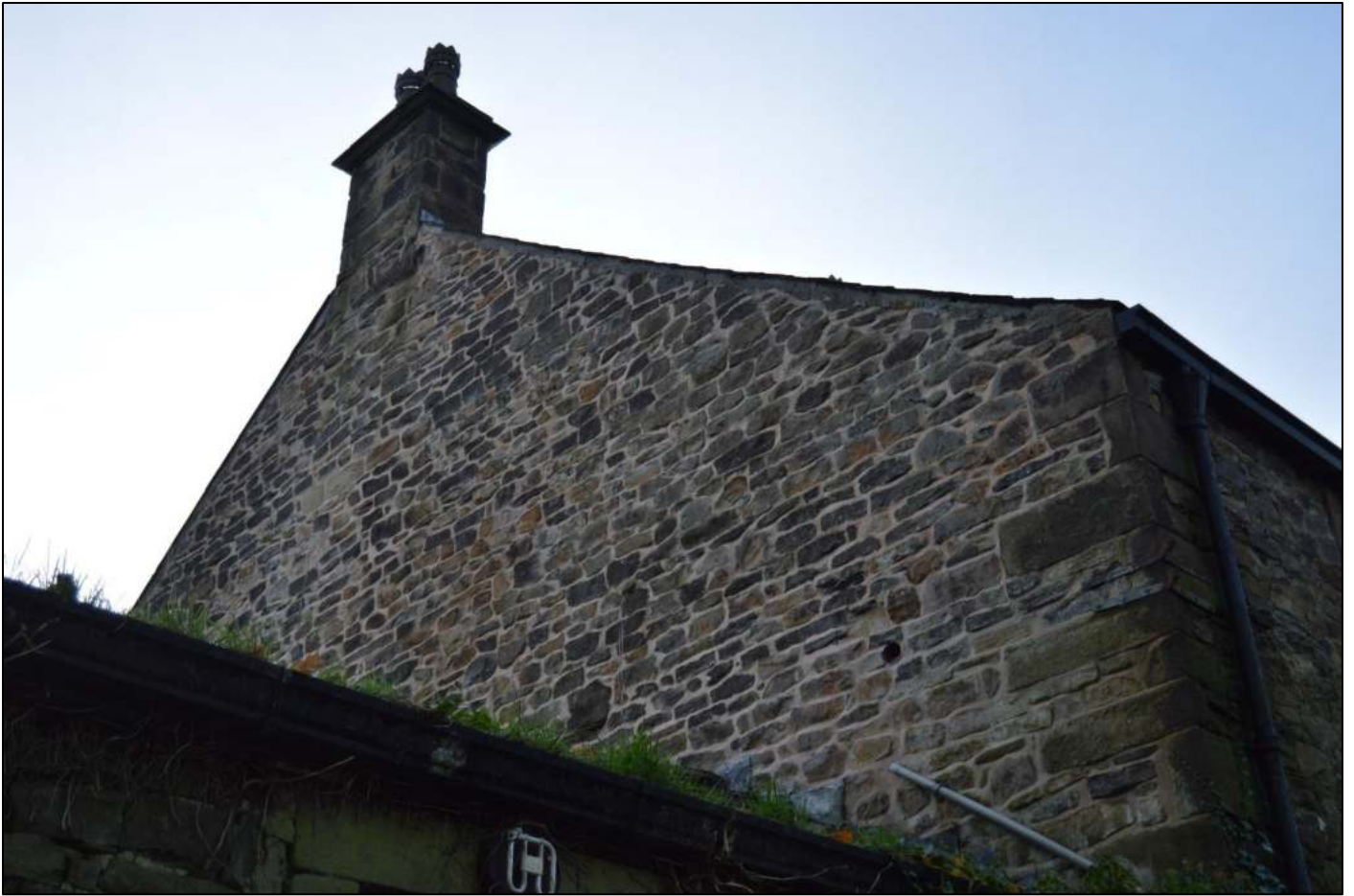
PL15: View of the north east gable end.
