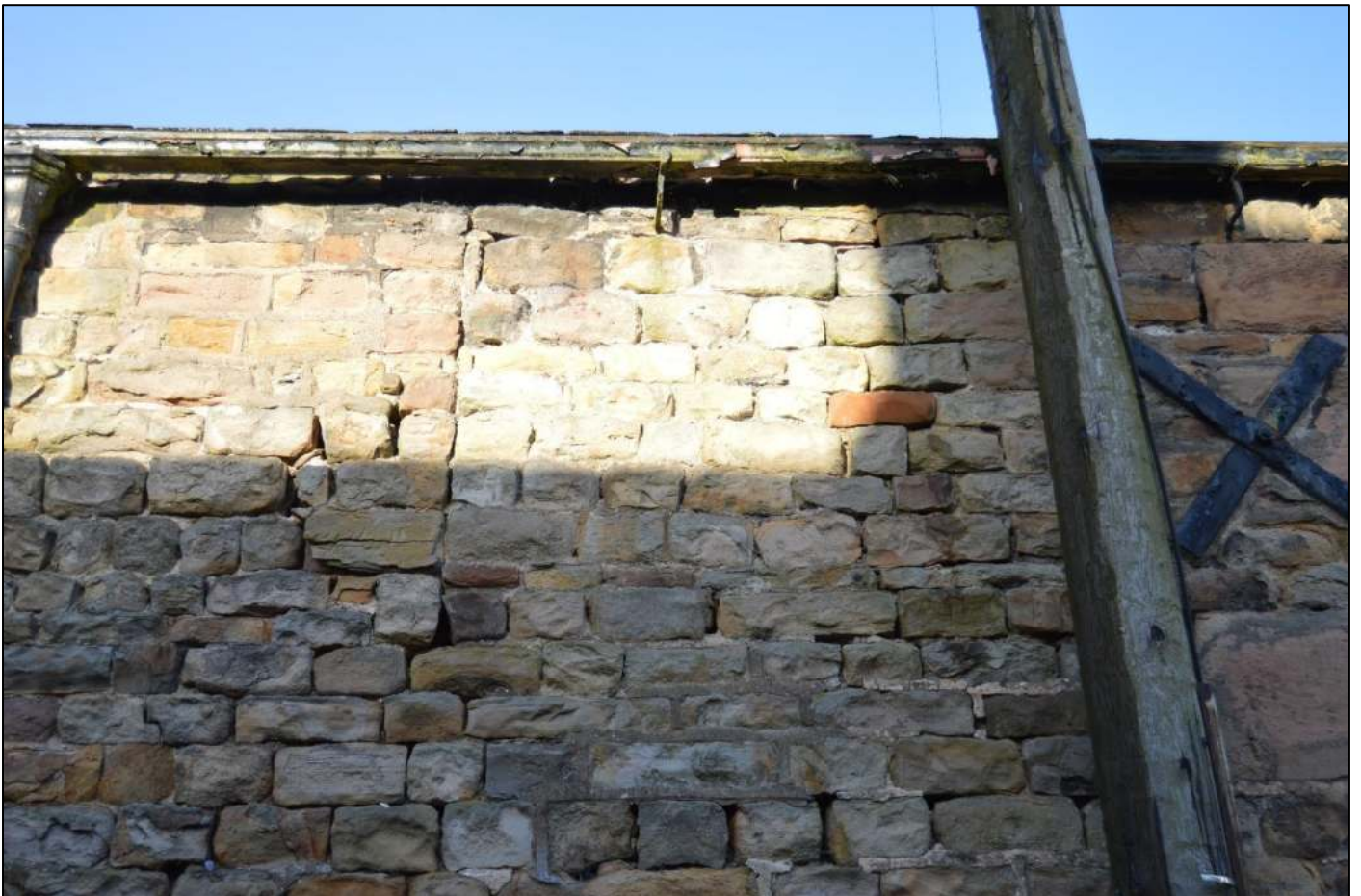
PL74: View of the blocked-up forking hole to the east end of the front south east facing elevation of the barn.
