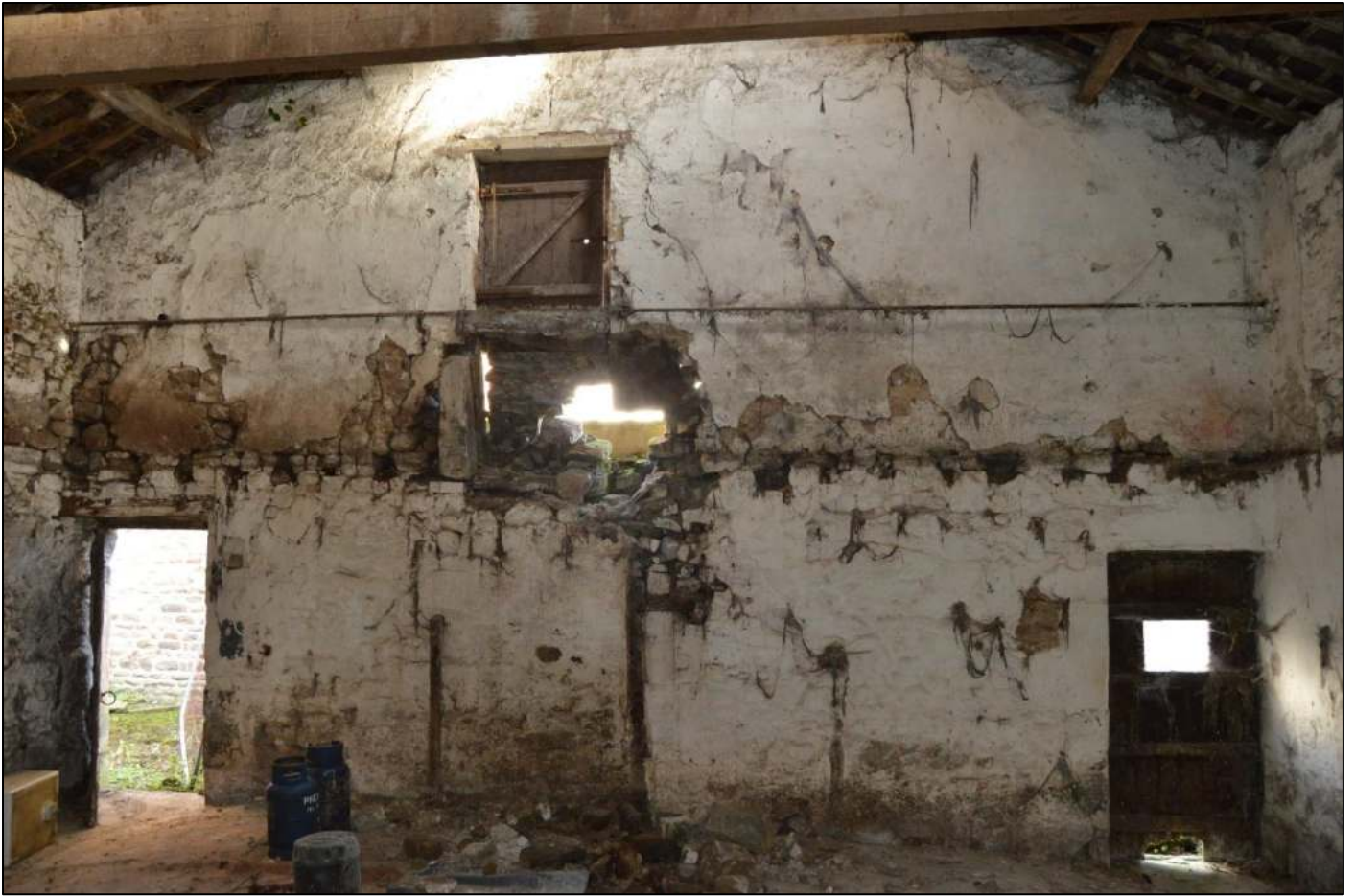
PL87: View of the north east gable end and joist sockets.
