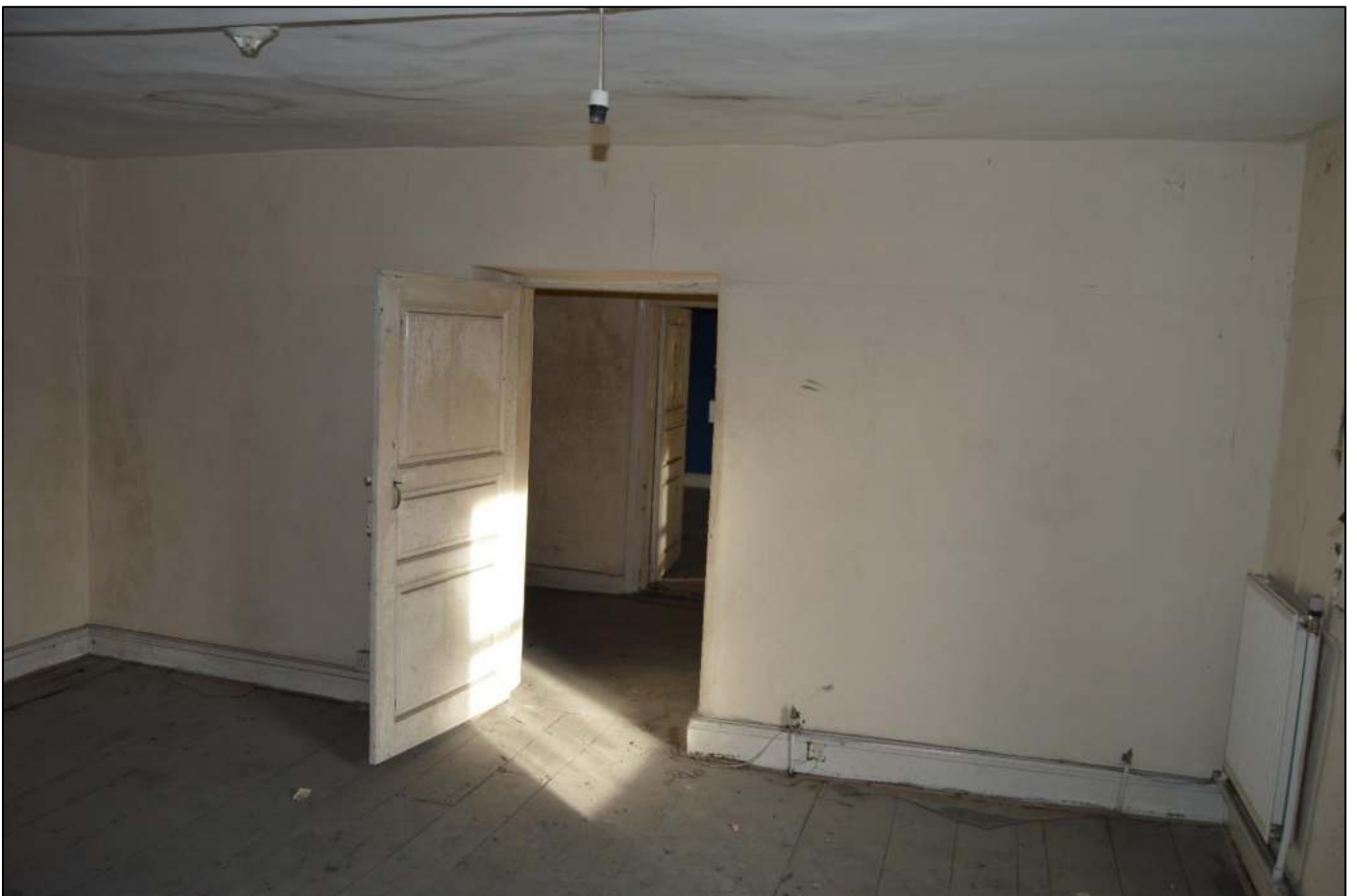
PL48: View north east within the first-floor south unit.
