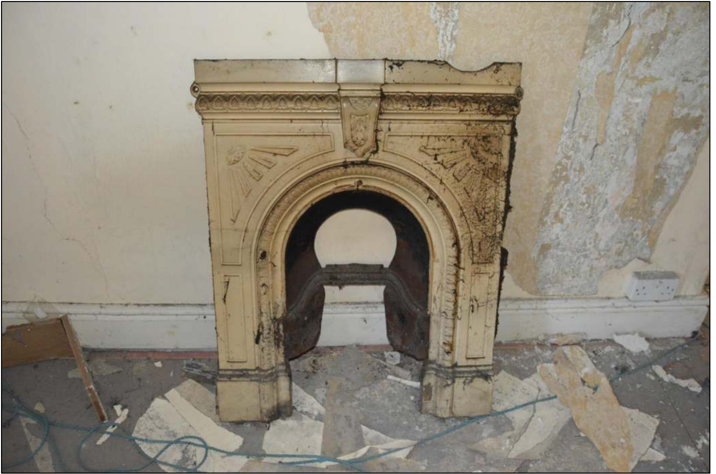
PL61: View of removed fireplace surround to the first-floor west unit.
