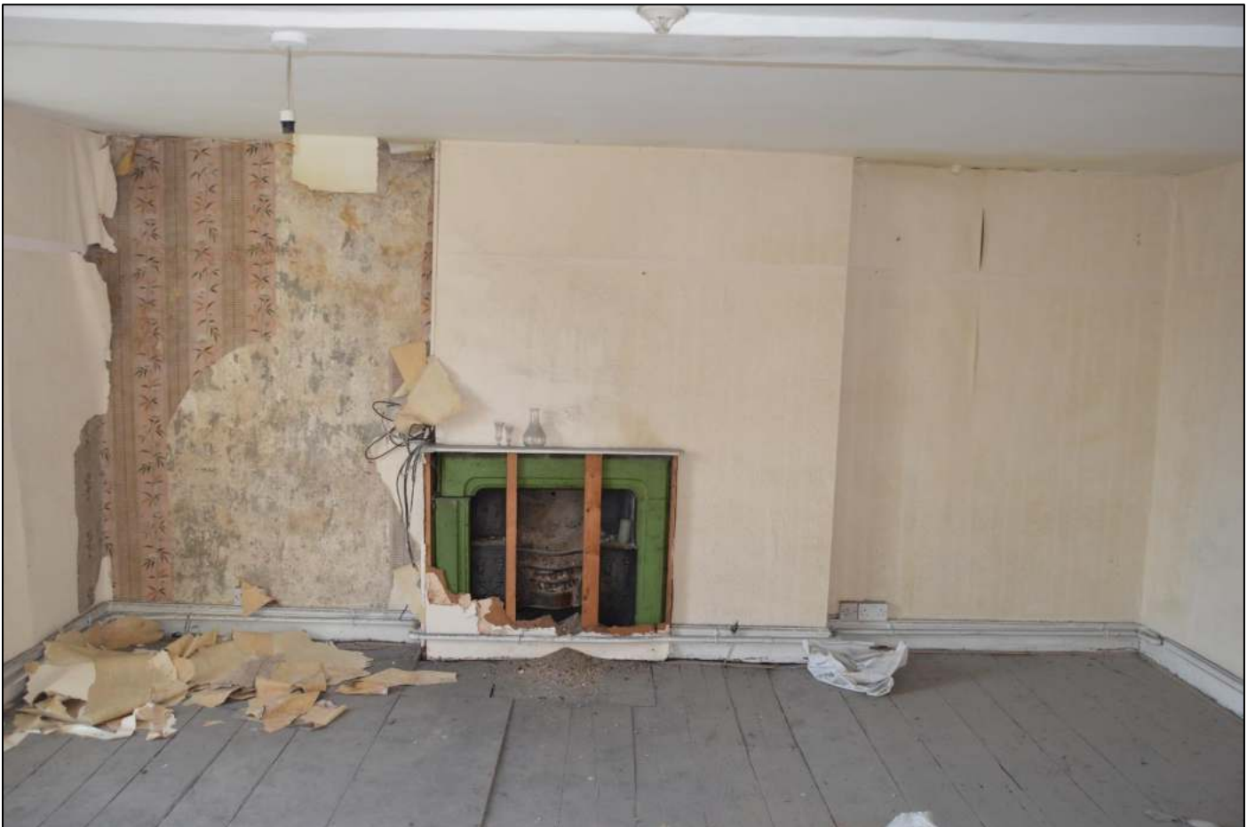
PL50: View south west within the first-floor south unit.
