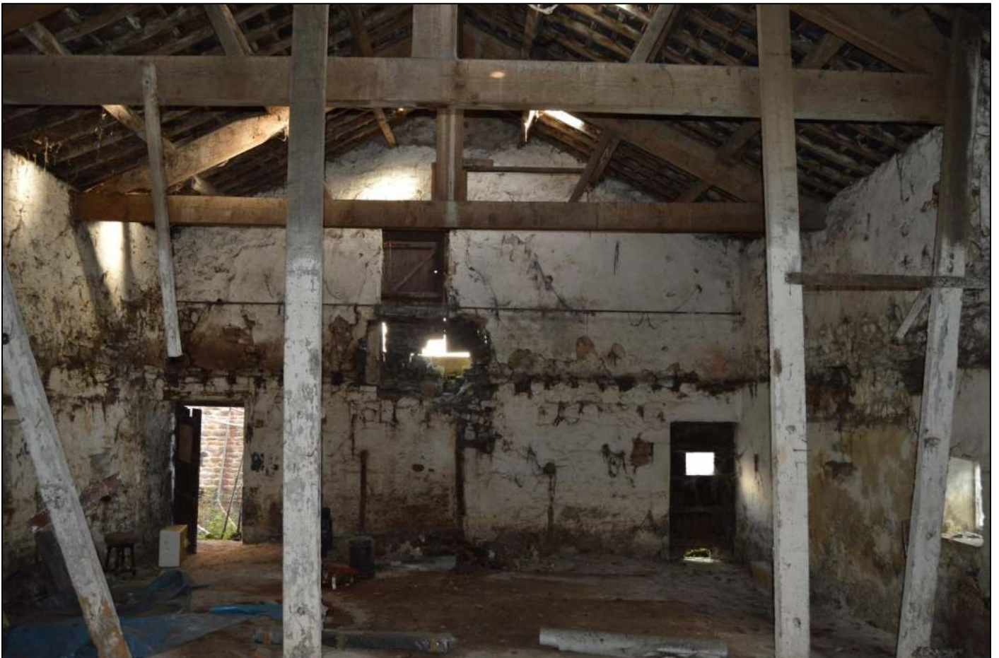
PL86: View of the barn interior from the north east.
