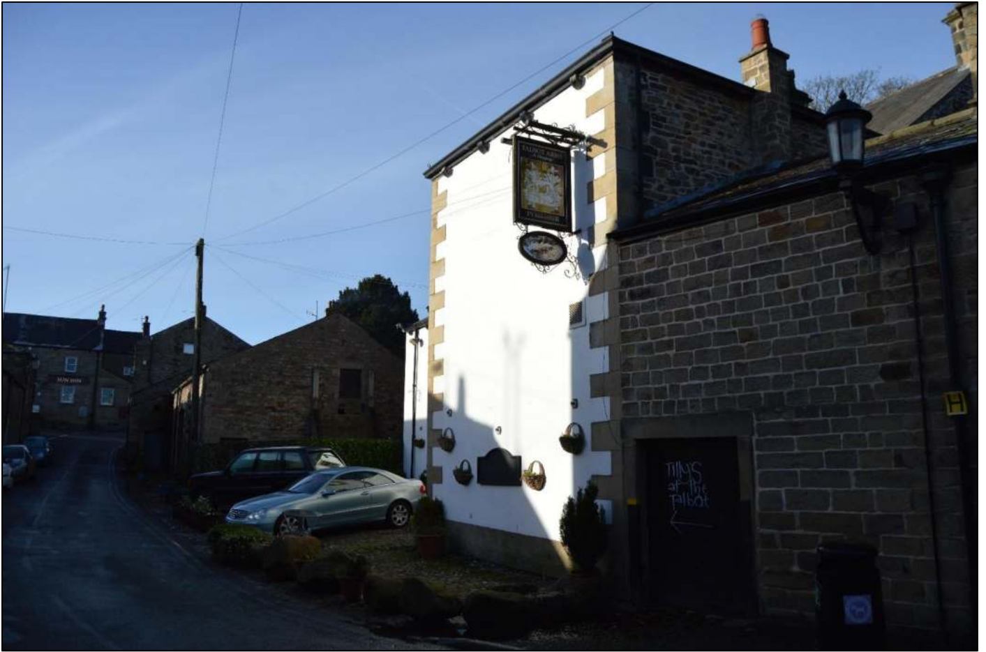
PL05: View of the Talbot Hotel and adjacent barn from the north east end of Talbot Road.
