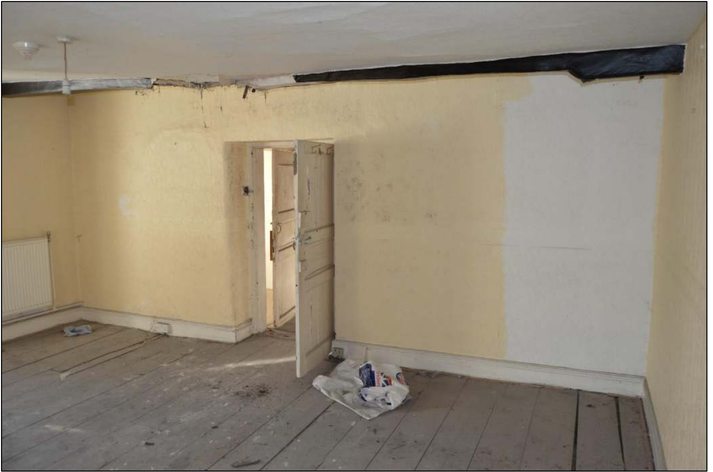
PL53: View south west within the first-floor east unit.
