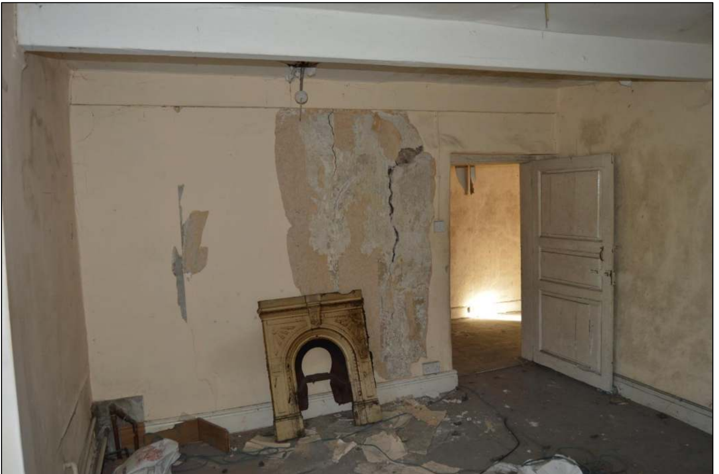
PL58: View north east within the first-floor west unit.
