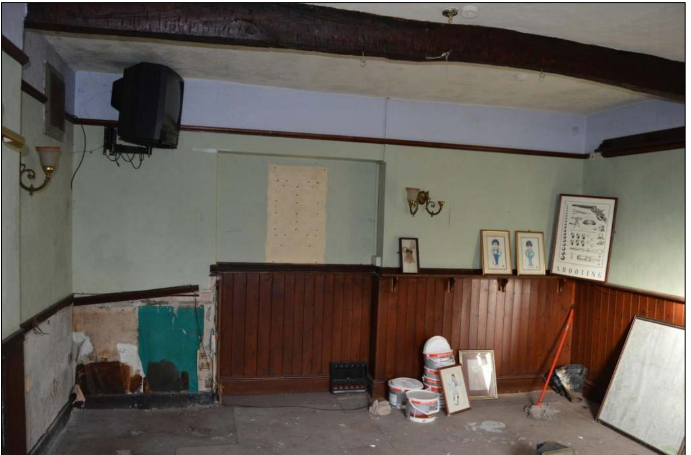
PL16: View north east within the ground floor south unit.
