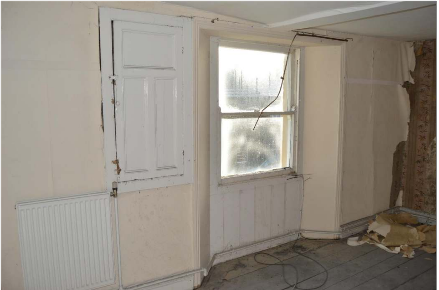
PL51: View south east within the first-floor south unit.
