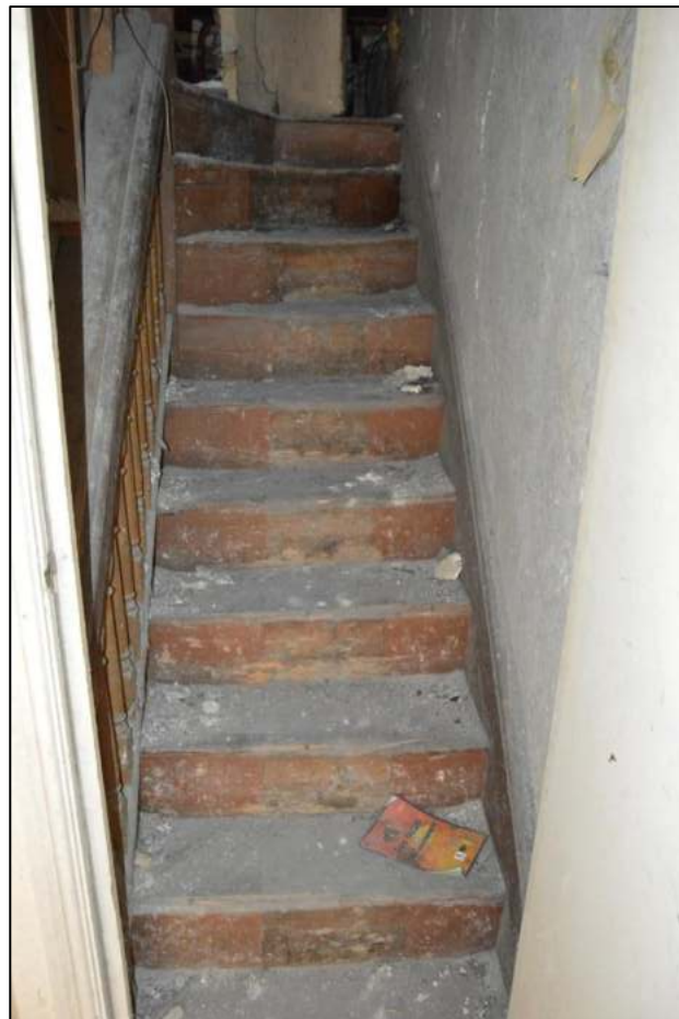
PL62: View of attic staircase.
