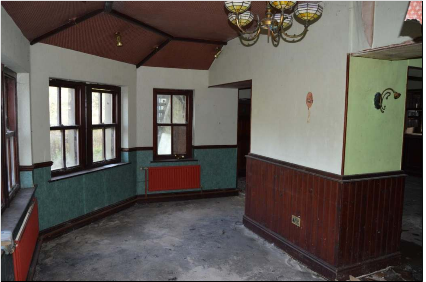
PL31: View north east within the rear extension.
