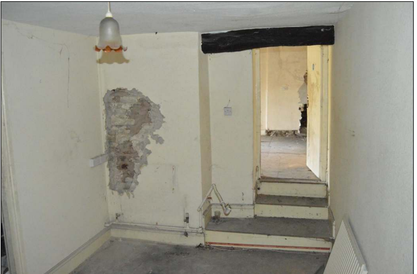
PL46: View north east within the first-floor north unit
