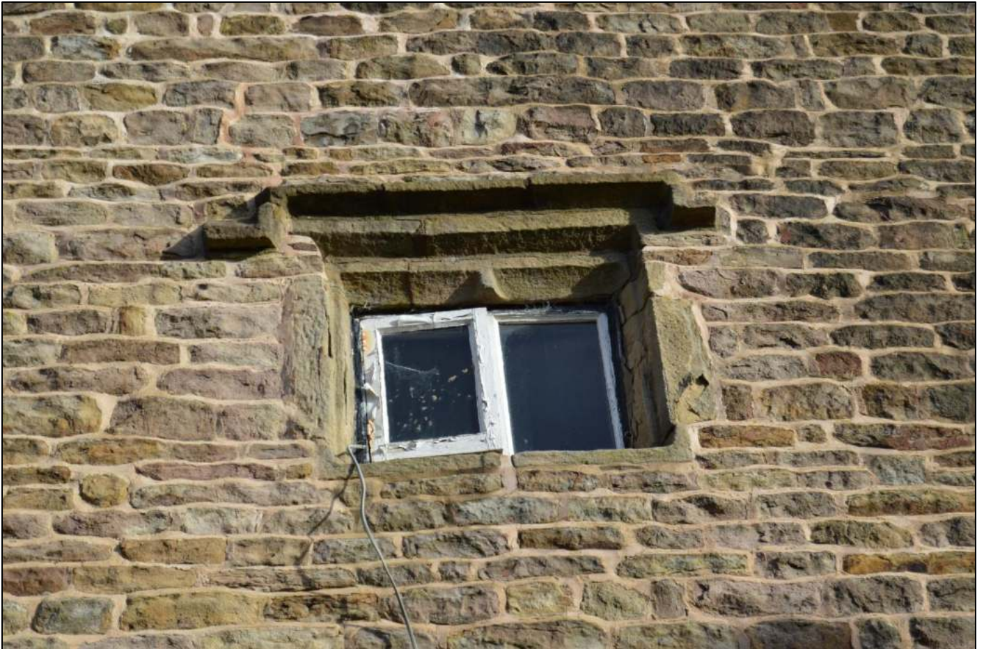
PL09: View of the re-used 17 th century mullioned window (mullion missing), with hood mould present to the south west elevation.
