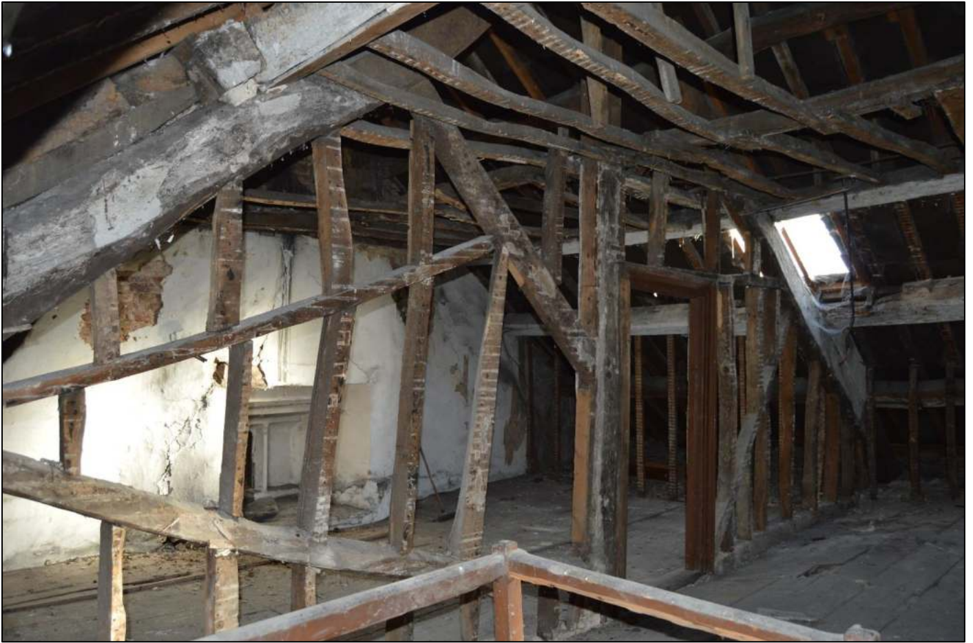
PL65: View of truss and partition timbers from the attic landing.
