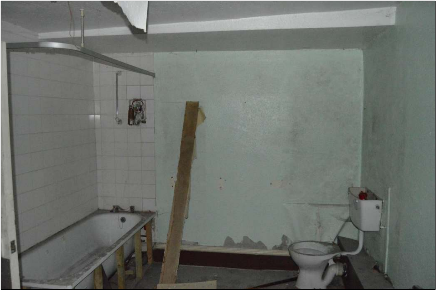
PL43: View south west within the first-floor north unit.
