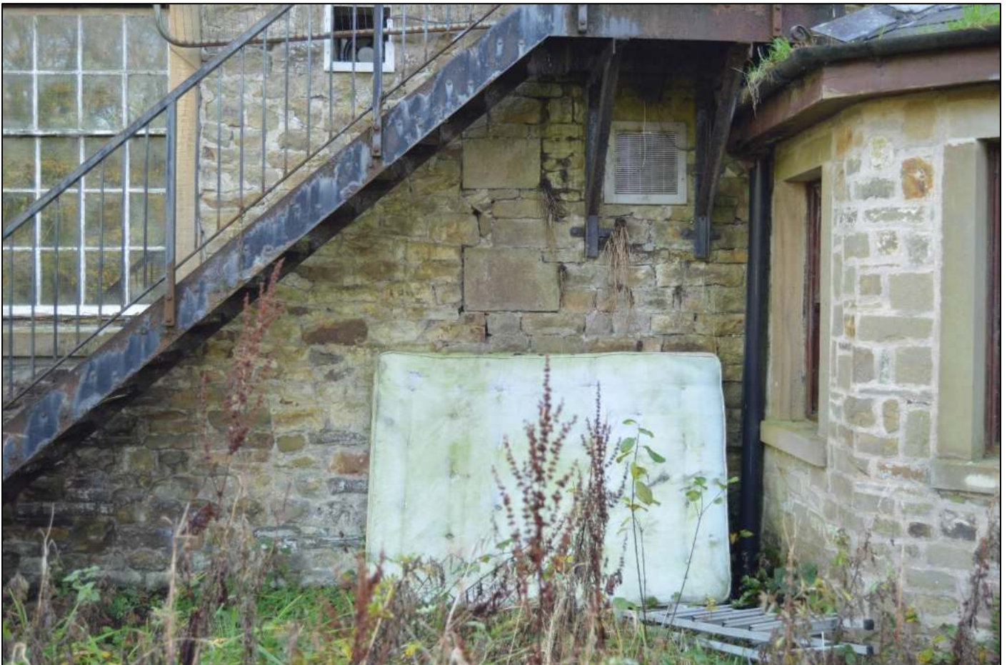
PL14: View of unused quoins denoting the extents of the Talbot Hotel prior to the construction of the coach house.
