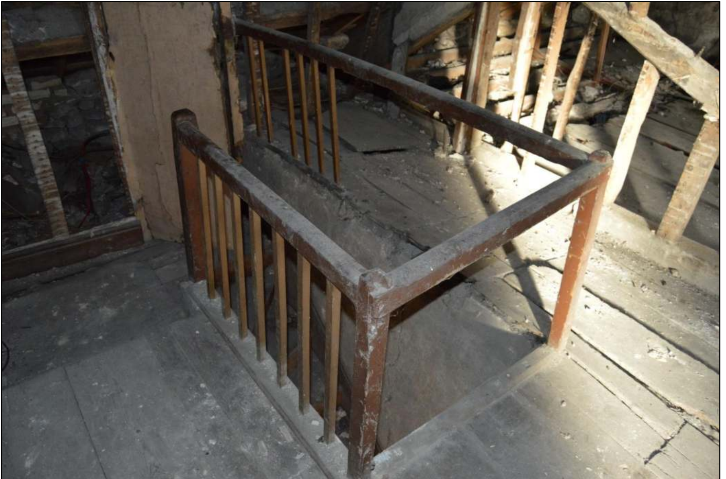
PL63: View of plain and square balustrade and balusters to the attic staircase.
