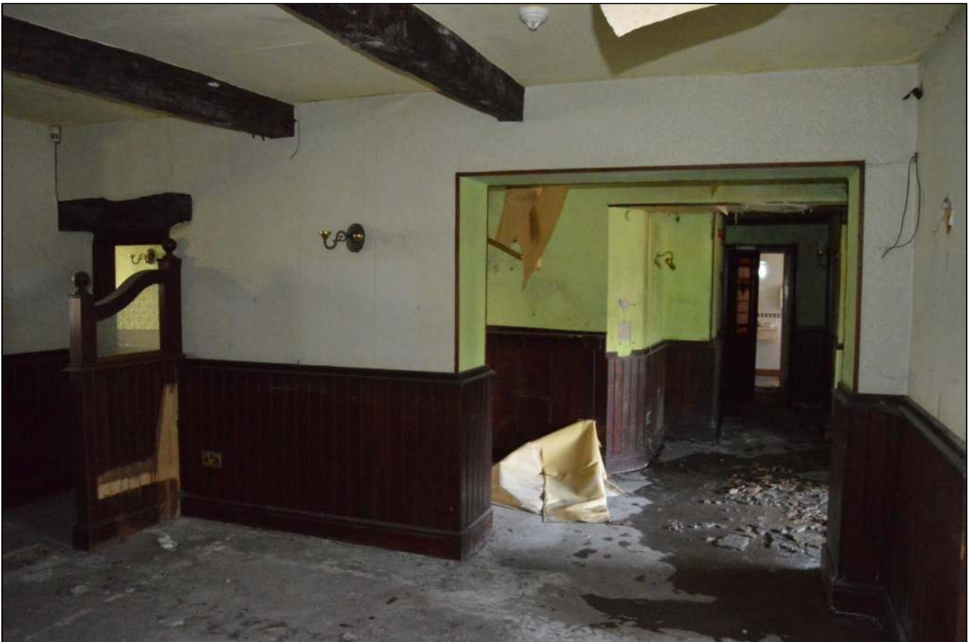
PL30: View south west within the ground floor north unit.
