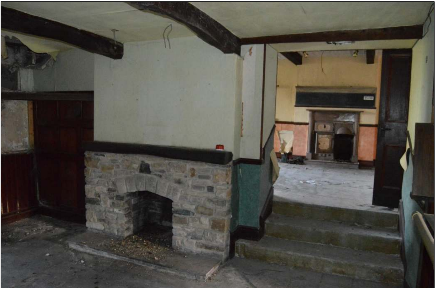
PL28: View north east within the ground floor north unit.
