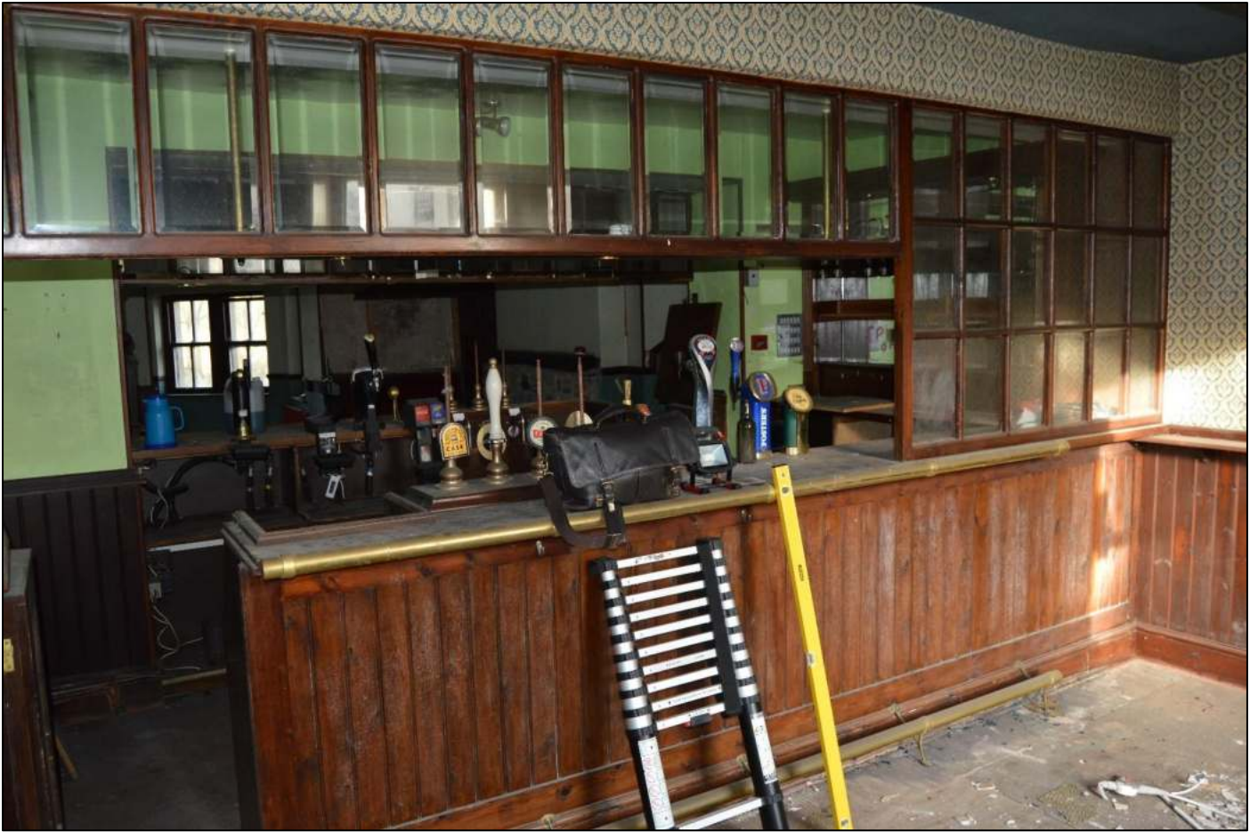
PL23: View north west within the ground floor east unit.
