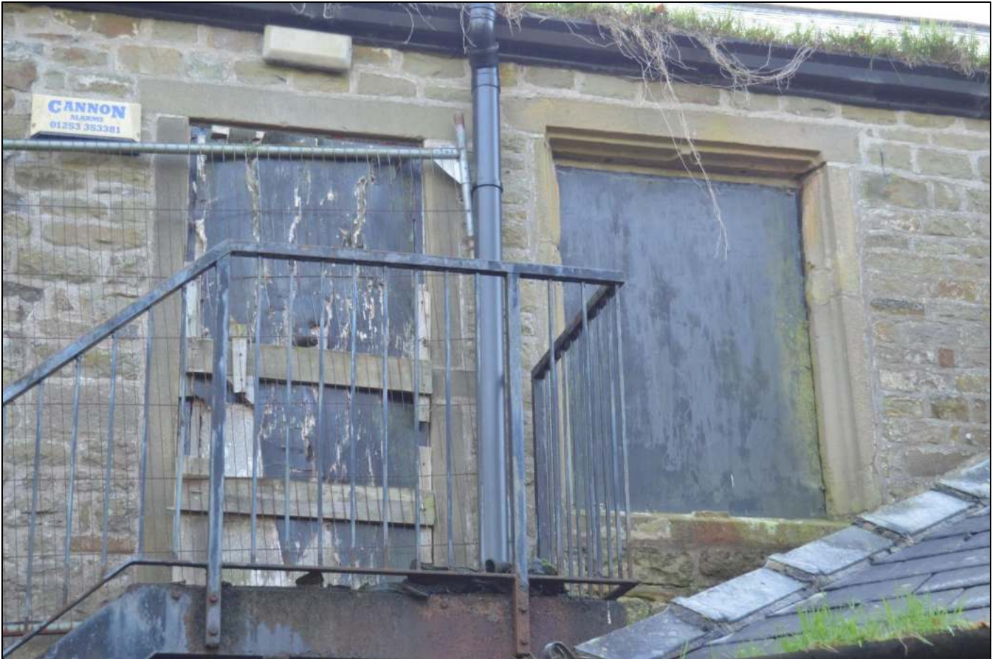
PL13: View of the inserted first floor doorway and the re-used 17 th century former cross window (mullion and transom missing).
