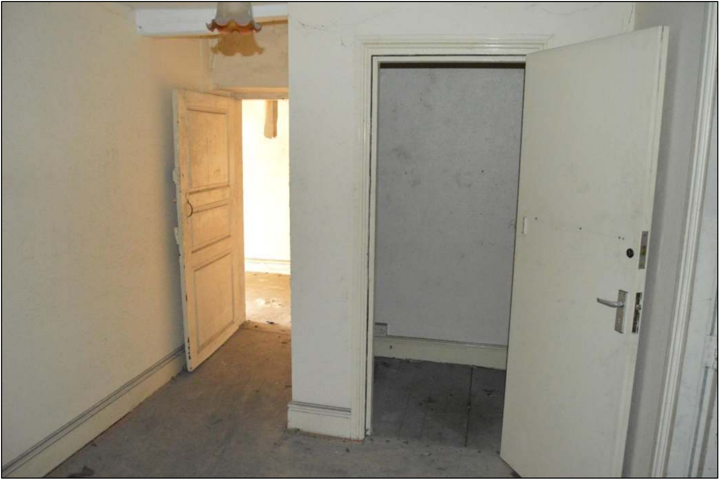
PL45: View south west within the first-floor north unit.
