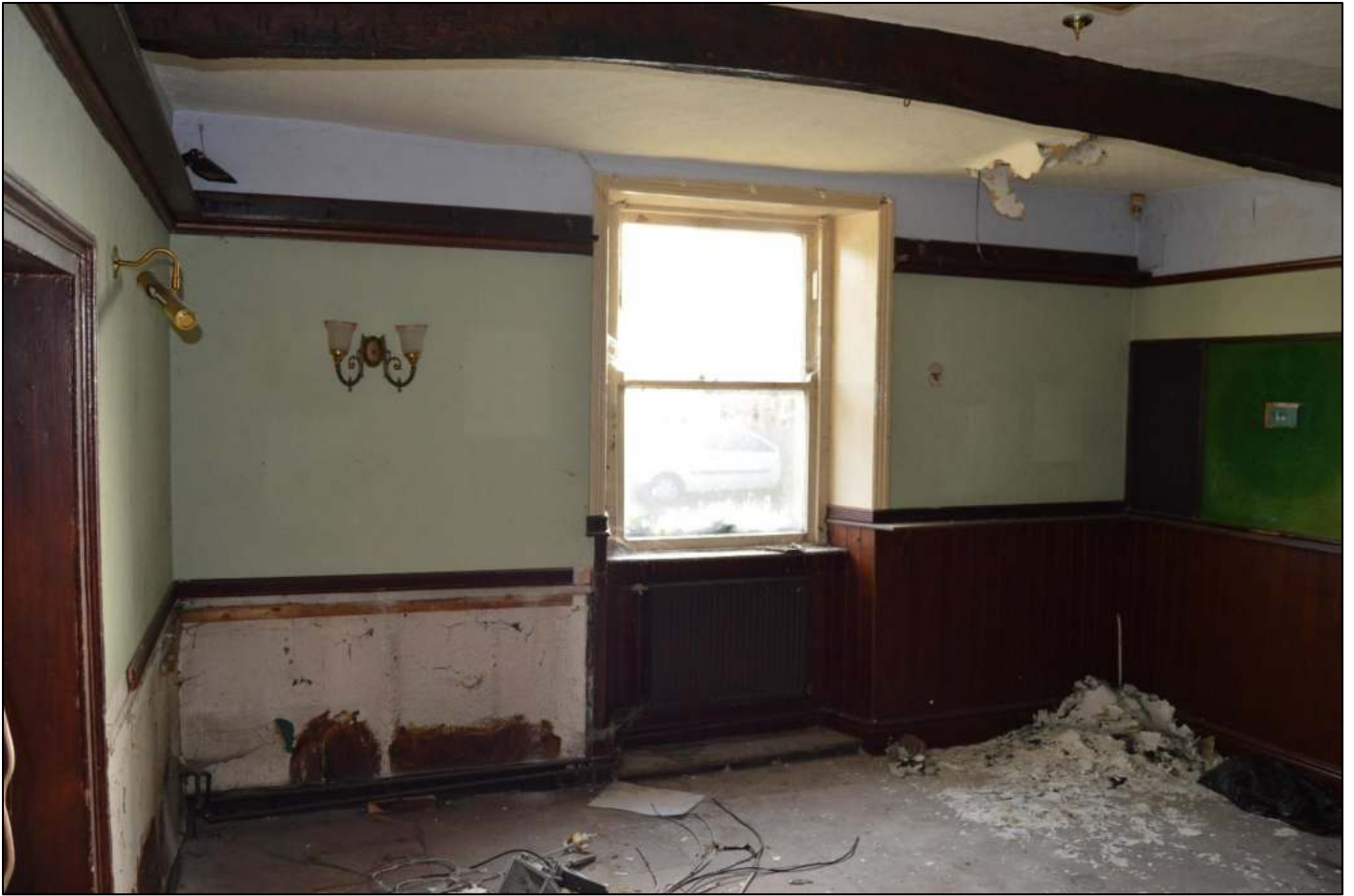
PLI 7: View south west within the ground floor south unit.
