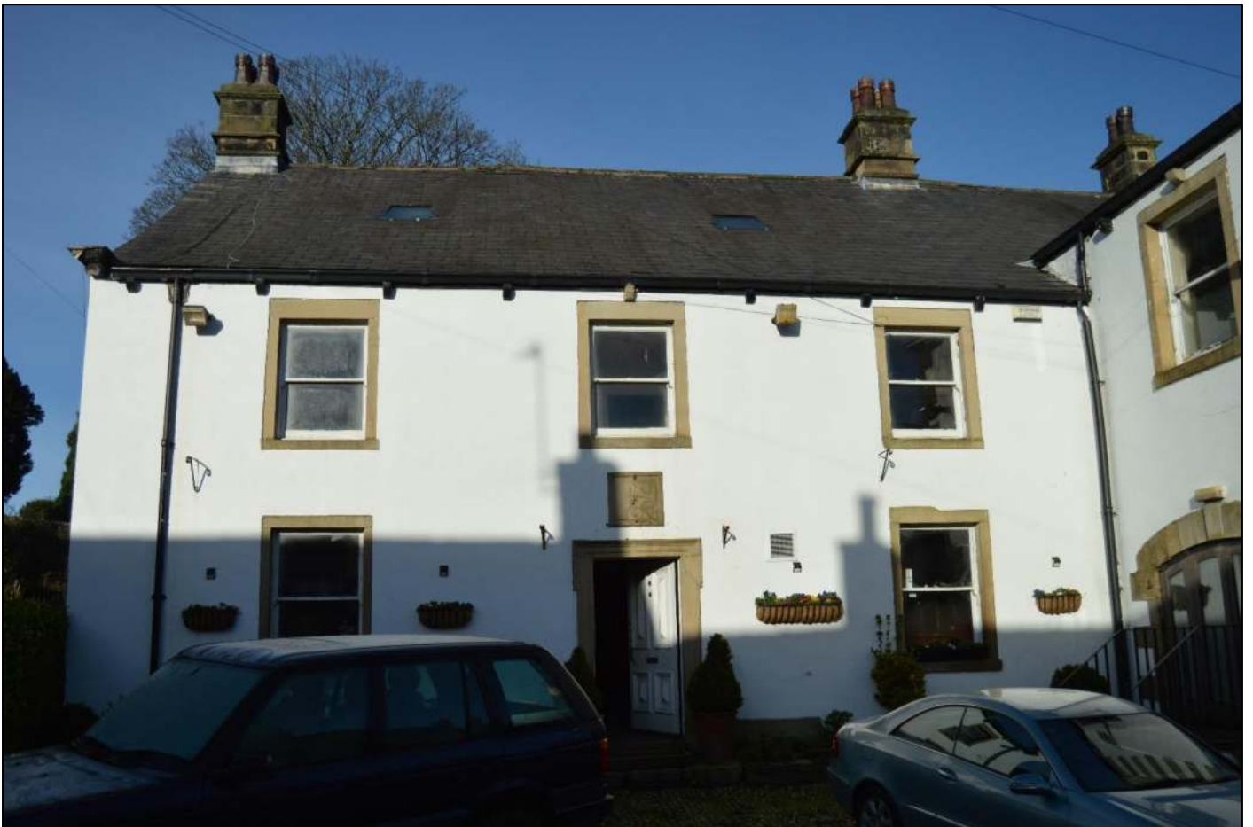
PL02: View of the front south east facing elevation of the Talbot Hotel.
