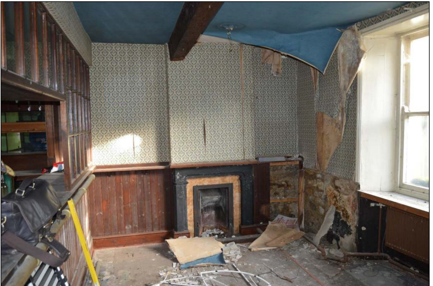
PL20: View north within the ground floor east unit.
