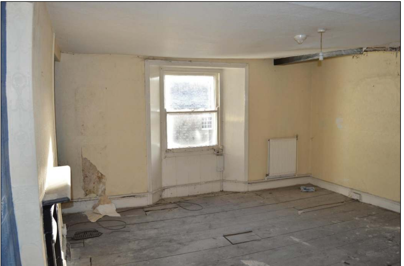
PL54: View south east within the first-floor east unit.
