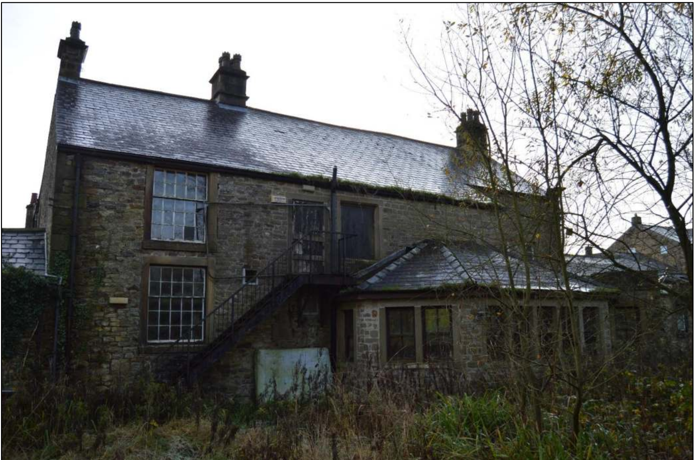
PL12: View of the Talbot Hotel from the North East.
