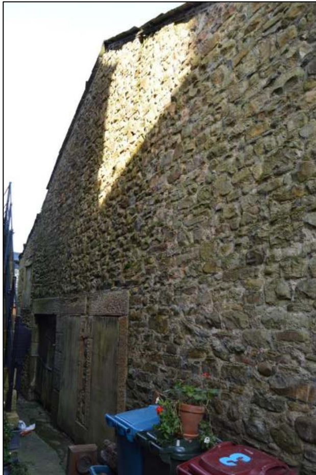
PL77: View of the south west gable from the south.
