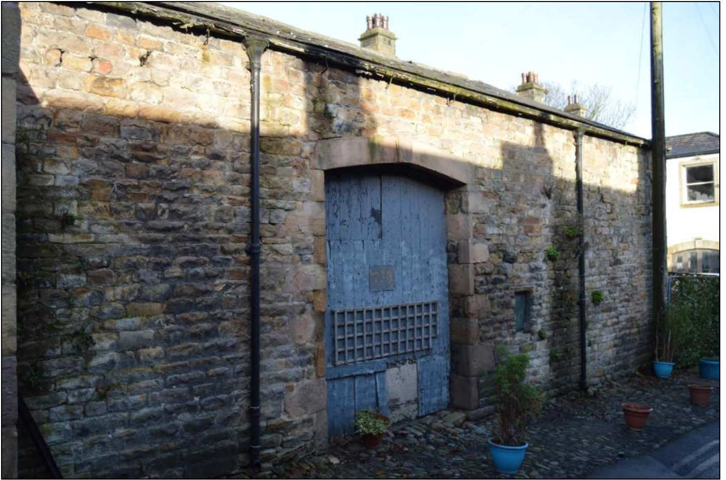
PL73: View of the front south east facing elevation of the barn.
