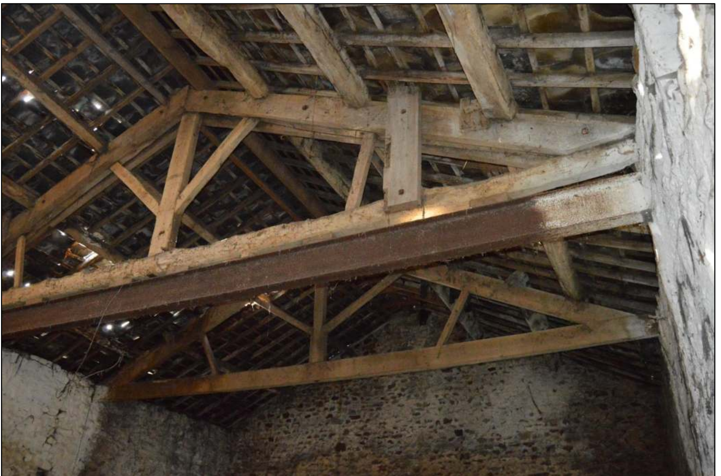
PL84: View of the 2no timber king post roof trusses to the south end of the barn.
