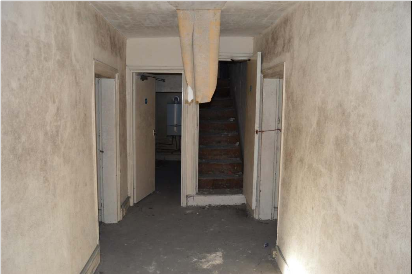
PL47: View north west within the first-floor landing.
