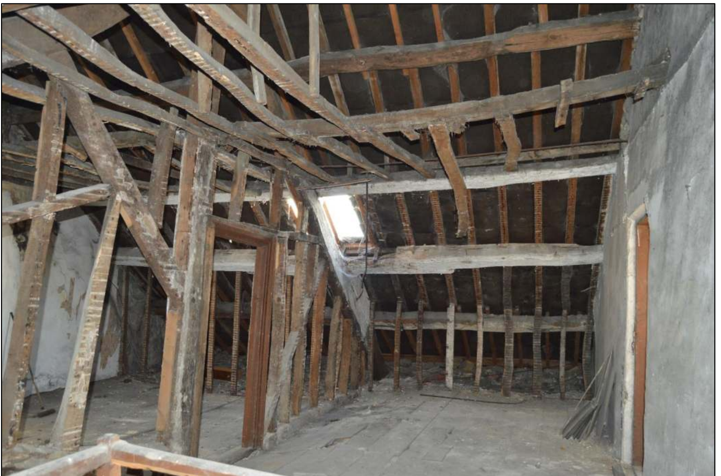
PL64: View south west within the central attic landing.
