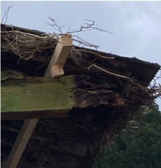
Please see above photographs of the existing beams at close range, as shown there has been large ingress of water over the years it has been derelict, resulting in excessive water damage to the beam ends. This is then worsened by the insect infestation which has resulted in the original timber being able to be pulled apart by hand.
