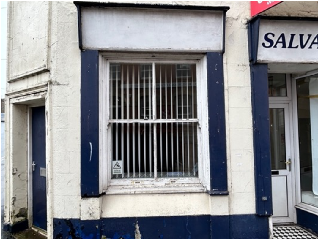
PL03: Ground floor sash window, likely re-glazed late C20.
