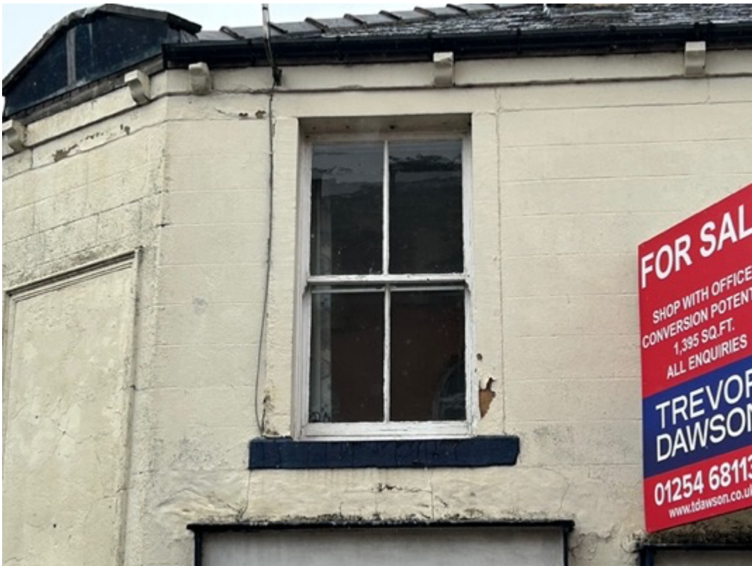
PL04: First floor sash window. Original cylinder/ drawn glazing in-situ.
