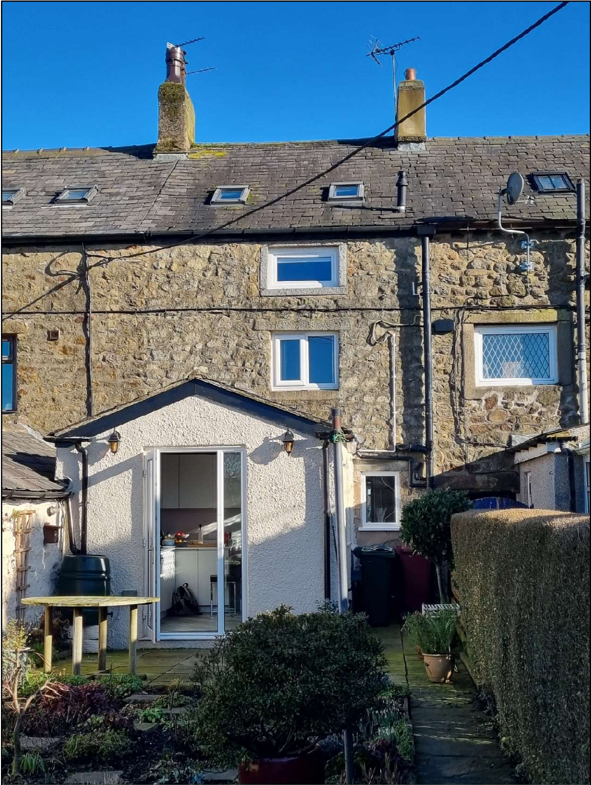
Figure 11 A more detailed photograph of the rear elevation of the asset. The proposed alterations apply to the windows embedded in the original fabric of the build, and does not include the frames or glazing in the modern kitchen extension (source - Jamie Skuse)
