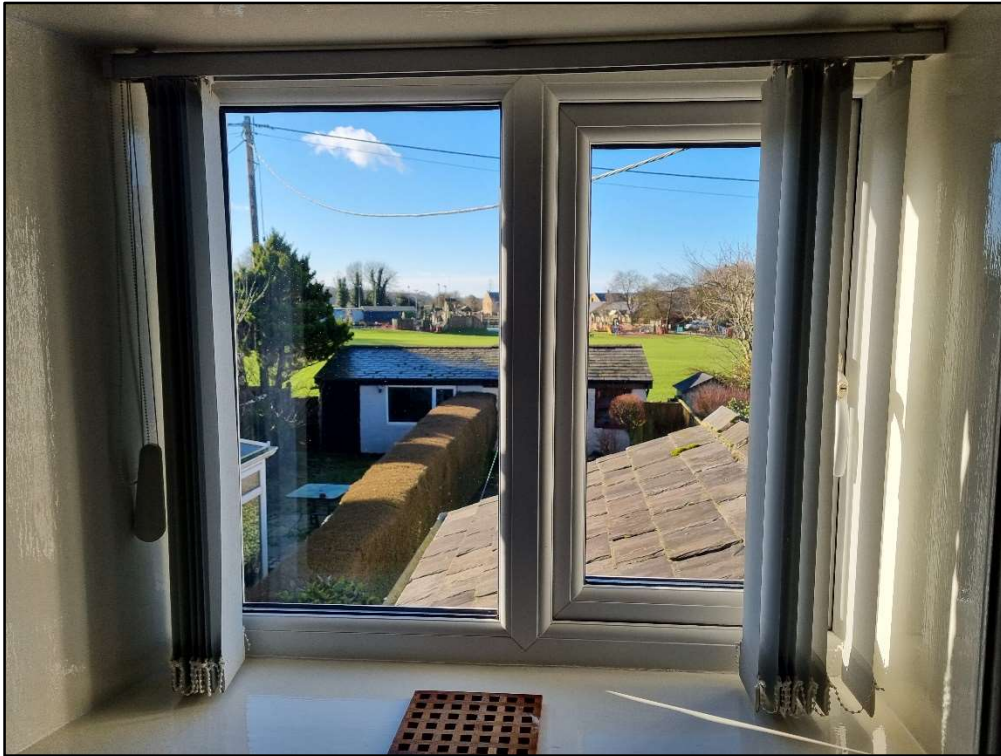
Figure 15 The internal aspect of the first-floor window on the rear elevation (source - Jamie Skuse)
