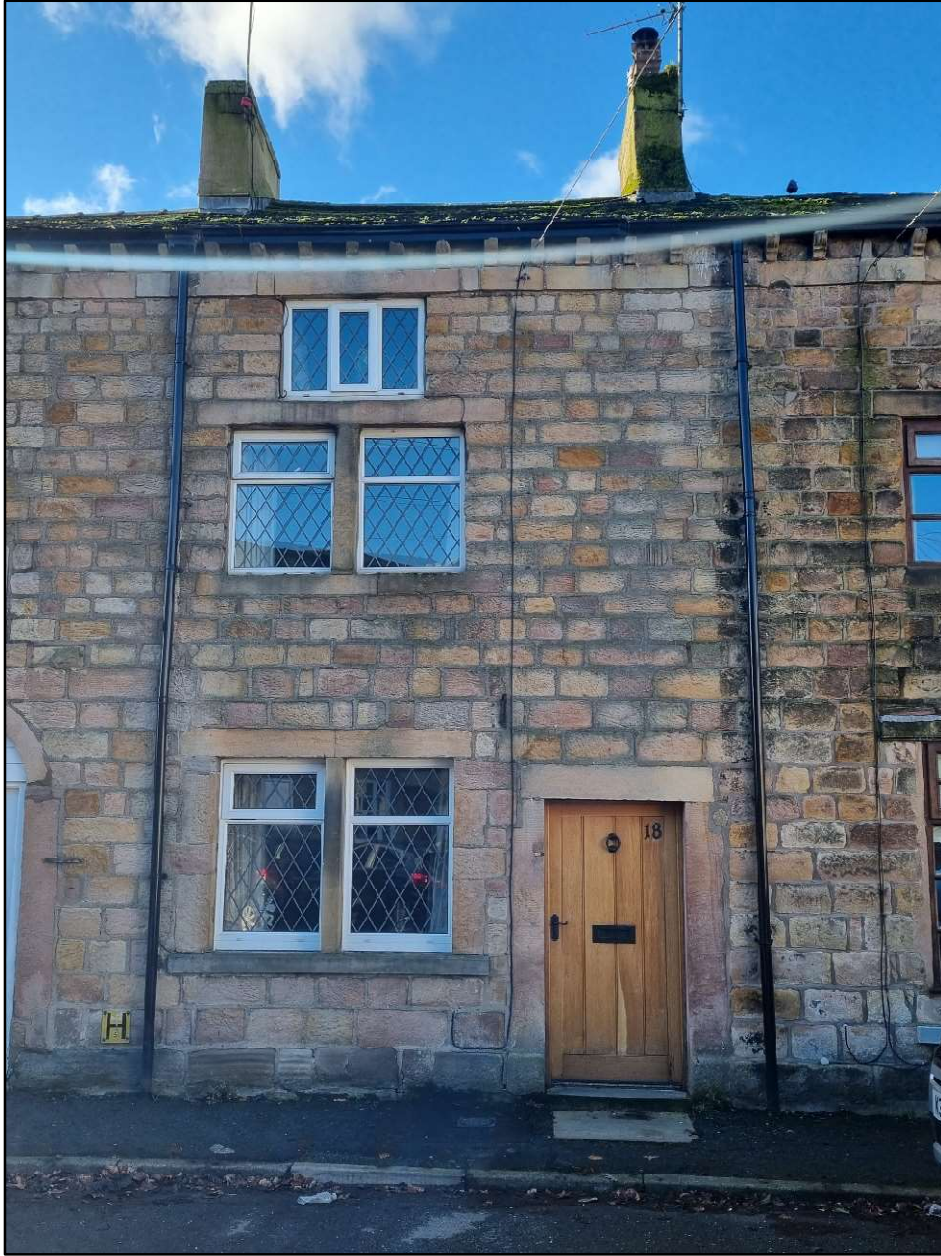
Figure 1 The front elevation of No 18 Church Street. The windows are the subject of the proposed alterations to the heritage asset (source - Jamie Skuse)
