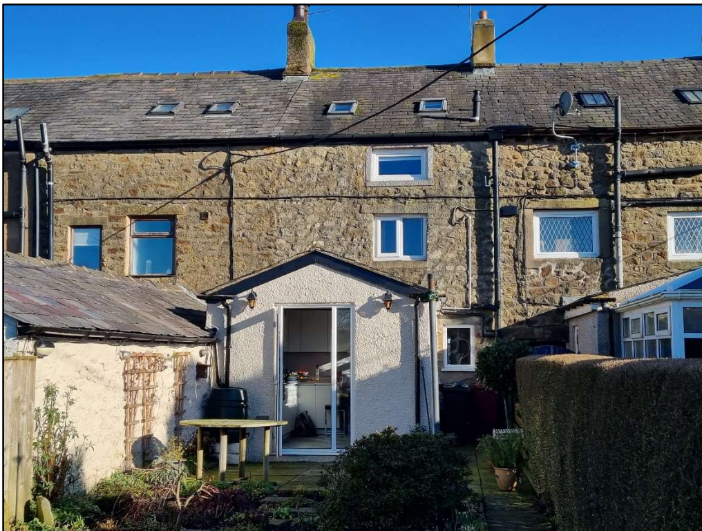
Figure 4 The rear elevation of the asset. The three windows on the original rear facing wall are subject to the proposed alterations (source - Jamie Skuse)
