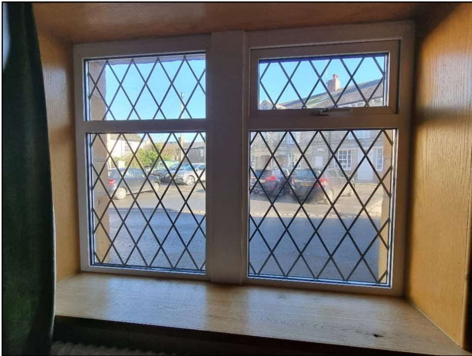
Figure 8 The internal aspect of the ground floor window on the front elevation looking outwards towards Church Street (source – Jamie Skuse)
