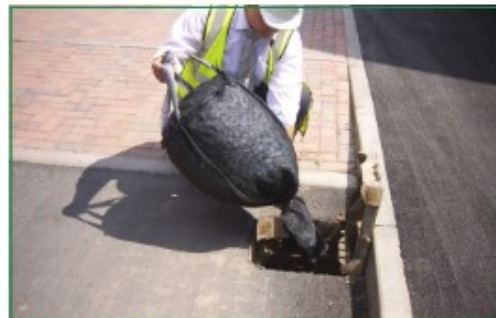
2. Hold handles at top of the Gully Guard, work beads to top and insert base into water filled gully pot.
