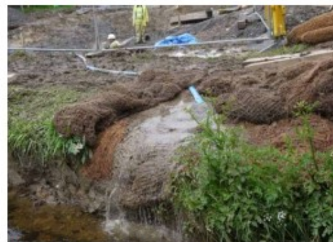
Deployed to treat muddy excavation water
