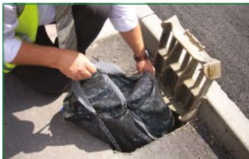
3. Lower the Gully Guard into the pot. The beads will fall freely into the void within the pot.
