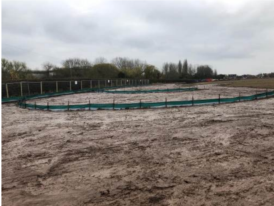
Installation of silt fencing to control run-off from an unsurfaced area
