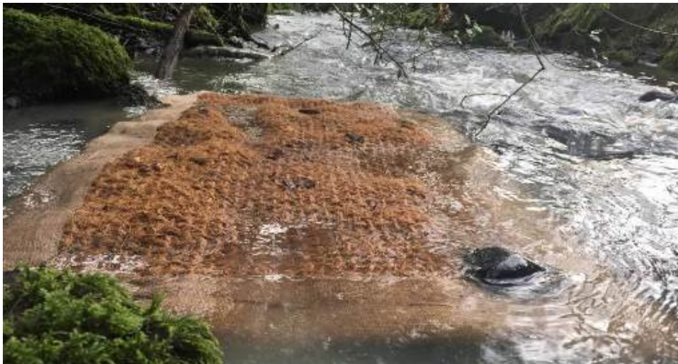
Placement of silt matting to capture settled silt downgradient within a surface watercourse (image courtesy of Frog Environmental)
