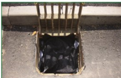
5. Close gully grid.
