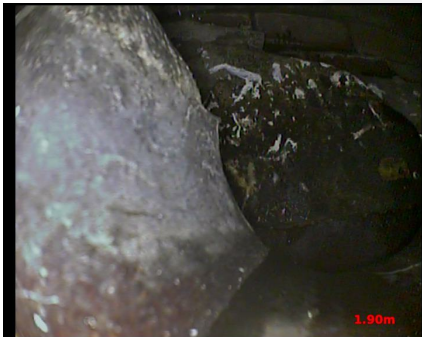
Observation [5]: MH4 INTERNAL
