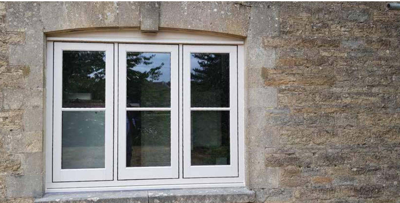
Timberlook windows have been specifically designed with a slimmer sash profile to accurately mimic heritage timber frame sections. It features a traditional chamfer on the outside, with a fully sculptured ovolو detail internally.
