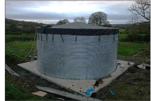
Image of Existing Water Tank
