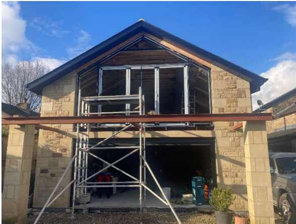
Photograph 5: south elevation of subject development as constructed. The piers and steel work to the front, designed to support a terrace, are proposed to be removed
