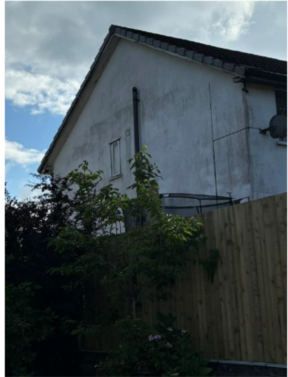
Photograph 3: Overview of the northwest elevation.
