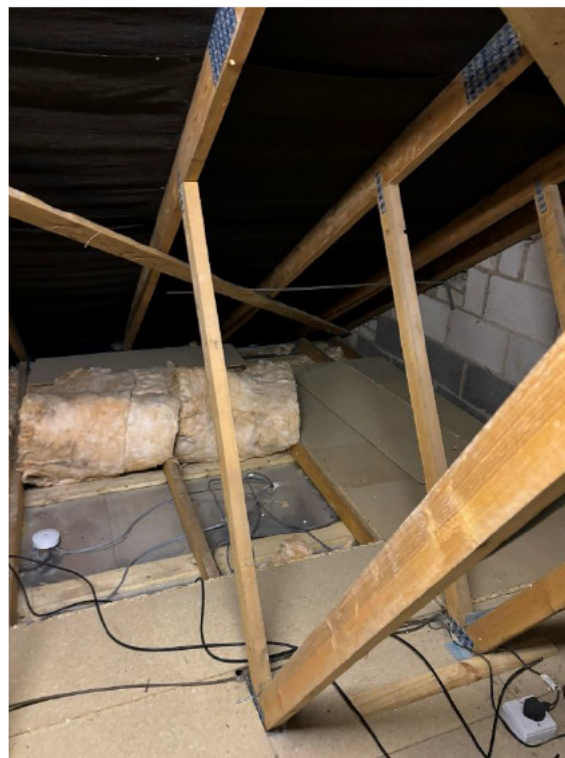
Photograph 8: Timber frames, rafters and roof felt. No evidence of bats identified.
