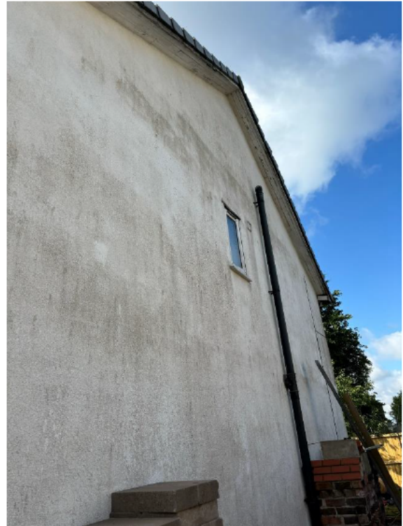
Photograph 4: Under view of northwest elevations wooden soffit, in good condition.
