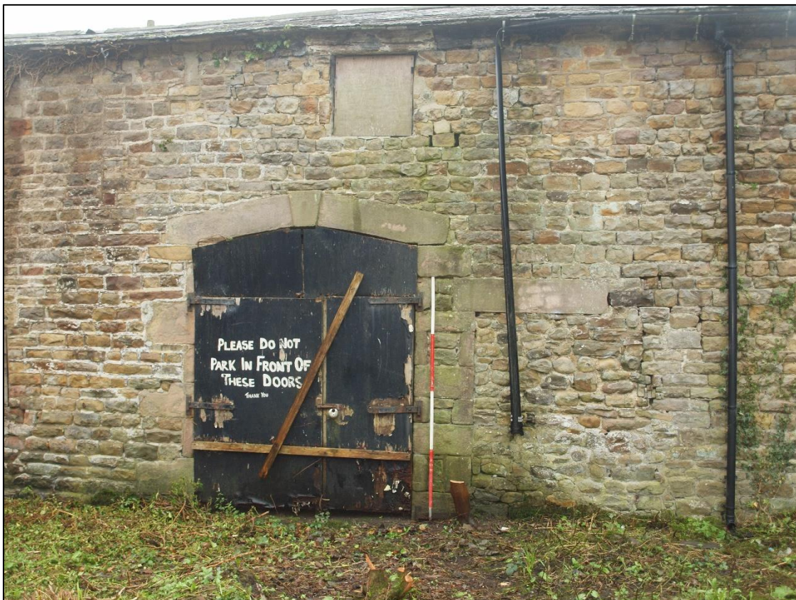
Plate 10: Barn door with cill to be raised
