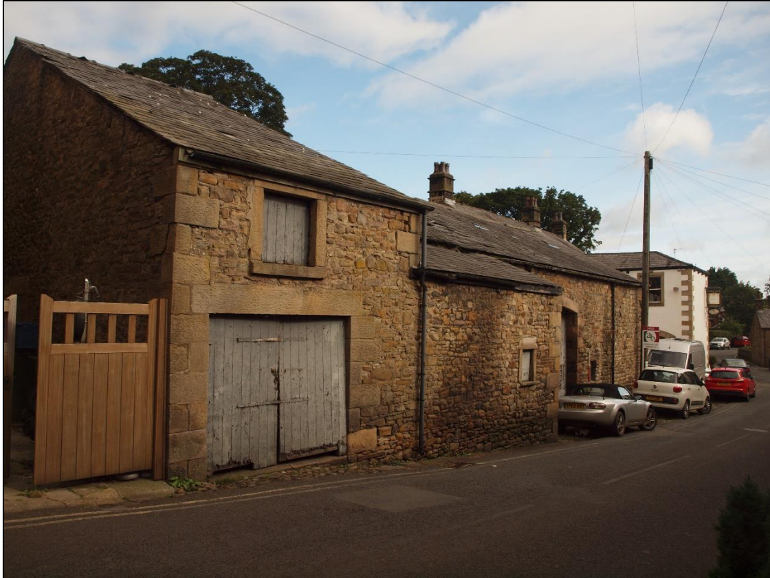
Plate 2: General shot of barn From Talbot Street showing cart door to have cill raised
