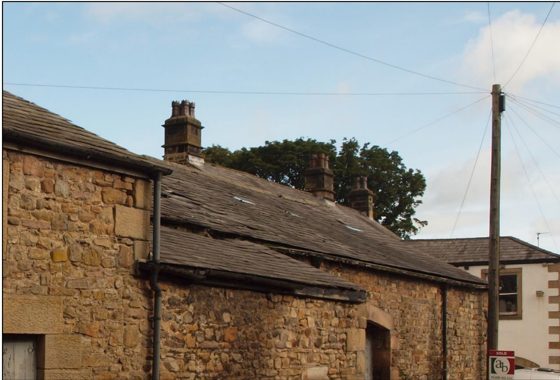
Plate 3: Detail of roof showing skylights and ridge
