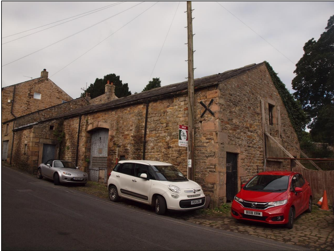
Plate 1: General shot of barn from Talbot Street
