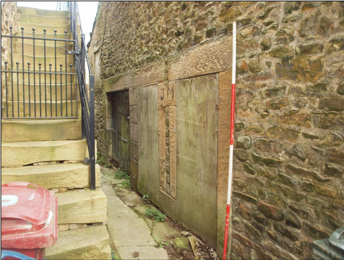
Plate 7: West gable showing doorways with cills to be raised
