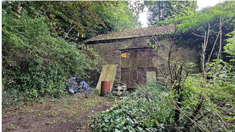
Photograph 7: Substation in the eastern section of the site – not to be affected by the proposals.
