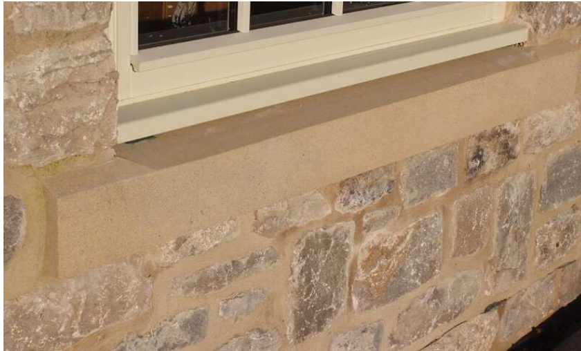
Typical detail of a natural stone cill
