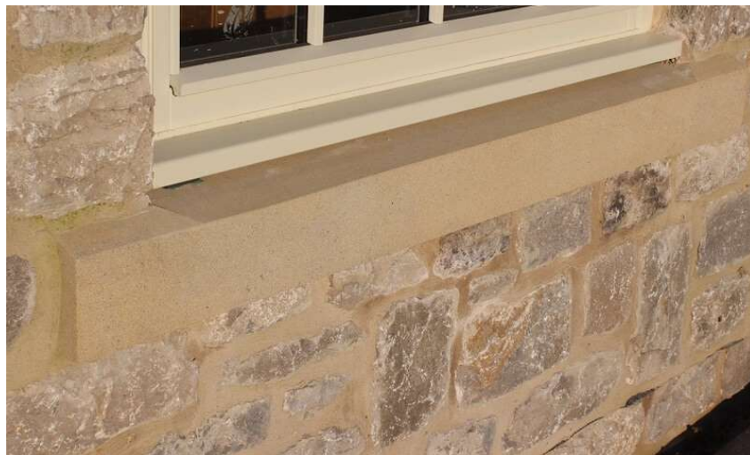
Typical detail of a natural stone cill
