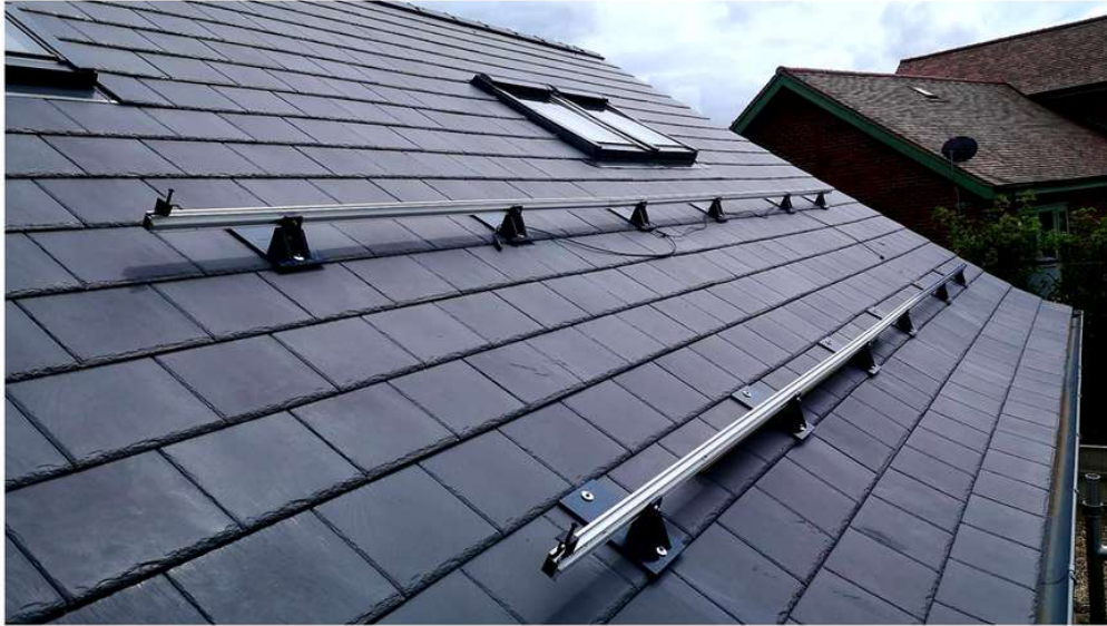
Retro fit framing for the solar PV array
