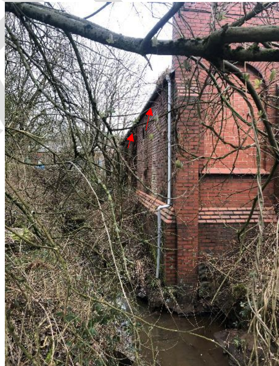
Photograph 12: Watercourse and riparian corridor immediately adjacent to west of Building 3.
