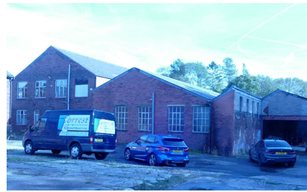
External View - Service Yard
