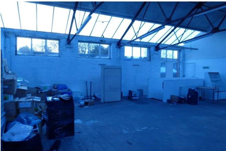
Internal view of upper floor
