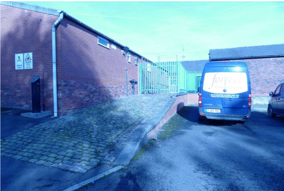
The "protected" access route within the site.
