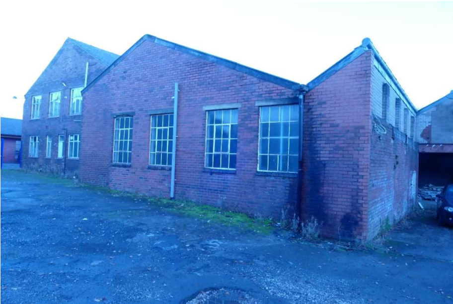
North facing elevation of the former Bakery building.
