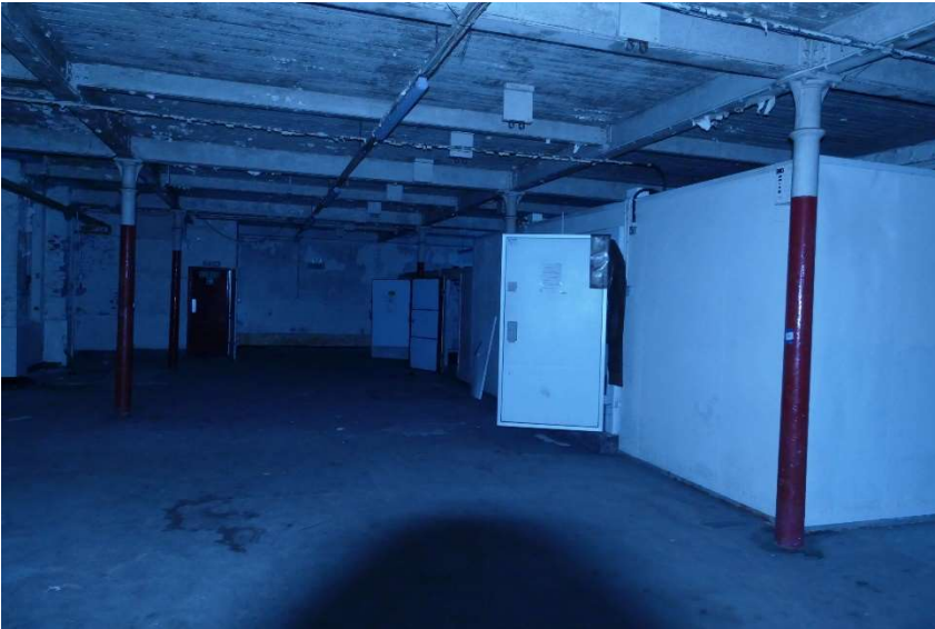
Typical interior view of the former Bakery
