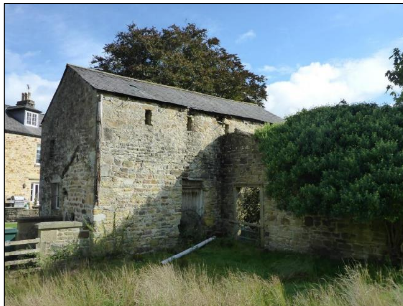
Plate 6. Photograph of the Rear (south) Elevation of the (Paul Waite Associates, 2023)
