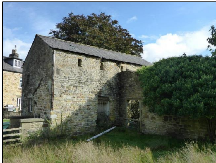
Plate 5. Photograph of the Rear (south) Elevation of the (Paul Waite Associates, 2023)
