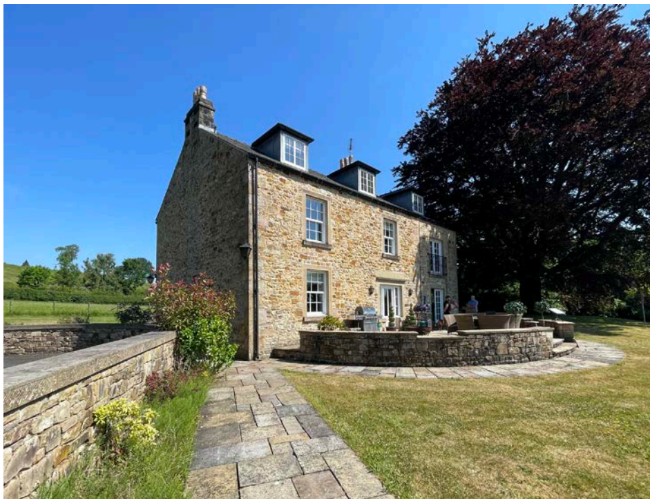
Rear elevation and patio area.
