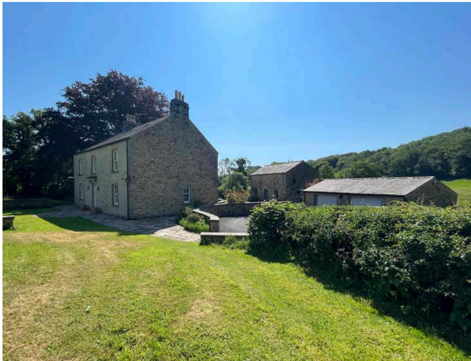
View along original driveway.
