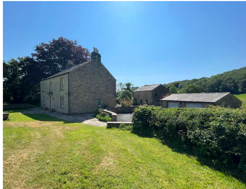
View along original driveway.
