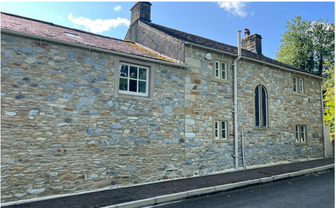
Figure 6) Road facing elevation showing vertical joint between house and barn parts and arch topped stair window to the centre of the house
