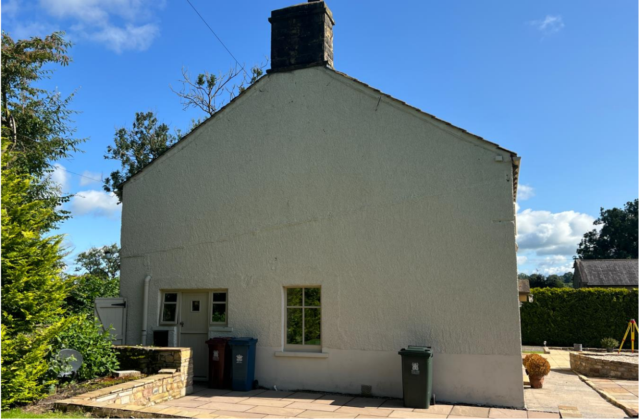
Figure 5) Western gable – both openings appear inserted (non-original)
