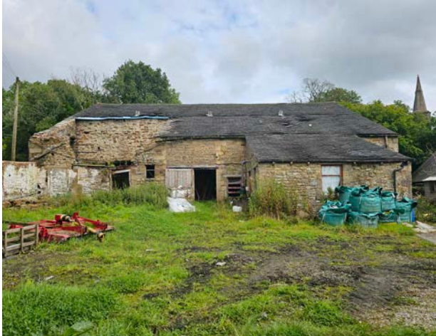
Figure 8 View of the west facing elevation of the main barn.
