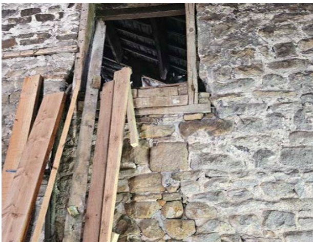
Figure 18 View of an opening in the central passageway.
