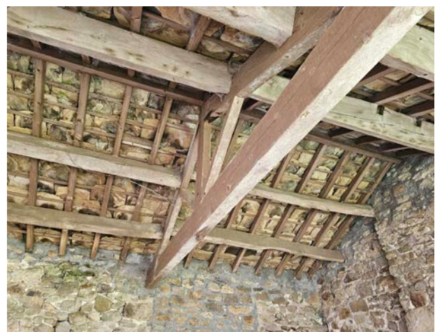
Figure 7 Interior of the open fronted structure.
