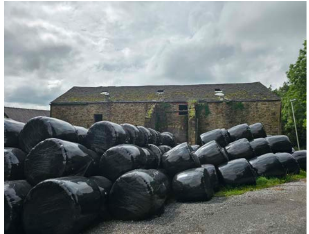
Figure 11 East facing elevation of the main barn.
