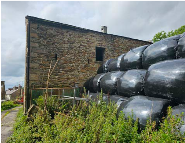
Figure 10 East facing elevation of the main barn.
