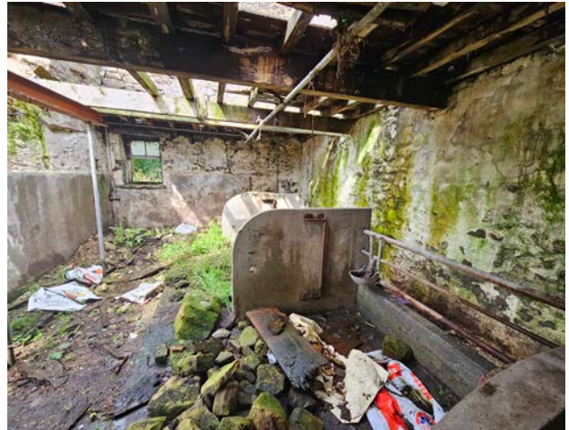
Figure 23 View of an additional room used for housing livestock.
