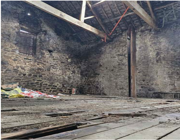
Figure 28 View of the first floor.
