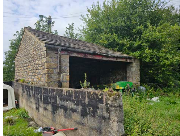
Figure 3 East facing elevation of the open fronted structure.
