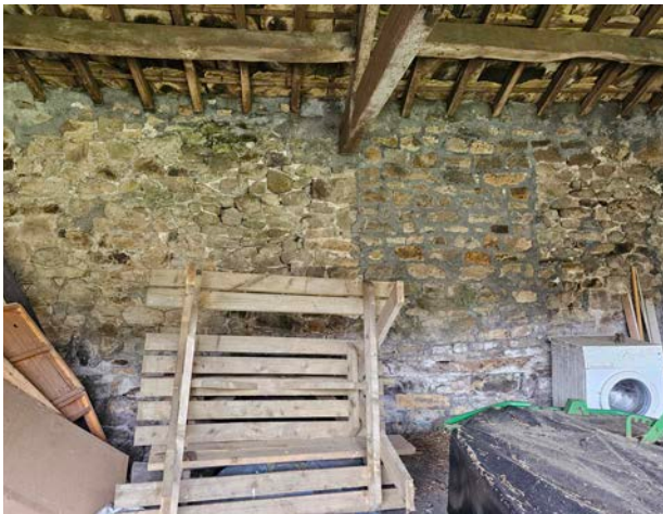
Figure 4 Interior of the open fronted structure.
