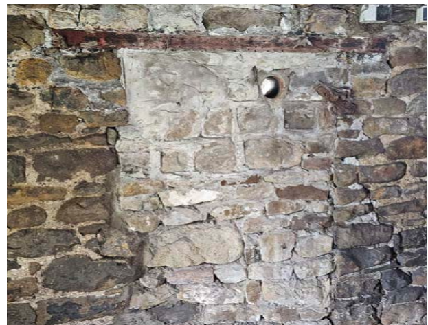
Figure 19 View of a blocked openings in the central passageway.
