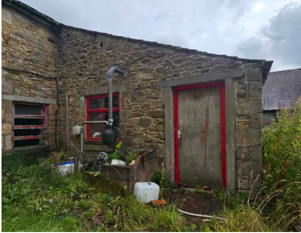
Figure 29 External view of a probable storage room.
