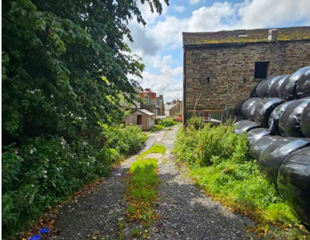
Figure 35 Views of the east facing elevation of the main barn.
