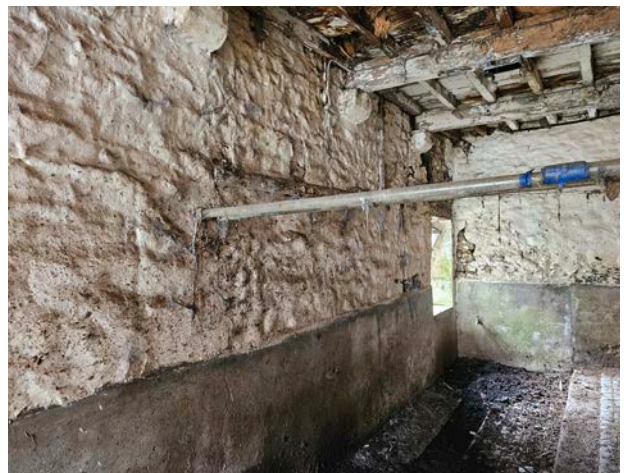
Figure 25 View of an additional room used for housing livestock.
