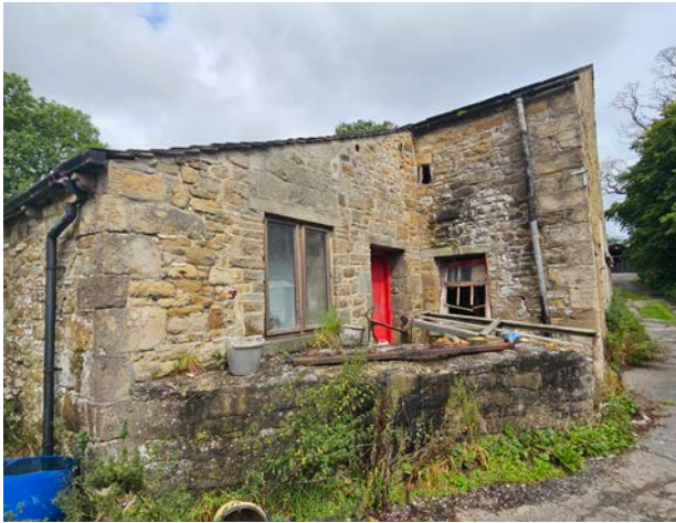
Figure 31 External view of a probable storage room.
