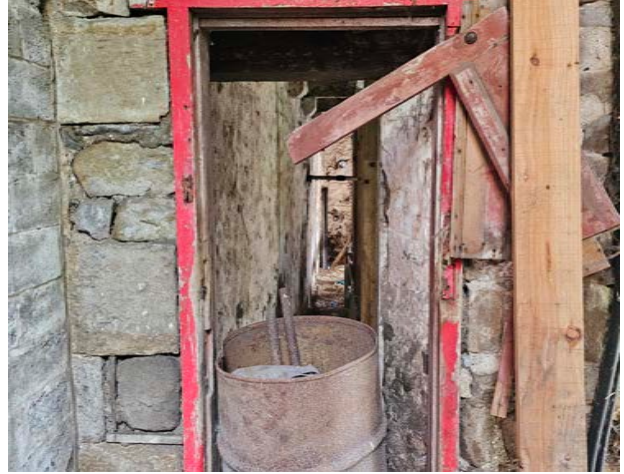
Figure 21 View of an opening in the central passageway.
