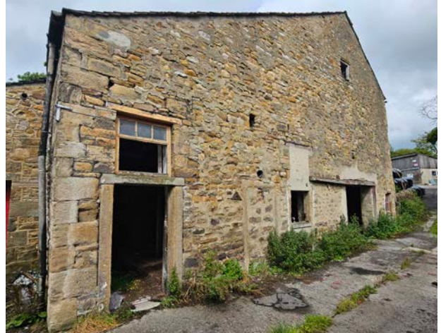
Figure 9 South facing elevation of the main barn.
