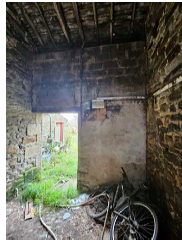
Figure 17 View of the central passageway.
