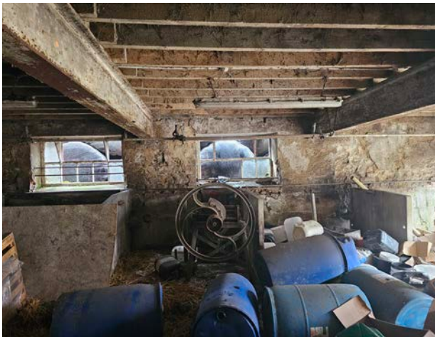
Figure 16 View of the concrete stalling in the main cowhouse.
