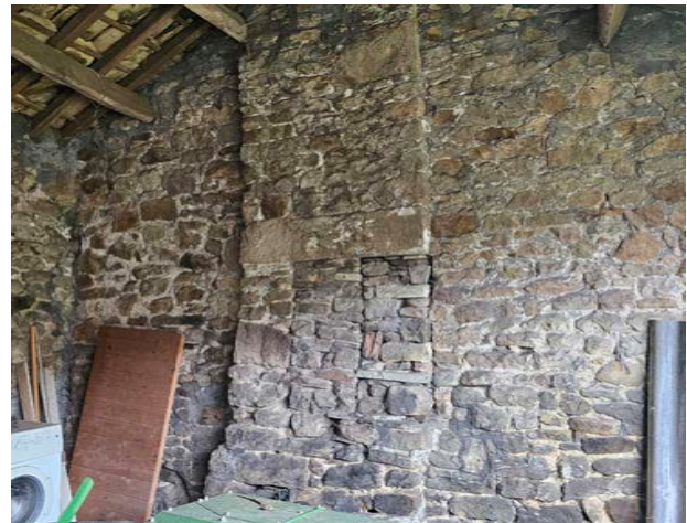
Figure 5 Interior of the open fronted structure.
