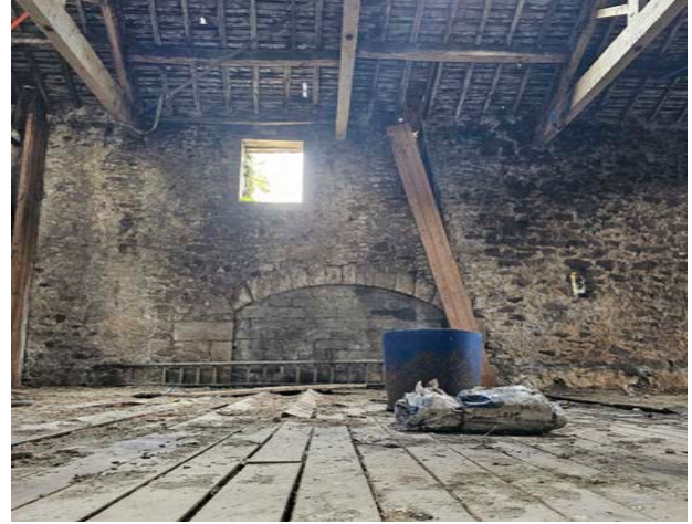
Figure 27 View of the first floor.
