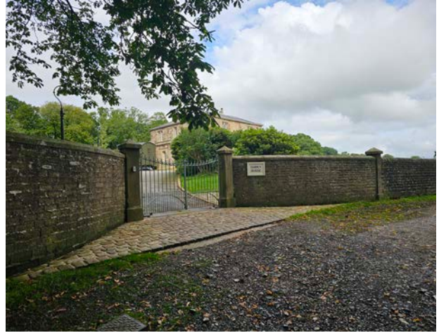
Figure 45 View of Sabden House, Sabden.
