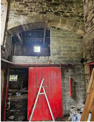
Figure 20 View of the central passageway.
