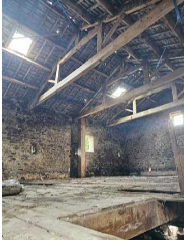
Figure 26 View of the first floor.
