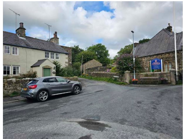
Figure 38 View of Cockshotts Barn from Stubbins Lane.
