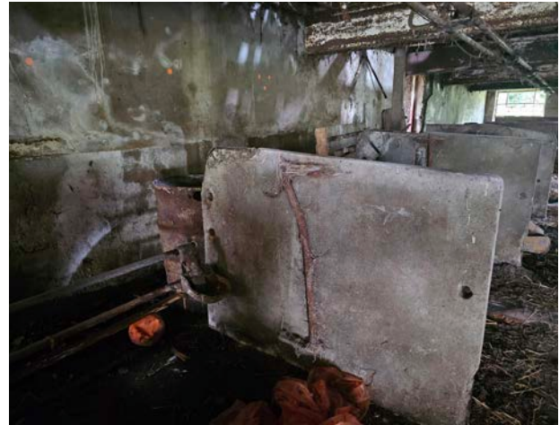
Figure 15 View of the concrete stalling in the main cowhouse.
