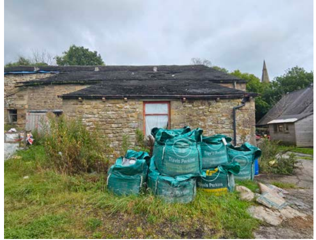
Figure 30 External view of a probable storage room.
