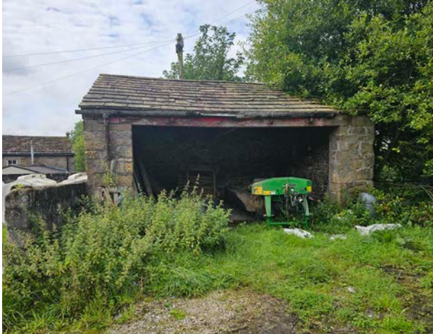
Figure 2 East facing elevation of the open fronted structure.
