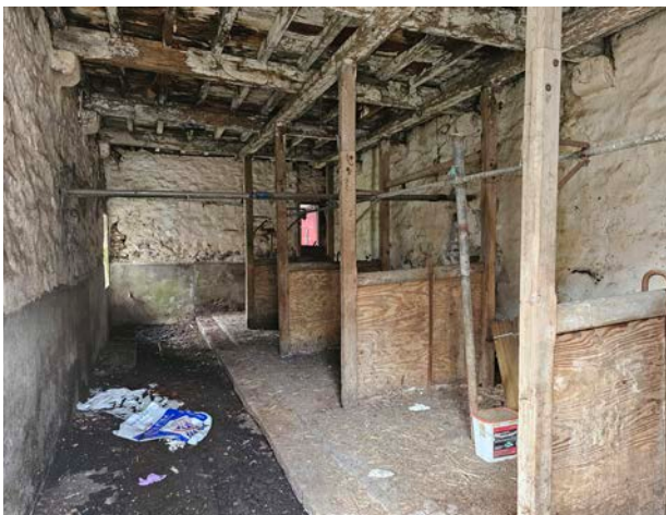
Figure 24 View of an additional room used for housing livestock.
