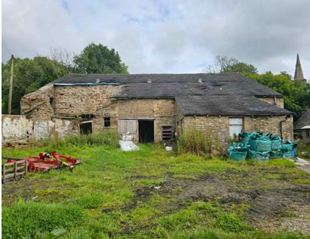
Figure 7 View of the west facing elevation of Cockshotts Barn
