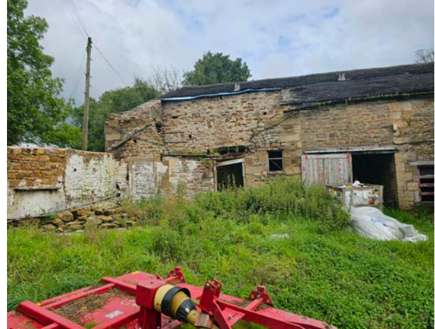
Figure 8 View of the west facing elevation of Cockshotts Barn
