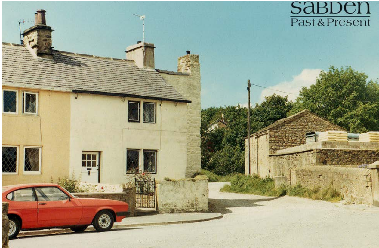
Figure 55 Heyhouses Cottages around the mid 1980s (Source - Heyhouses Cottages 2023)
