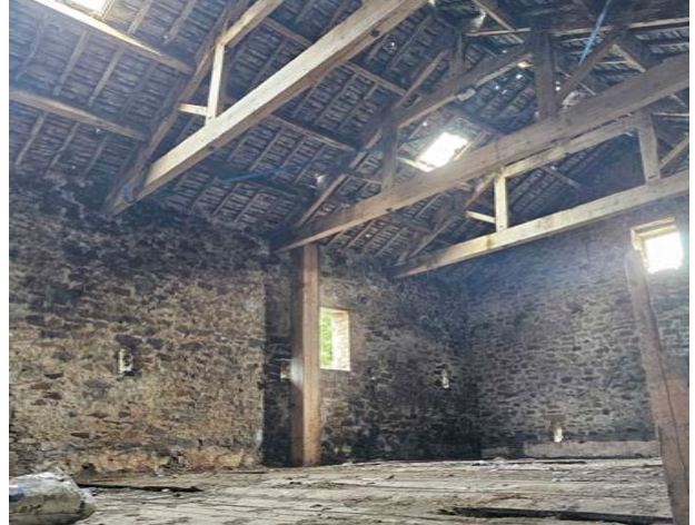
Figure 26 View of the first floor
