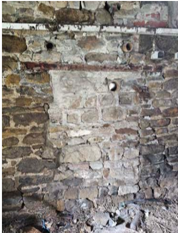
Figure 19 View of a blocked opening in the central passageway
