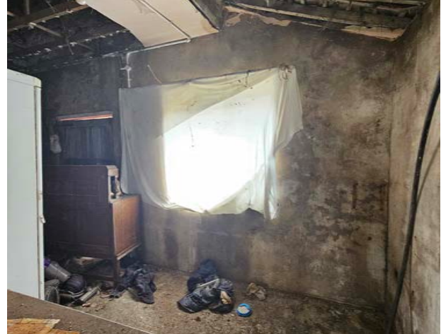
Figure 32 Internal view of a probable storage room
