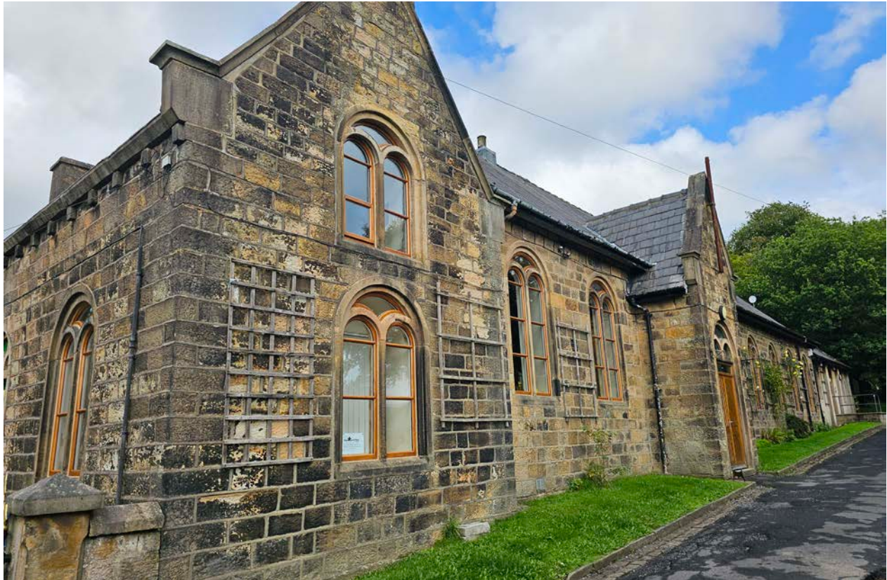
Figure 48 View of Sabden Village Hall
