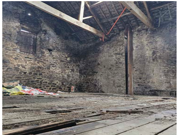
Figure 28 View of the first floor
