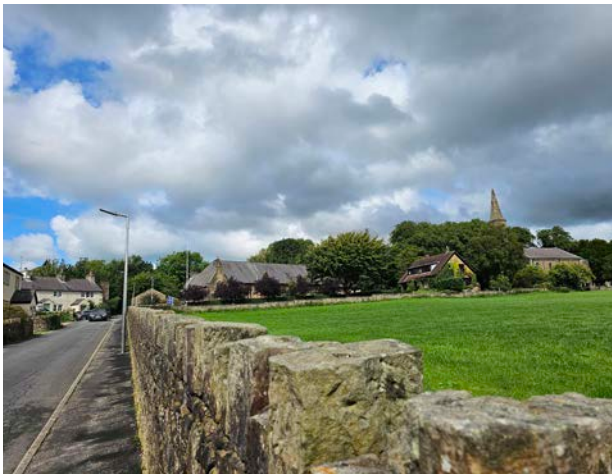
Figure 39 View of Cockshotts Barn from Stubbins Lane
