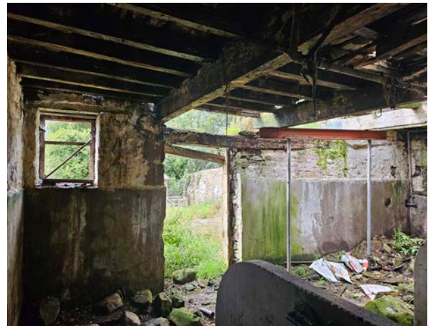
Figure 22 View of an additional room used for housing livestock
