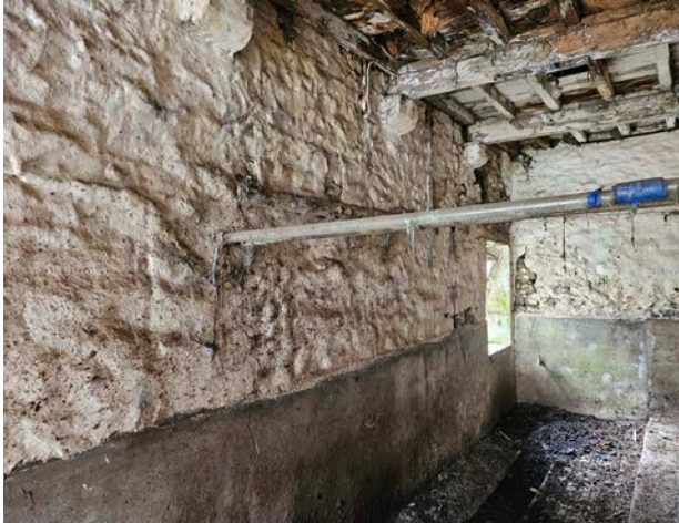
Figure 25 View of an additional room used for housing livestock
