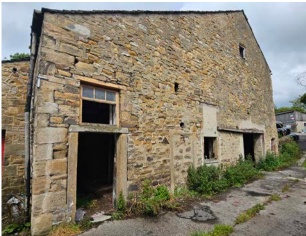
Figure 9 South facing elevation of Cockshotts Barn
