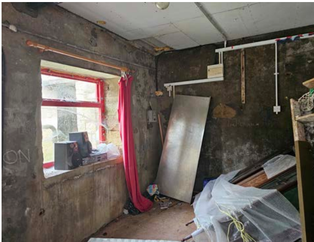
Figure 33 Internal view of a probable storage room
