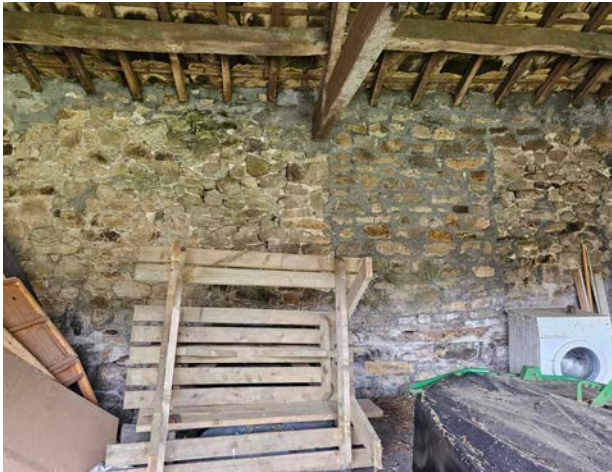
Figure 4 Interior of the remains of the Heyhouses Cottages
