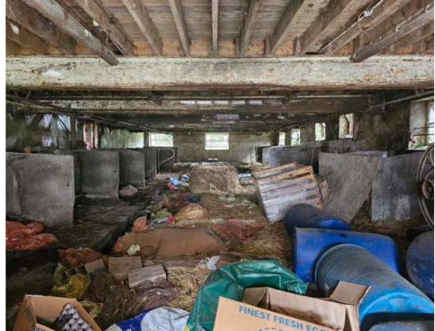
Figure 14 General view of the main cowhouse section of the barn
