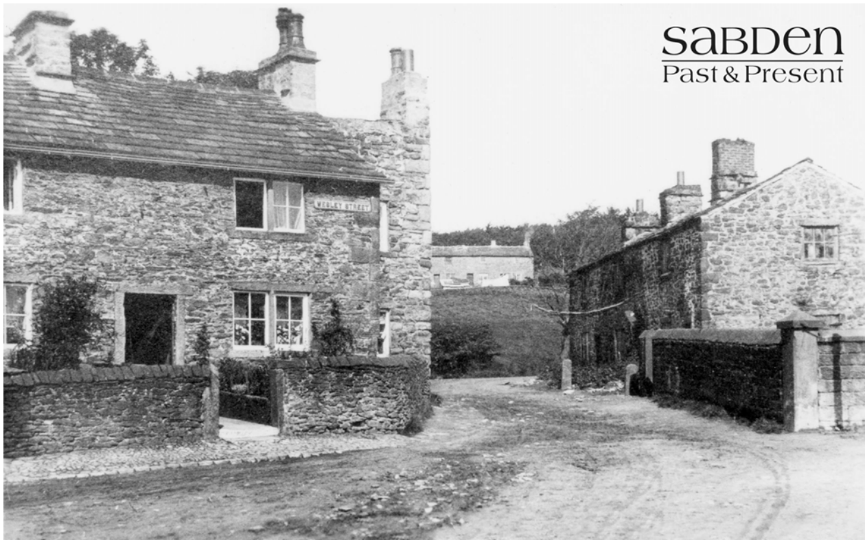
Figure 56 Heyhouses Cottages c.1900 (Source - Sabden Past and Present 2023)
