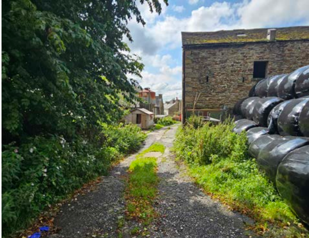
Figure 37 View of the east facing elevation of Cockshotts Barn
