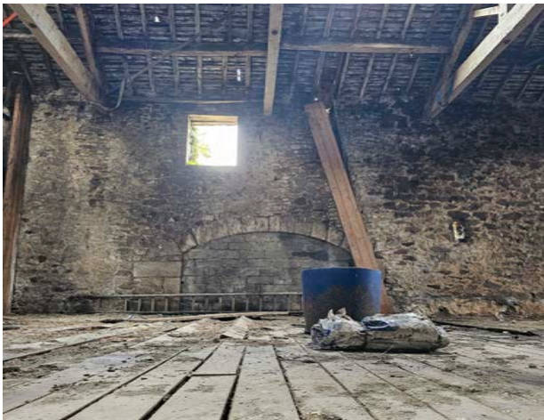
Figure 27 View of the first floor
