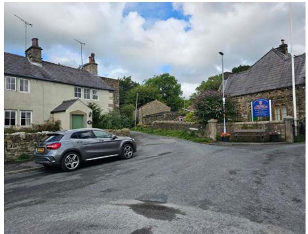
Figure 40 View of Cockshotts Barn from Stubbins Lane
