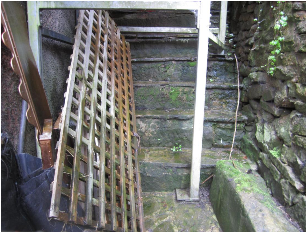
1 Existing stone steps beneath the timber stairs.
