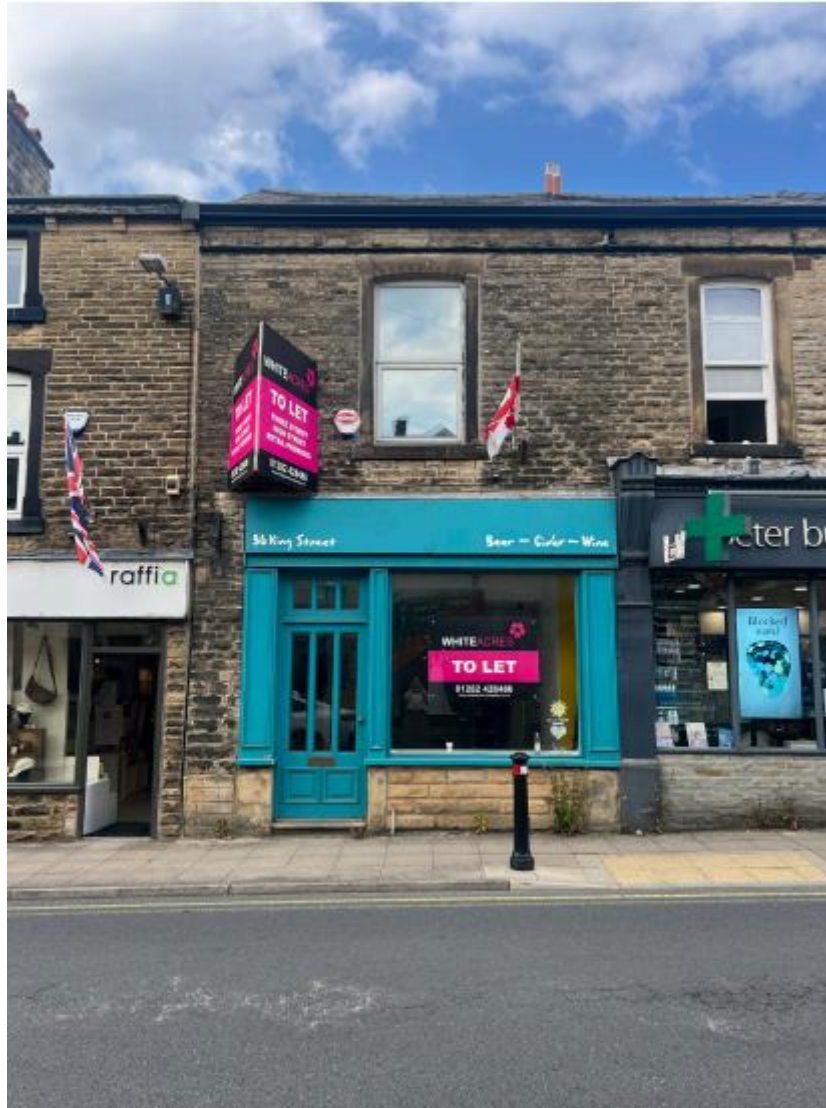
Figure 1 Existing appearance of 36 King Street, Clitheroe
