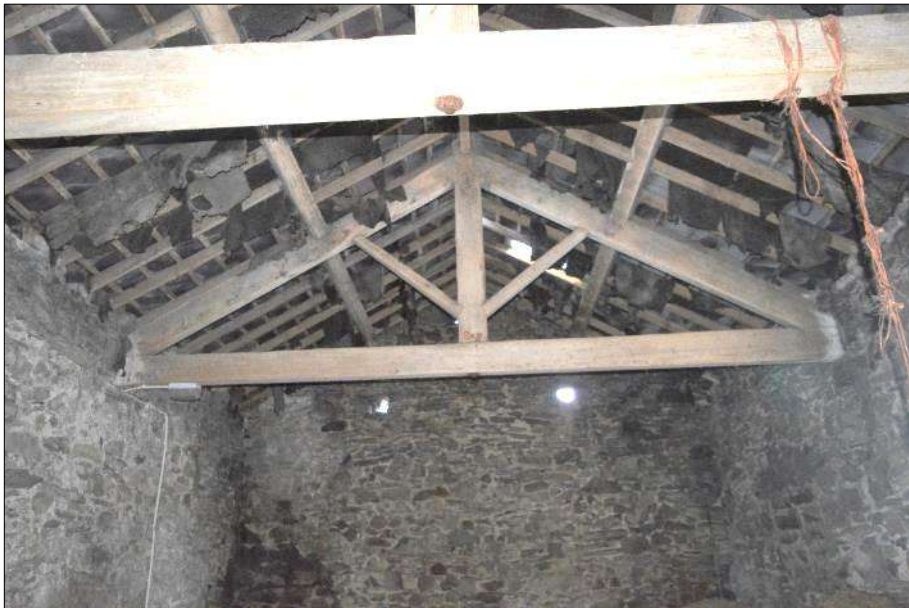
Plate 80 (shot 27): Kingpost roof truss, looking northwest
