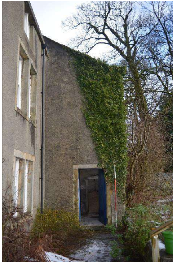
Plate 49 (shot 122): The southwest entrance to extension (A2), looking east-northeast, 2m scale
