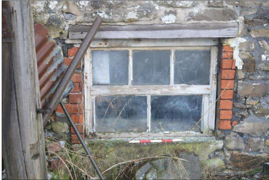
Plate 72 (shot 49): Repaired ground floor window, looking northeast, 0.5m scale
