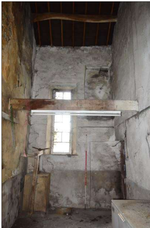
Plate 54 (shot 130): General view towards the staircase window, looking south-southeast, 2m scale
