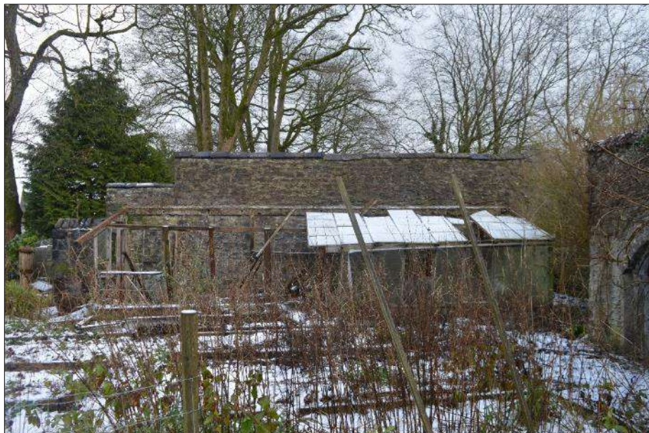
Plate 65 (shot 71): Southwest elevation of cart shed and storage, looking east-northeast
