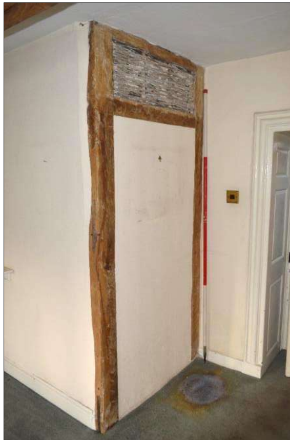
Plate 20 (shot 165): Blocked doorway to pantry with wattled panel above, looking west-northwest, 1m scale
