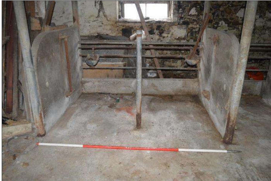
Plate 76 (shot 18): Representative shot of a two bay stall with galvanised drinkers and tethering bars (right hand side removed), looking southwest, 2m scale
