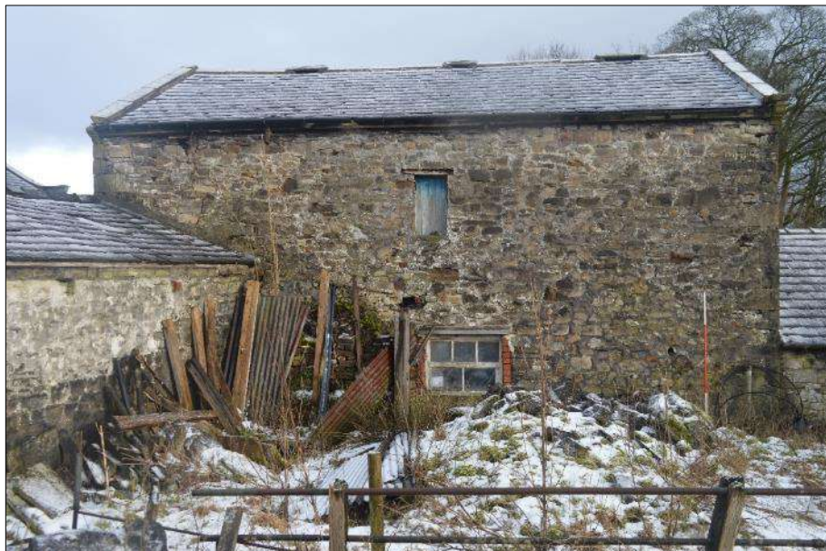
Plate 71 (shot 48): Southwest elevation, looking northeast, 2m scale
