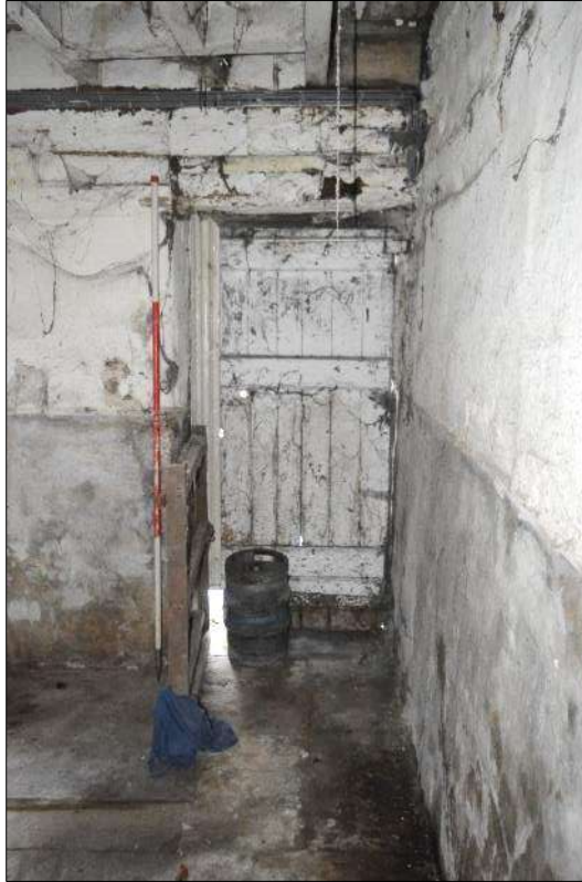
Plate 78 (shot 15): Early 19 th century style plank and batten door with beaded narrow planks, looking northeast, 2m scale
