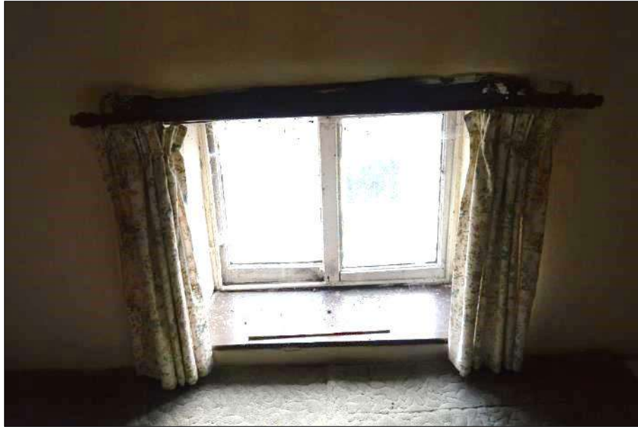
Plate 42 (shot 215): View of vertical sash in room (3.1), looking south-southeast, 1m scale
