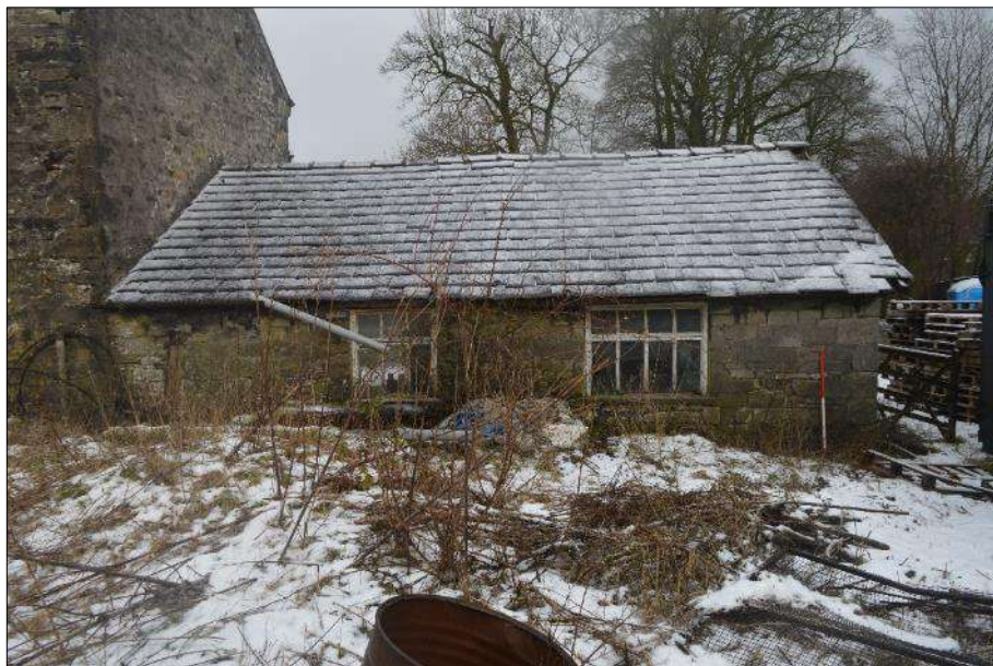
Plate 84 (shot 45): Southwest elevation, looking northeast, 1m scale
