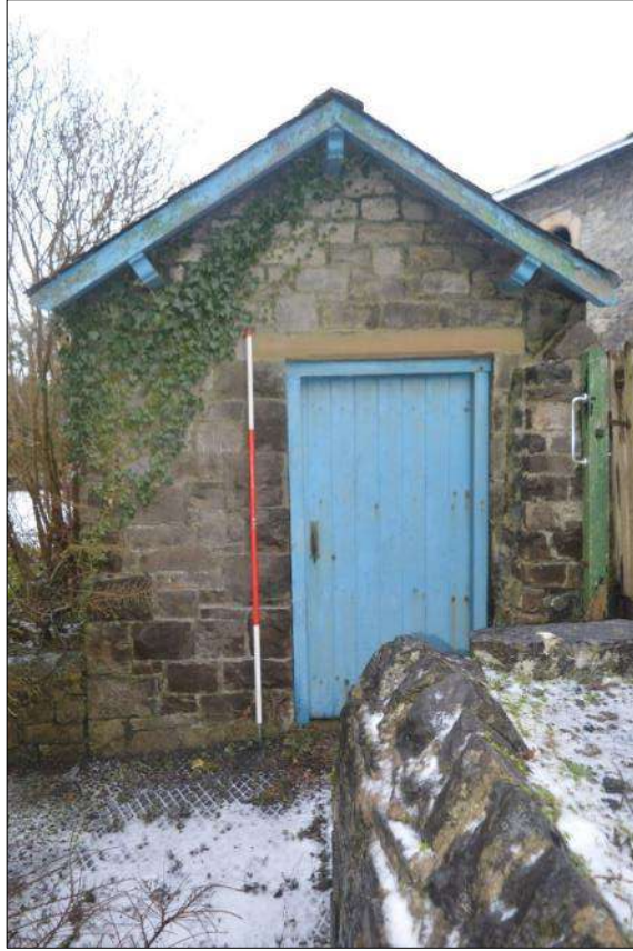
Plate 60 (shot 62): The coalhouse southwest of the farmhouse, looking south-southeast, 2m scale
