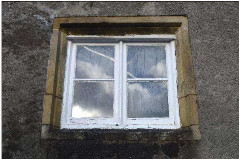
Plate 9 (shot 109): Close up of first floor window with moulded surround, looking north-northwest
