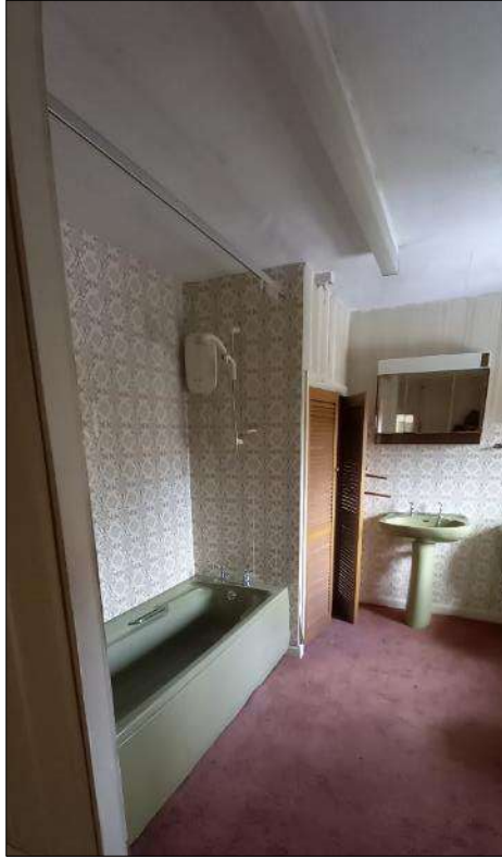
Plate 32 (shot 193): General view of first-floor bathroom (2.1), looking southwest
