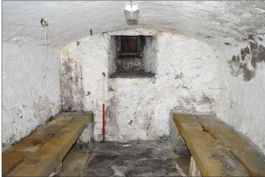
Plate 13 (shot 233): General view of the cellar, looking east-northeast, 1m scale
