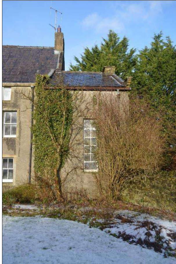
Plate 50 (shot 111): Southeast elevation of extension (A2), looking north-northwest
