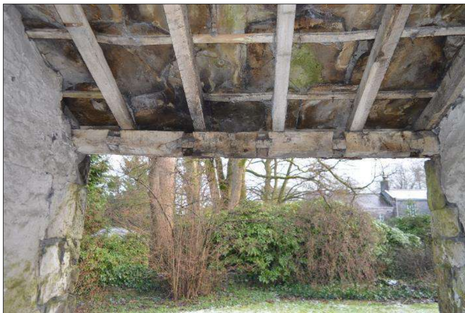
Plate 67 (shot 81): Reused main beam as wall plate, looking northeast
