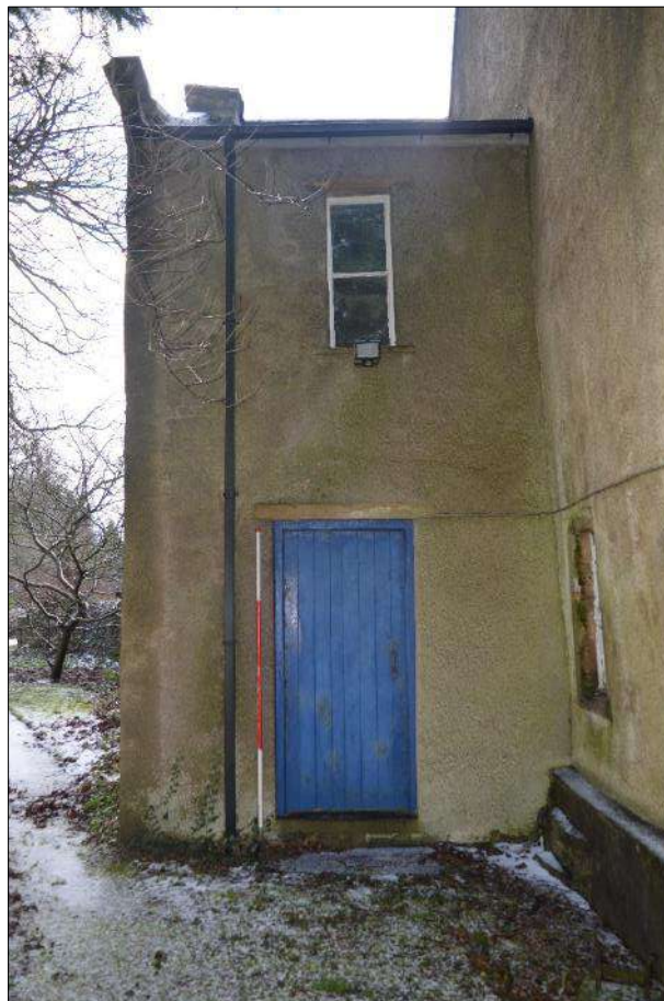
Plate 48 (shot 85): Northwest elevation, looking south-southeast, 2m scale
