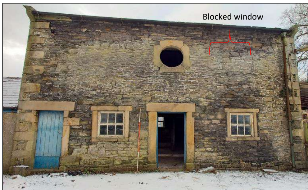
Plate 69 (shot 241): Northeast elevation of the byre, looking southwest, 2m scale
