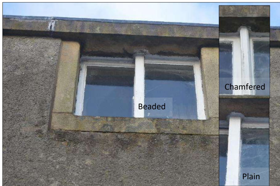
Plate 11 (shots 117, 121 and 115): Second floor Yorkshire sashes with variation of mullions, looking north-northwest
