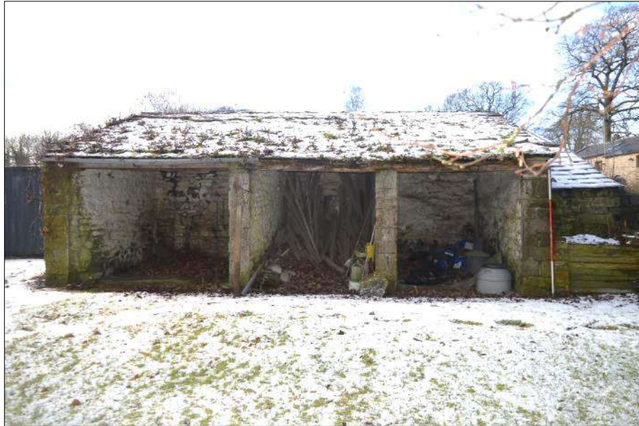
Plate 64 (shot 76): Cart shed/animal shelter, looking southwest, 2m scale
