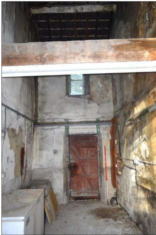
Plate 52 (shot 130): View of extension, looking south-southeast, 2m scale
