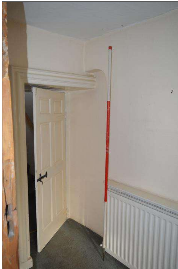
Plate 21 (shot 166): Doorway between the corridor and the living room (1.2), notice empty mortices for a possible strike plate on the post to the left, looking north-northeast, 2m scale
