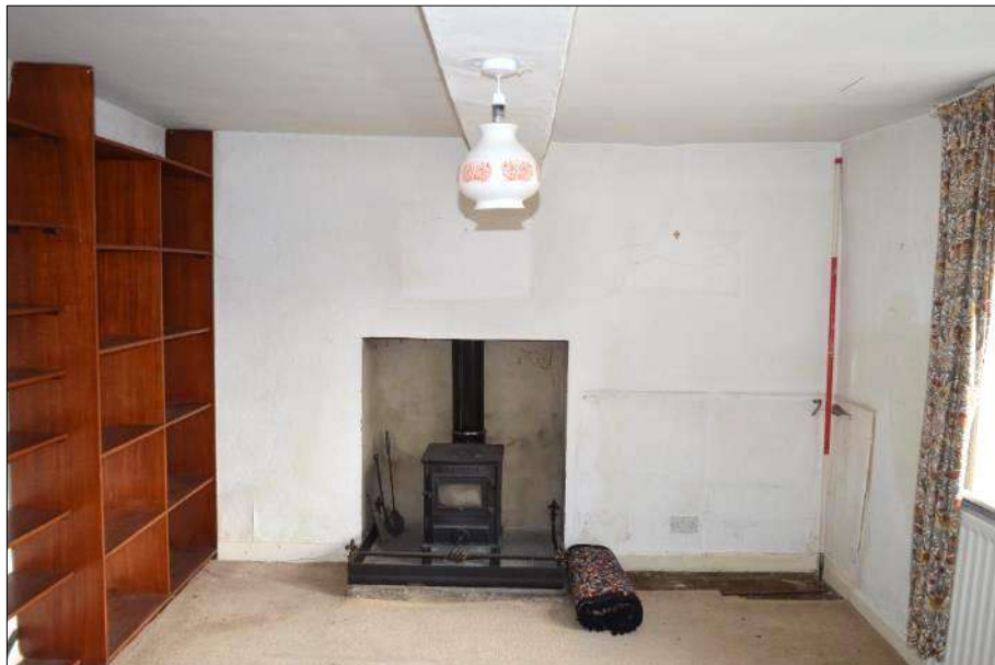
Plate 25 (shot 169): General view of sitting room (1.3) with wood burner in former fireplace, looking east-northeast, 2m scale
