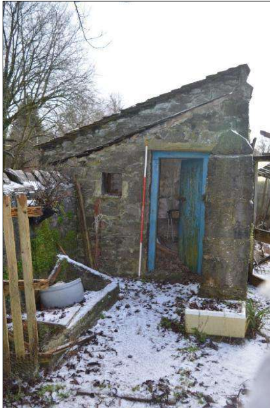
Plate 66 (shot 74): Small storage abutting the northwest wall, looking south-southeast, 2m scale
