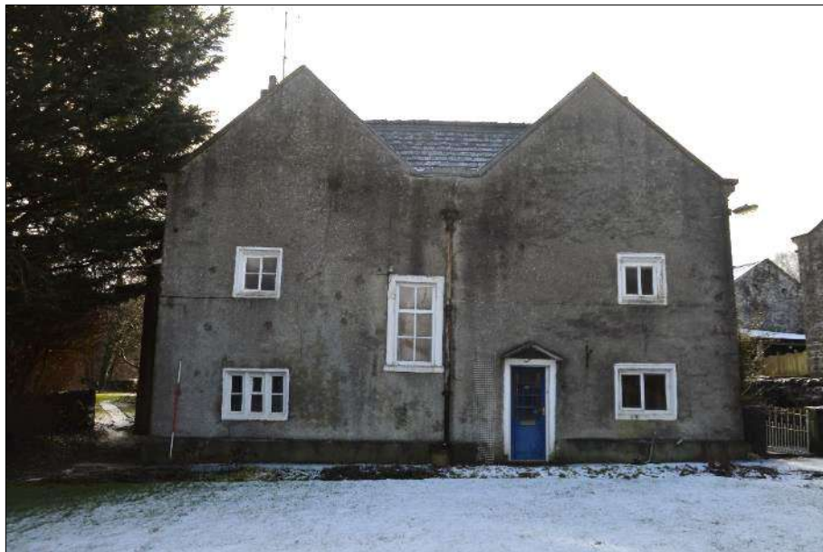
Plate 1 (shot 94): Northwest elevation of the farmhouse, looking south-southeast, 2m scale
