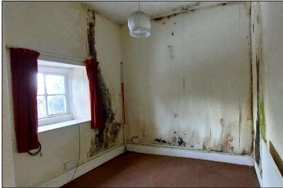
Plate 38 (shot 209): General view of bedroom (2.5), looking northeast, 2m scale
