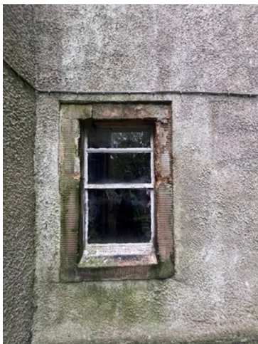
Fig: 7 Example of window in complete disrepair & example replacement in timber painted finish in RAL 7006 (Beige Grey)
