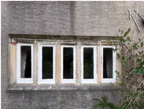
Fig: 9 Example original 17 th century window to be replaced with Altherm Heritage (or similar) aluminium to mimic the original 17 th century style, but offering modern energy efficiency finished in RAL 7006 (Beige Grey)
