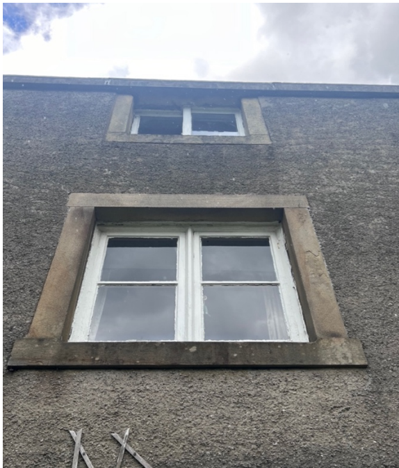
Fig: 4 Example of existing stone surround to be retained and cleaned
