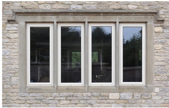
Fig: 9 Example original 17 th century window to be replaced with Altherm Heritage (or similar) aluminium to mimic the original 17 th century style, but offering modern energy efficiency finished in RAL 7006 (Beige Grey)
