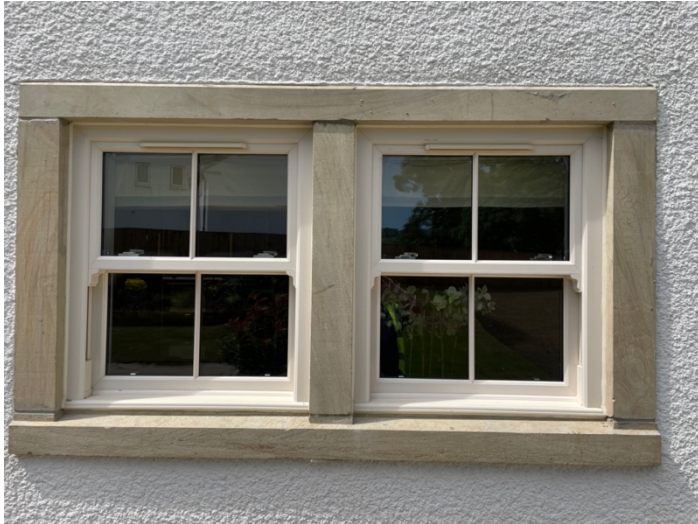
Fig: 6 Example of replacement natural stone window surround set in render. (Example of materials, actual stone will be made to replicate the original profile)
