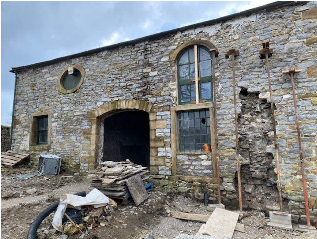
Image 2 – Natural stone walls and mixture of slate/stone flag roof
