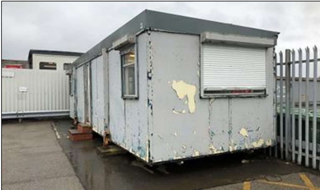
Plate 6: The buildings on site, including Building 128, were a selection of demountable structures and a steel portal frame building.
