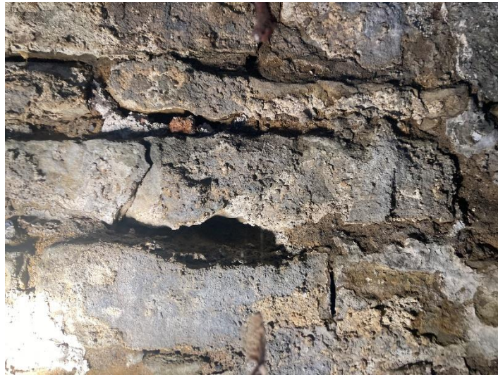
Figure 6 Showing Internal Crevices within Stonework
