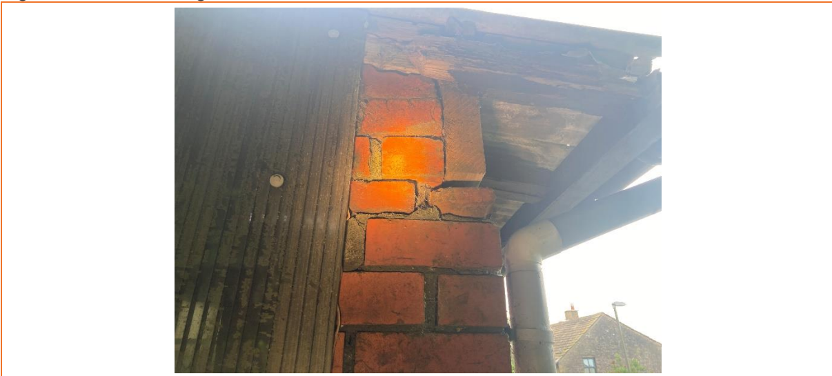
Figure 3 Showing Crevices on the Western Elevation
