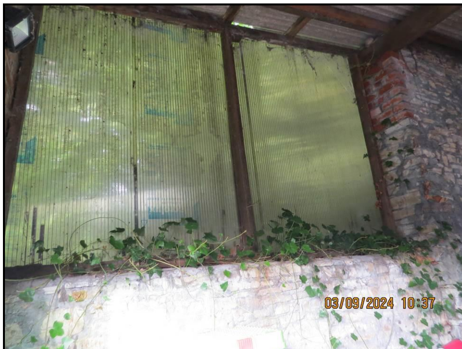
028 Double panel Perspex window
