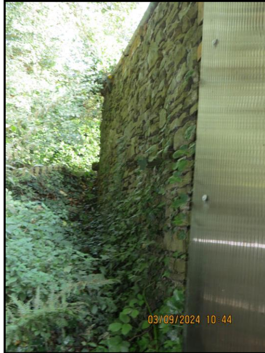
Photograph 031 North West flank, localised disturbance to outer leaf
