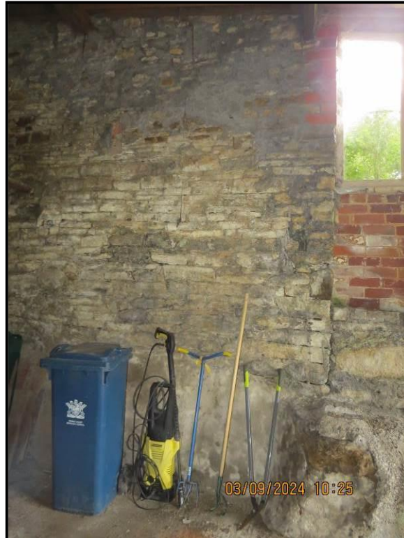
013 Construction joint between original barn and extended garage
