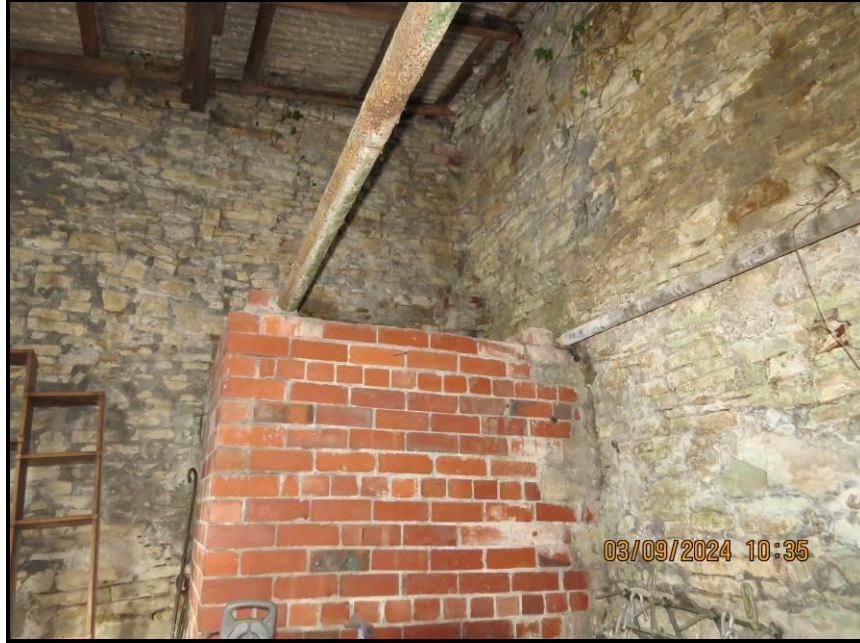
Photograph 024 Buttress support to steel struts
