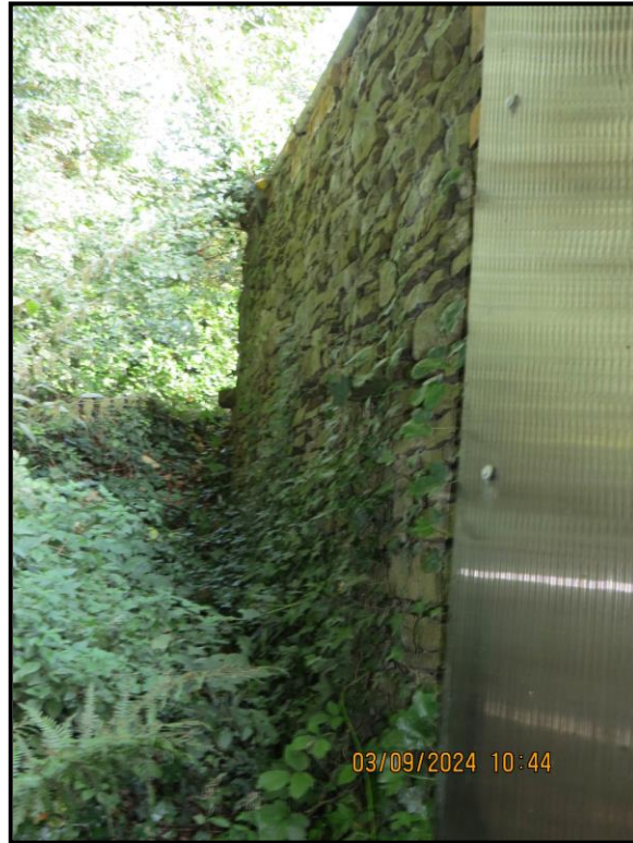
031 North Western flank, localised disturbance to outer leaf
