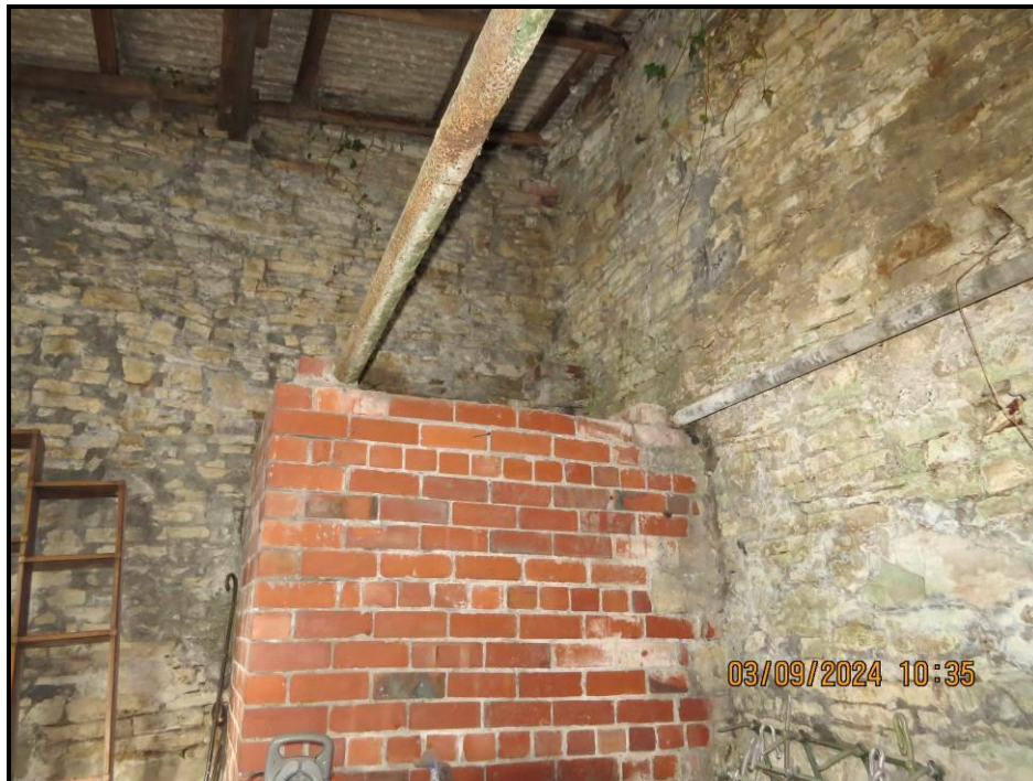
024 Buttress support to steel struts
