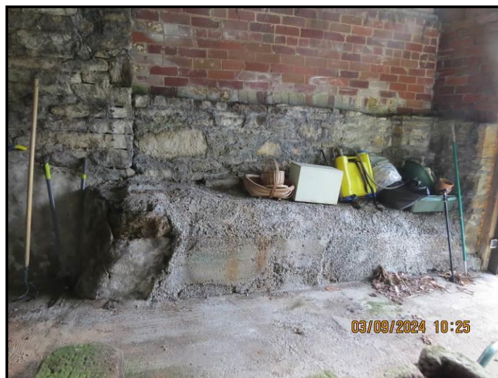
Photograph 015 Mixed plinth construction, chainage 0 – 3 metres (East)
