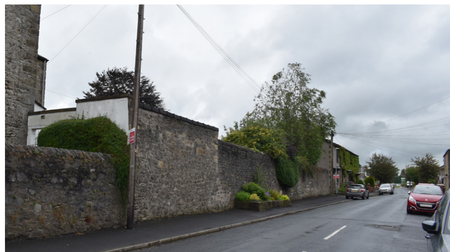
HM Land Registry and photograph of the east boundary wall
