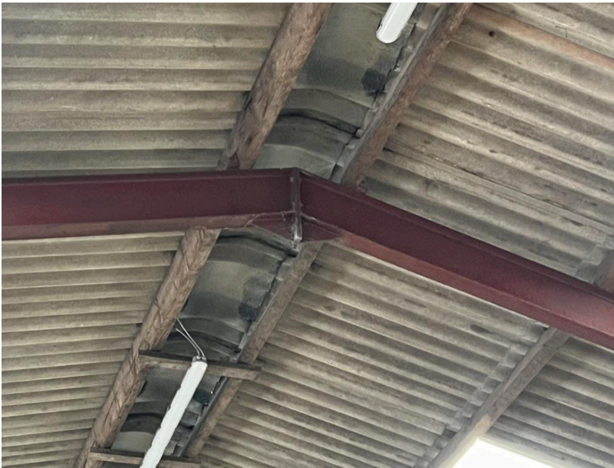
Photo 11 – Apex detail to frame
