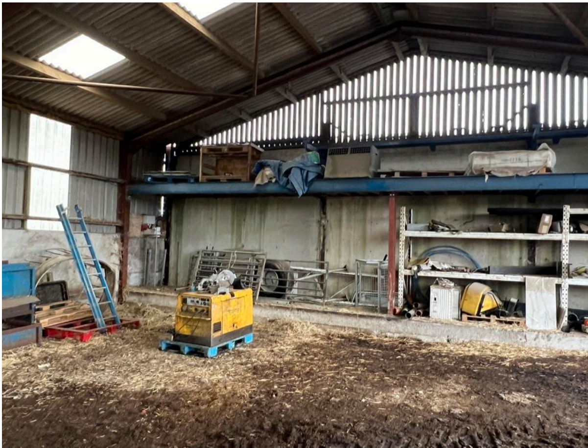
Photo 7 – West Gable (internal)
