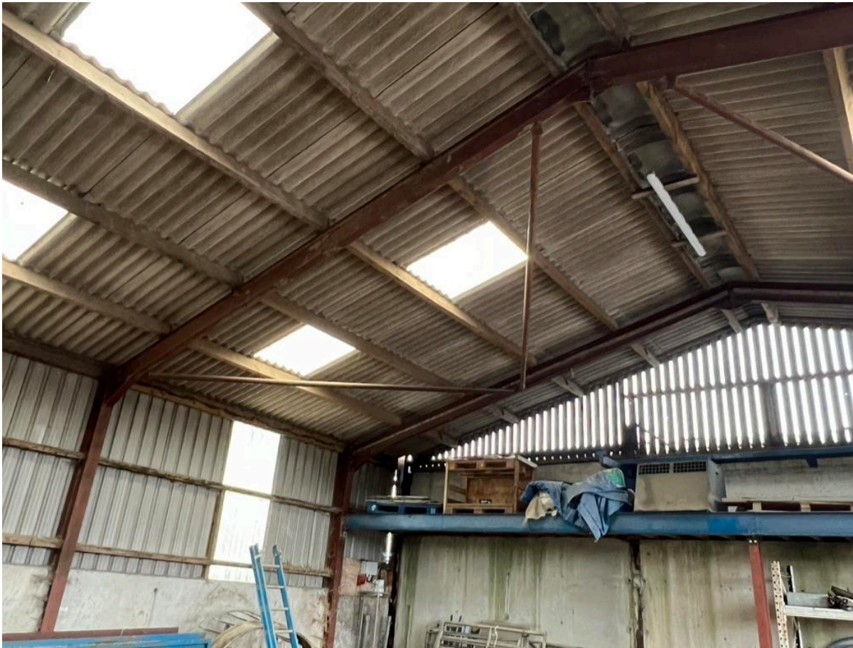
Photo 12 – Bracing to frames
