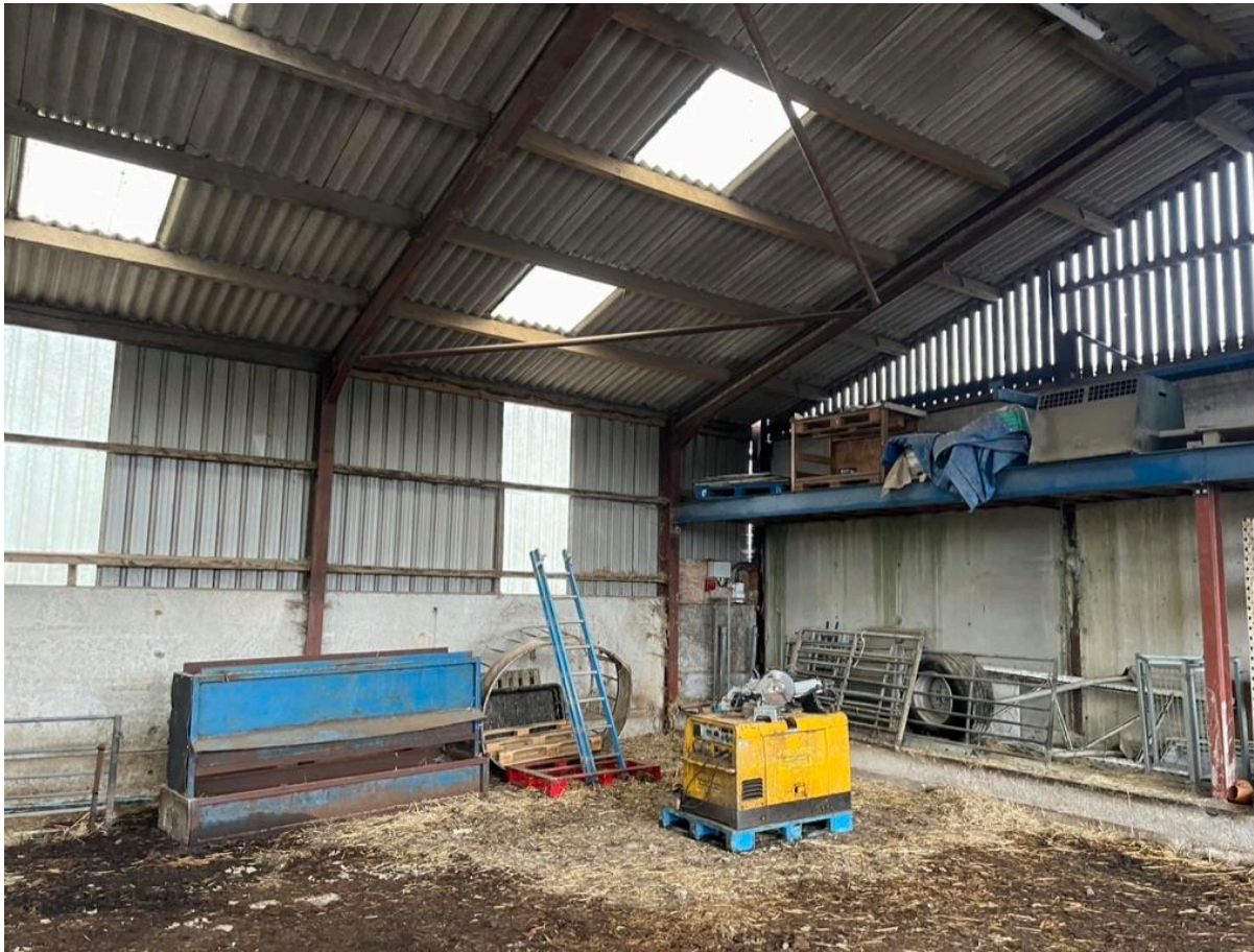
Photo 6 – South West Corner
