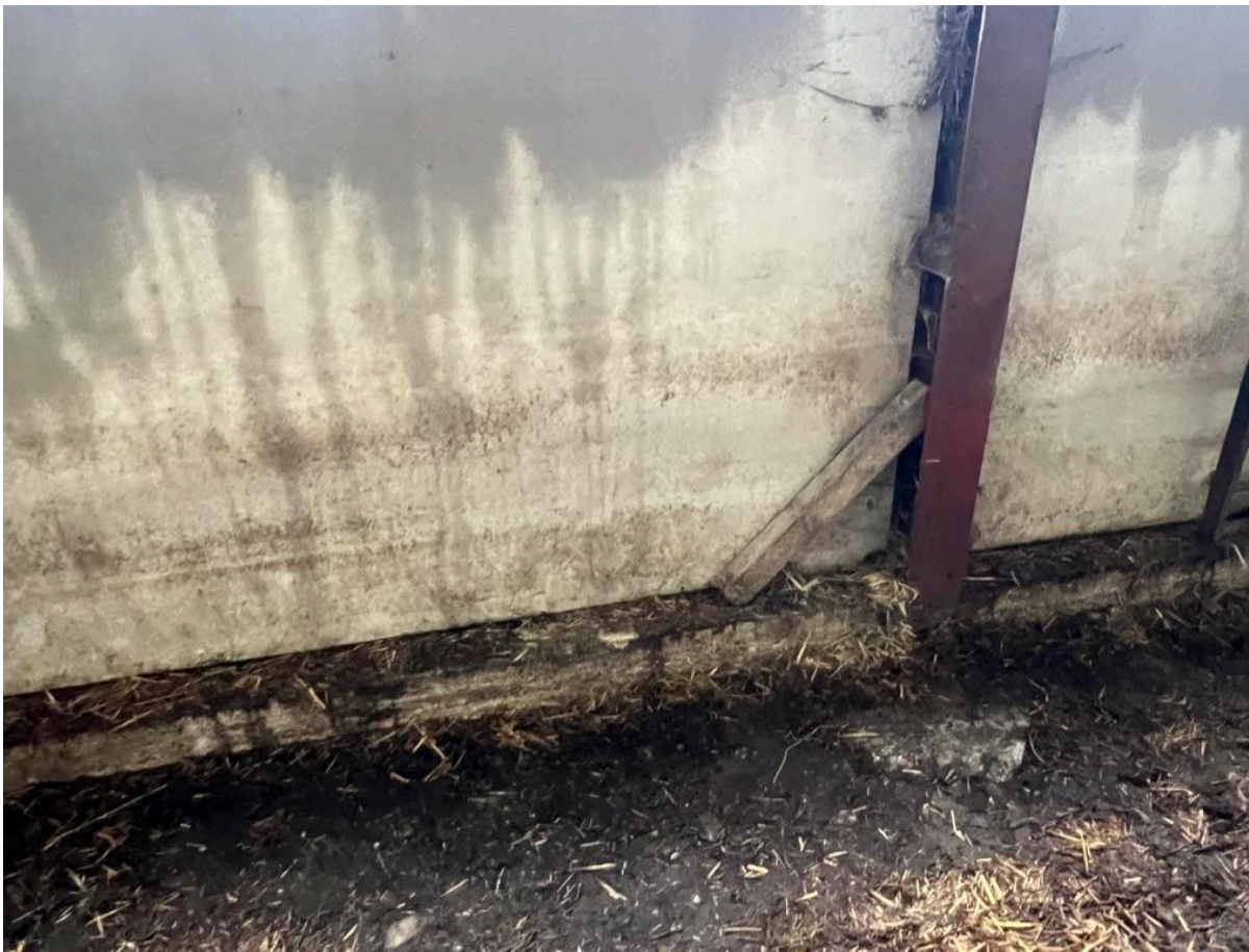
Photo 13 – Lower concrete wall
