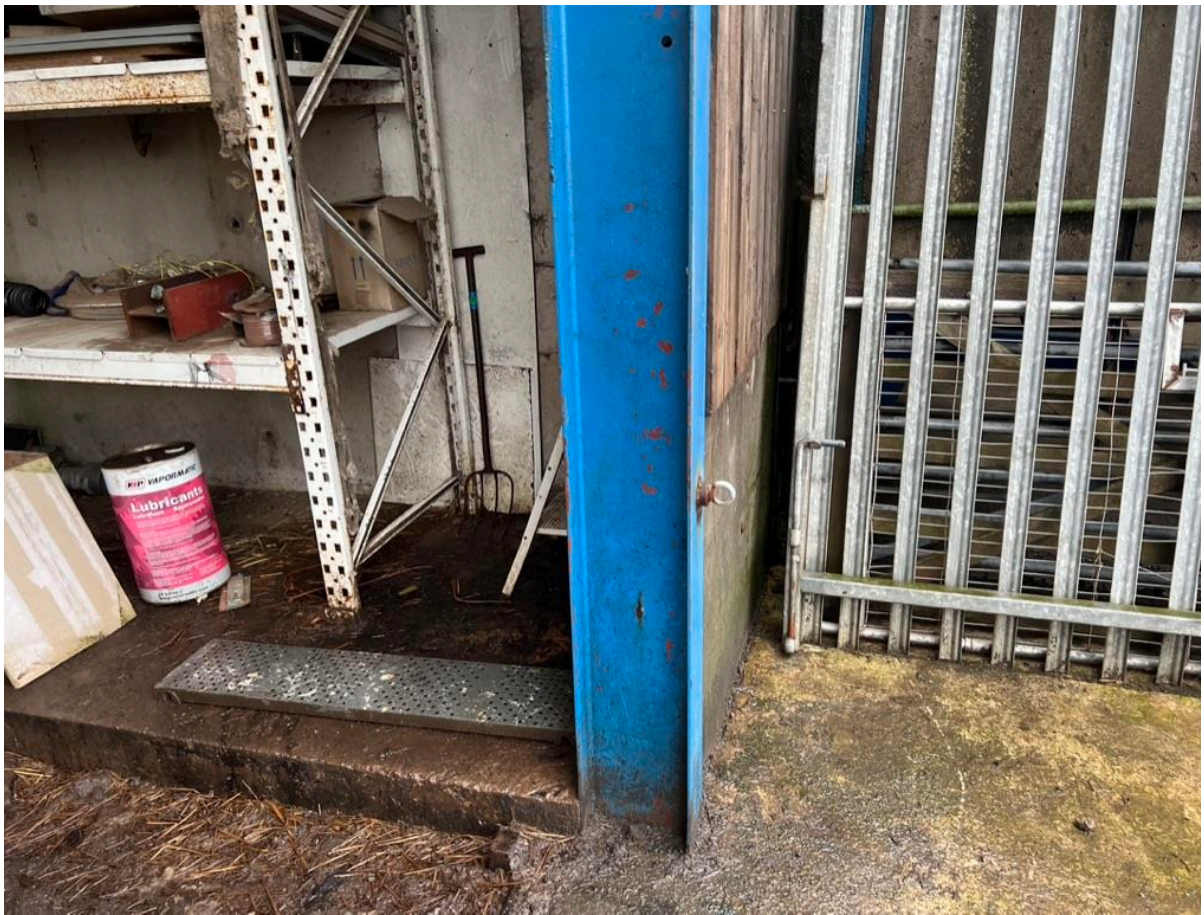
Photo 9 – Column to frame
