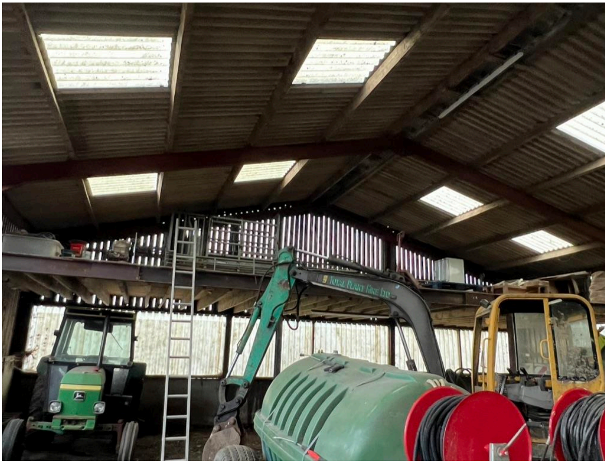
Photo 15 - East gable (internal)
