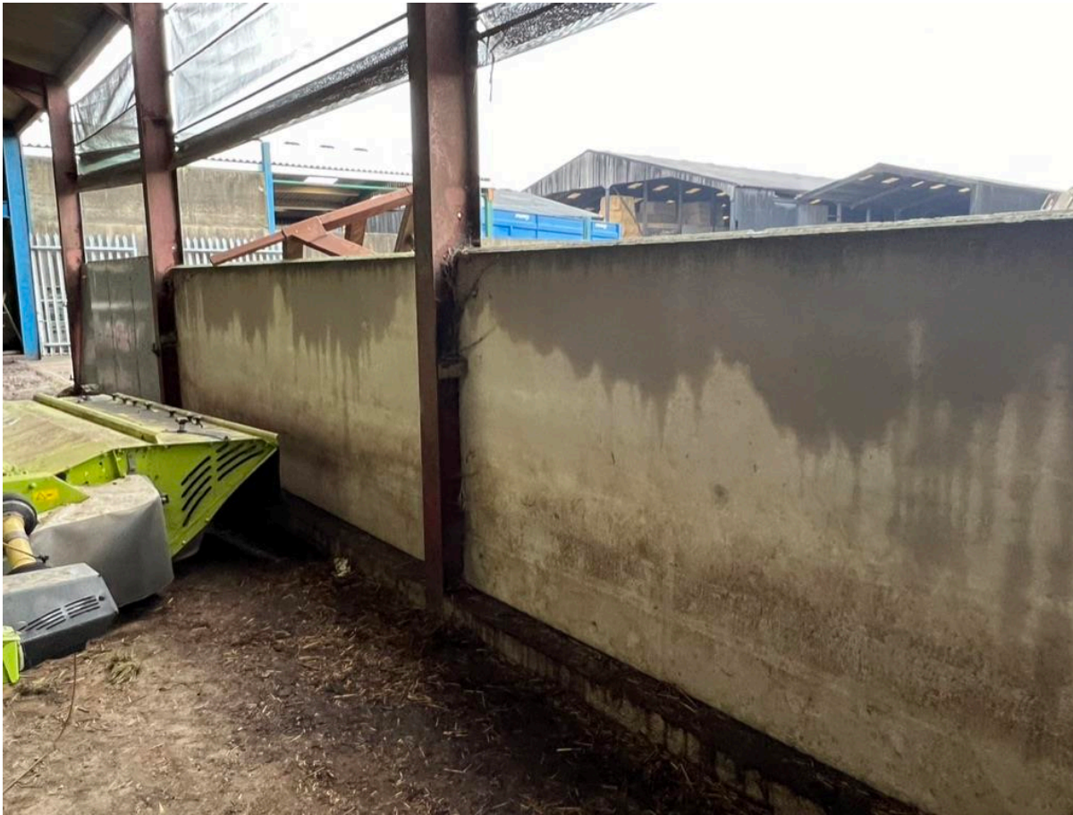
Photo 14 - North Elevation (internal)
