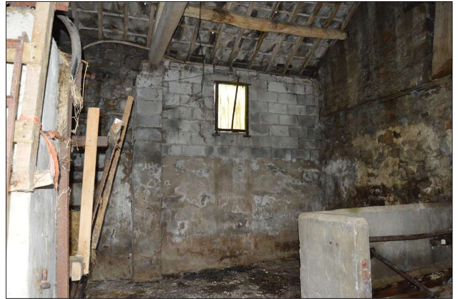
View 43: View of blocked up opening to the north west side for the south west addition.
