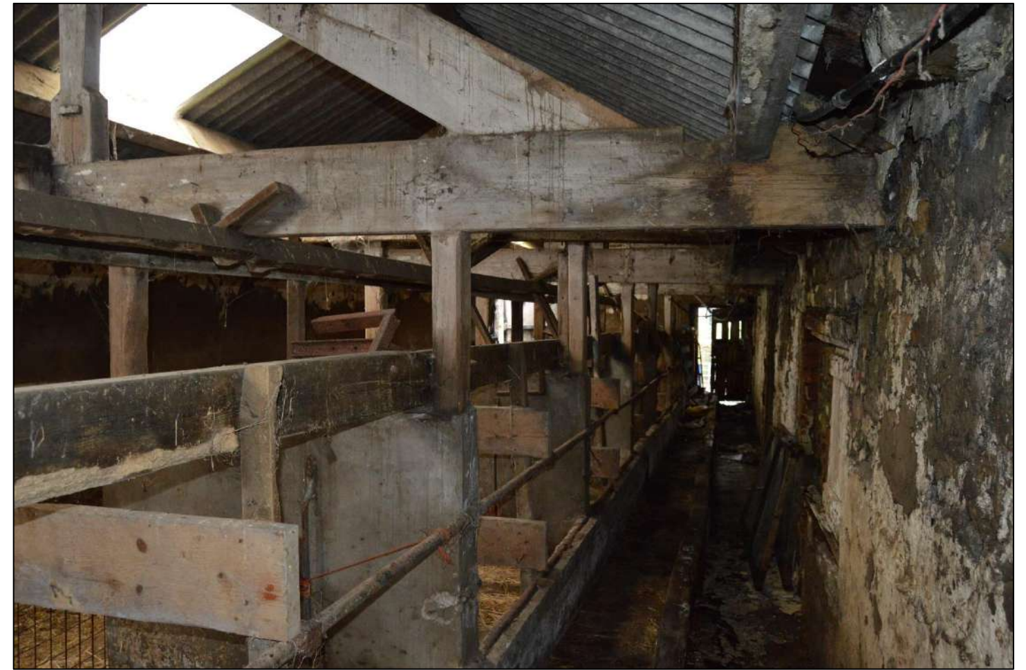
View 27: View north east within the shippon.
