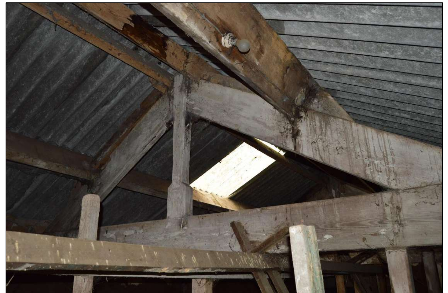
View 29: View of king post roof truss within the shippon.
