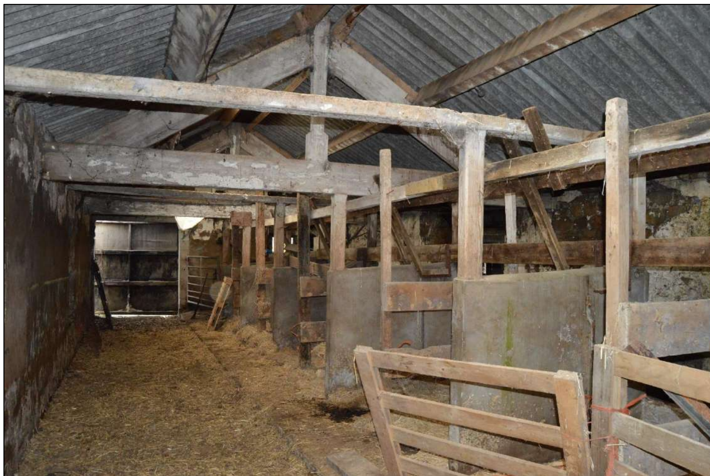
View 28: View north east within the shippon.
