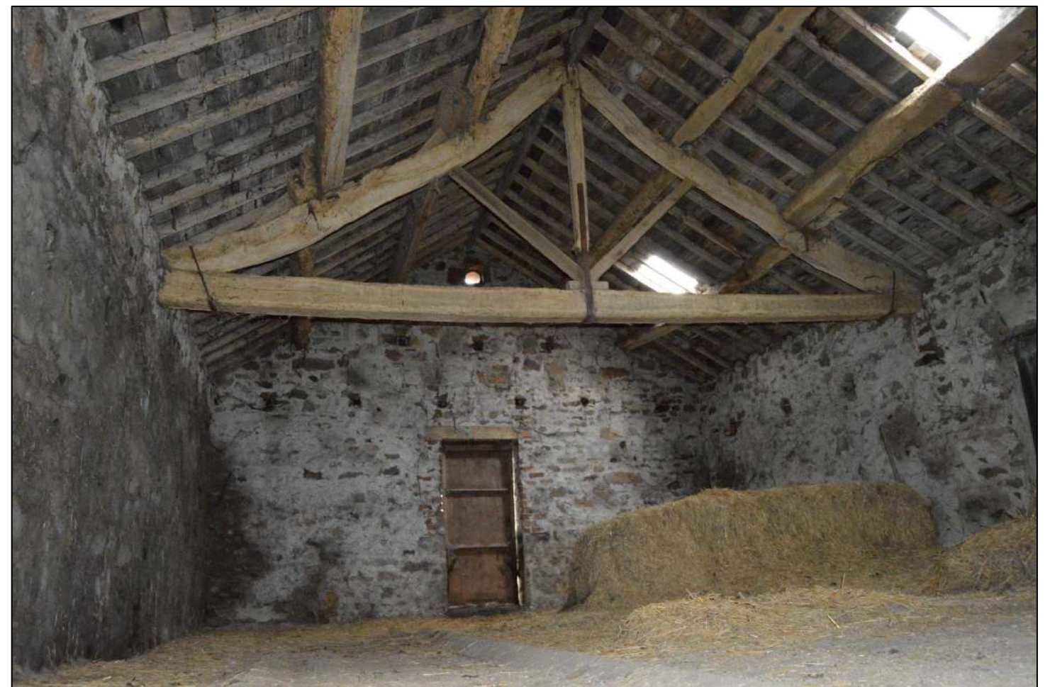
View 37: View north east above the hayloft.
