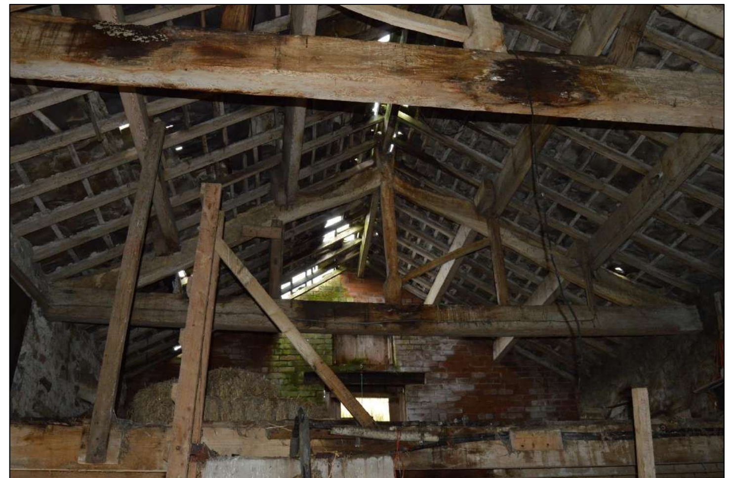
View 41: View of the timber king post roof truss to the south west addition of the barn.
