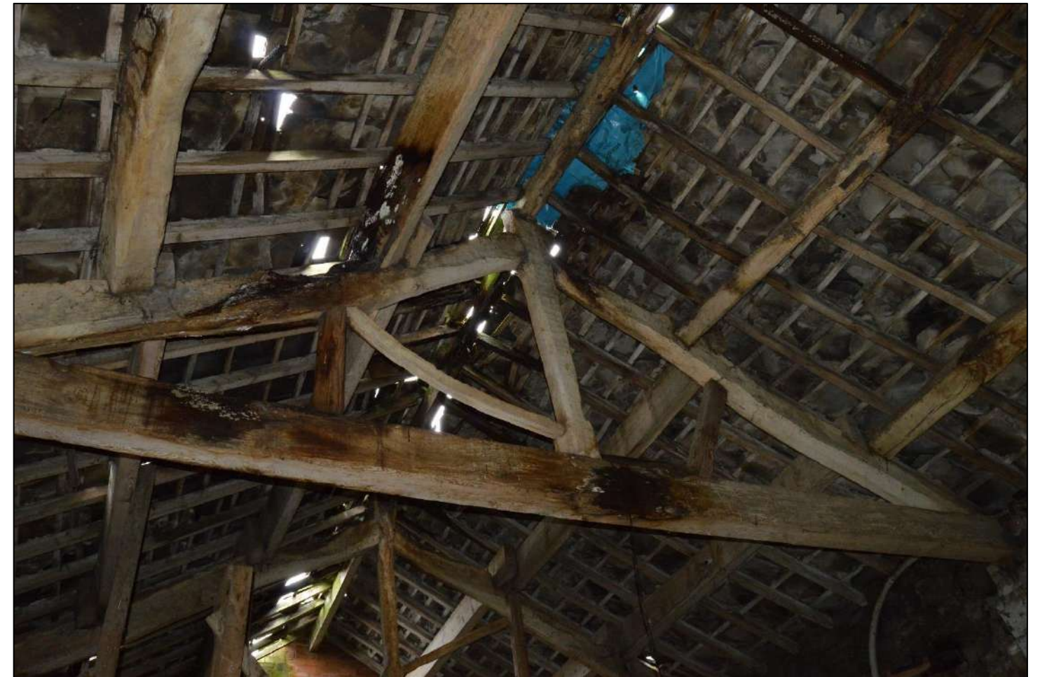
View 39: View of the timber king post roof truss to the south west addition of the barn.
