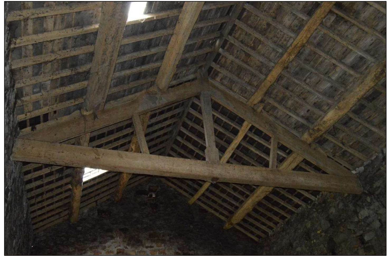
PL35: View of King Post roof truss to the south west end of the main barn.
