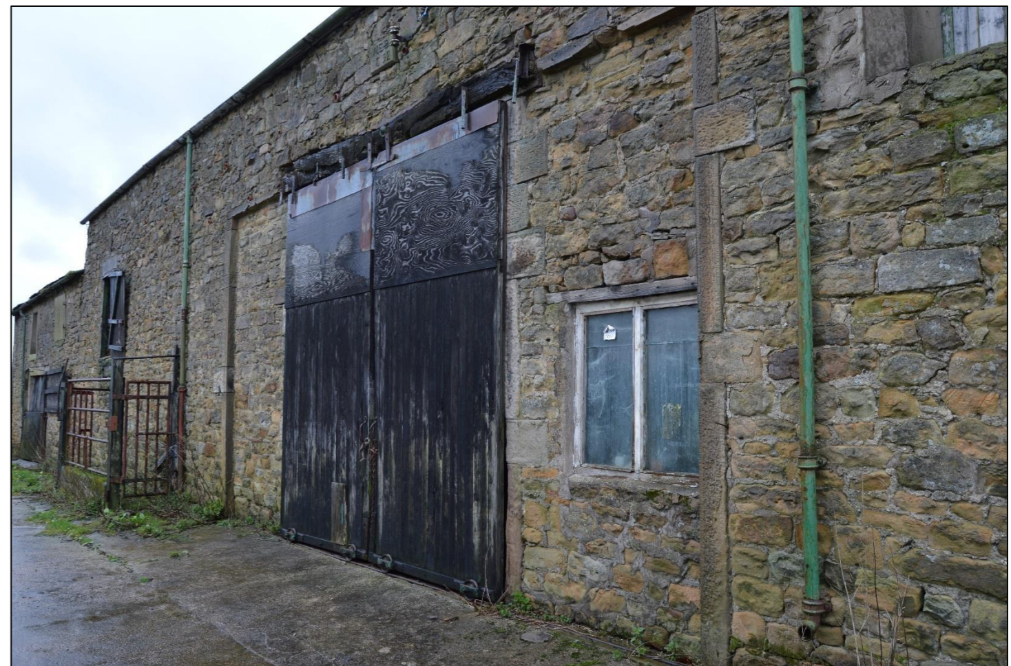
View 17: View of the existing 19 th century sliding cart entry door arrangement.
