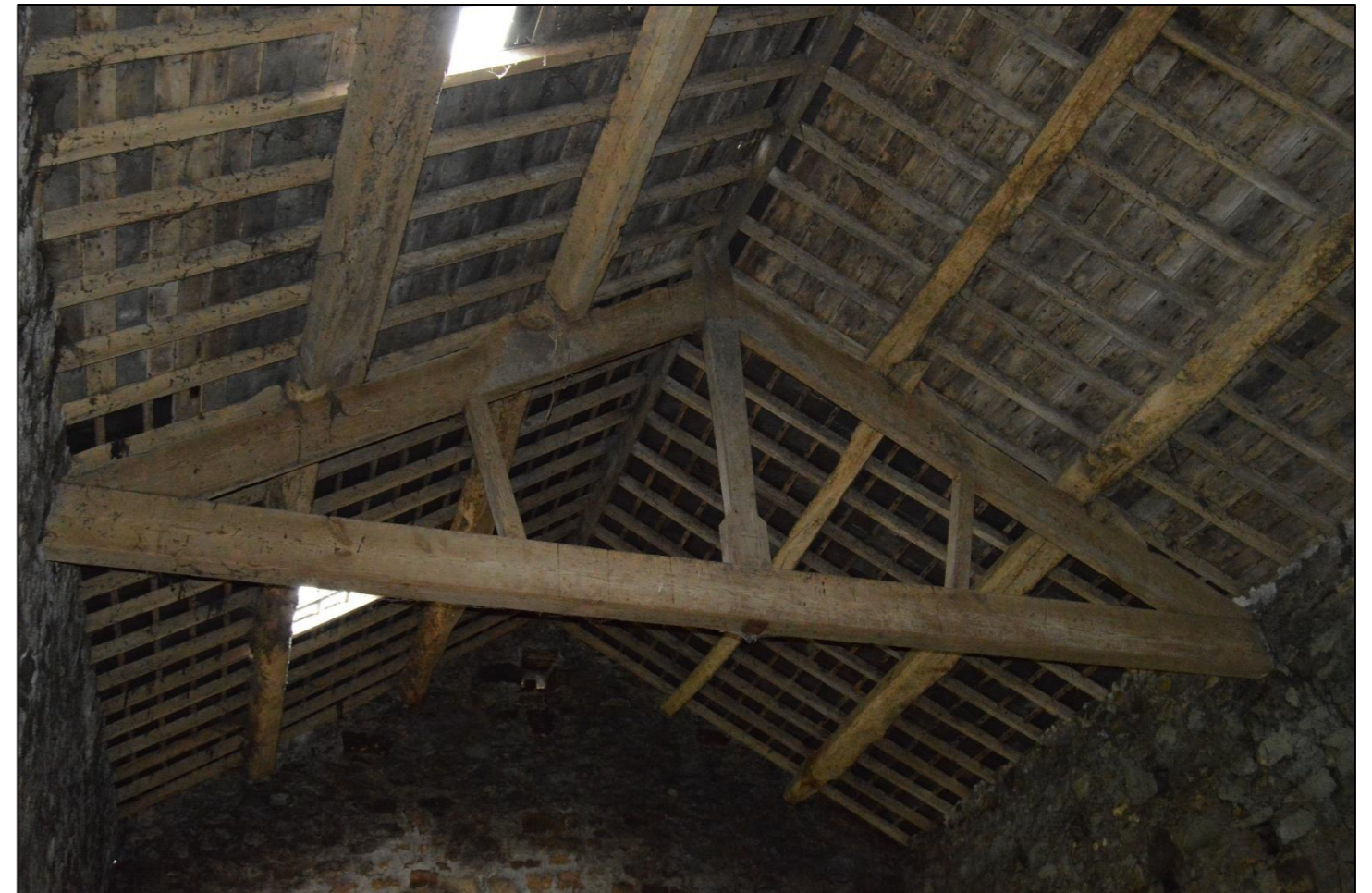
PL35: View of King Post roof truss to the south west end of the main barn.
