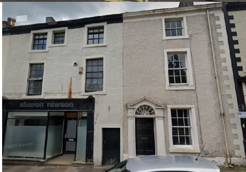
- Several examples of neighbouring properties on York Street with original or historic 12 pane Georgian timber sash windows and modern Georgian style 16 pane double glazed PVC or timber sash windows.
