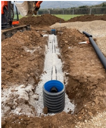
Installing drainage silt traps, Cheddar, Somerset
