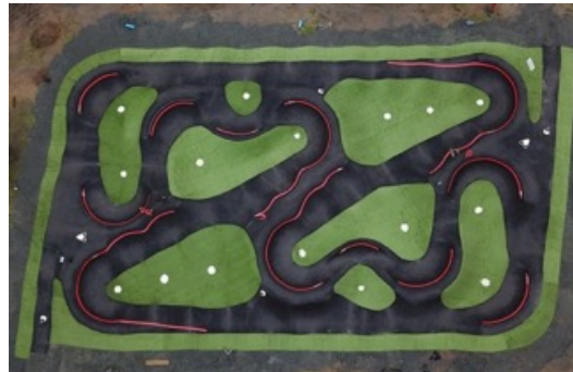
Painted Lines, Norway
