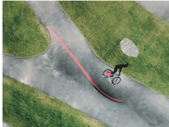
Clean drainage stone set away from track edge, Cathkin Braes, Glasgow
