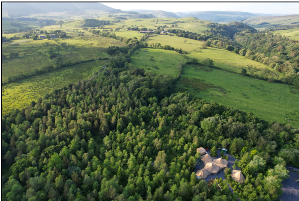
Image 2 – Wide oblique aerial view showing context of proposed development site. Wider landscape features shown include mixed plantation, broadleaved woodland, semi-improved and marshy grassland and rush pasture. June 2024
