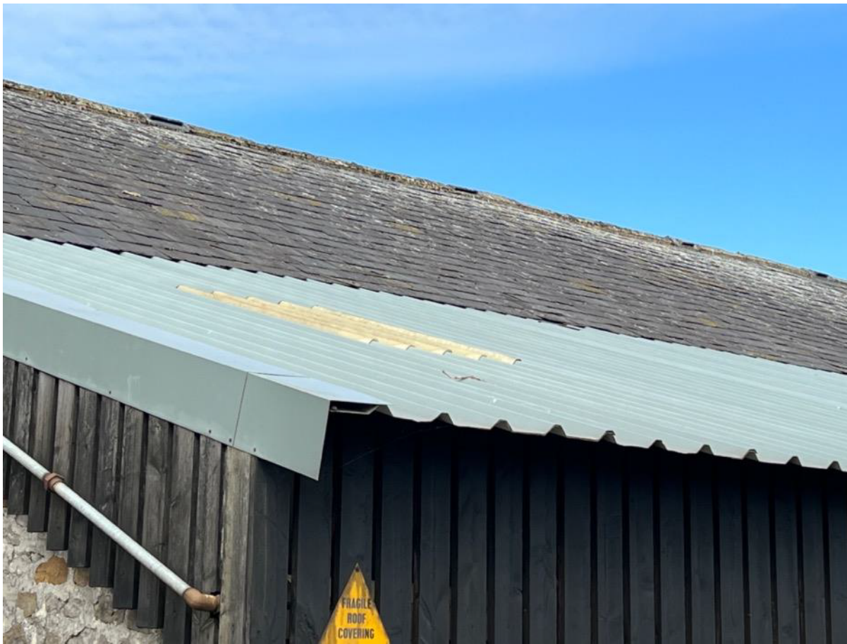
Photo 17 – Roof North East
