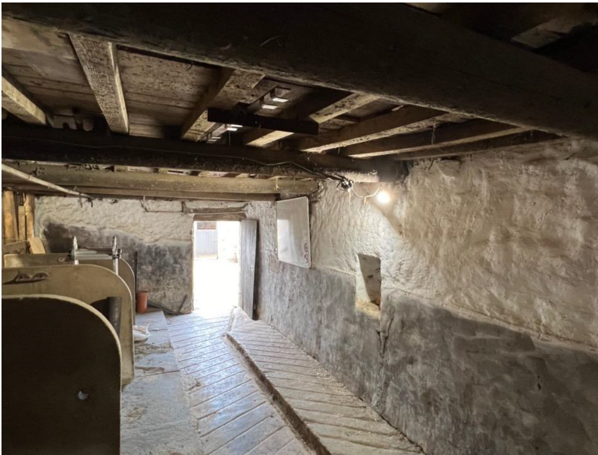
Photo 27 - Internal main barn – south east end
