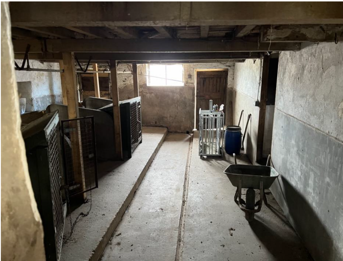
Photo 39 - Internal main barn – mid section
