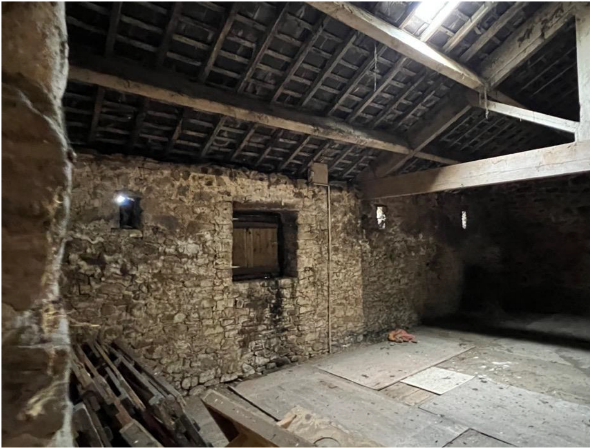
Photo 32 - Internal main barn – south west end
