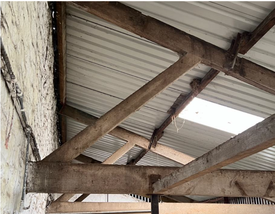
Photo 20 - Internal to rear single storey section – roof timbers
