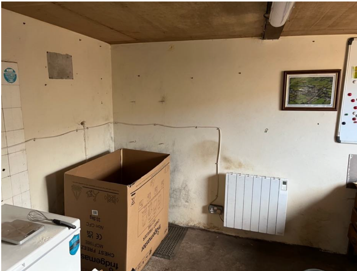
Photo 42 - Internal main barn – north west end
