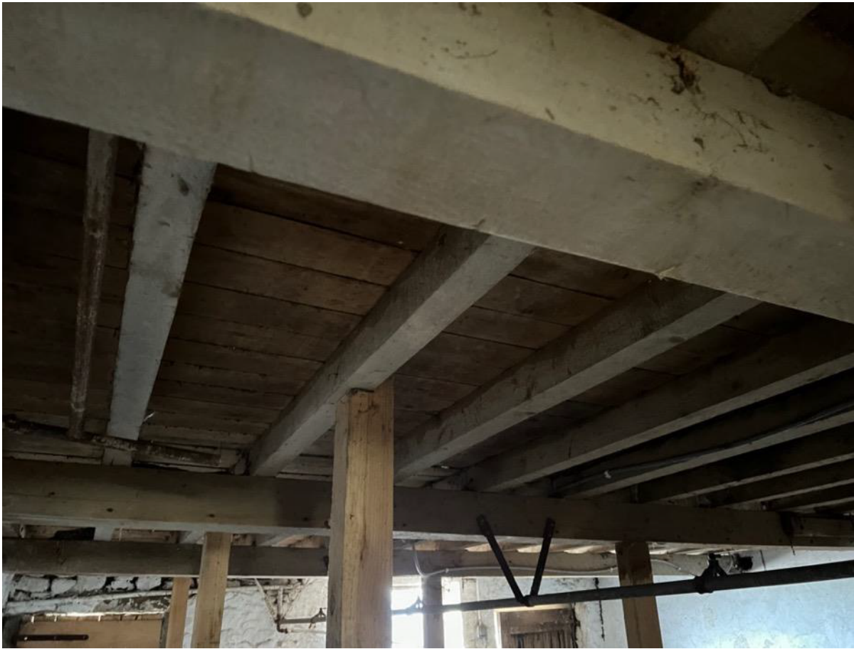
Photo 38 - Internal main barn – mid section – Floor to loft above
