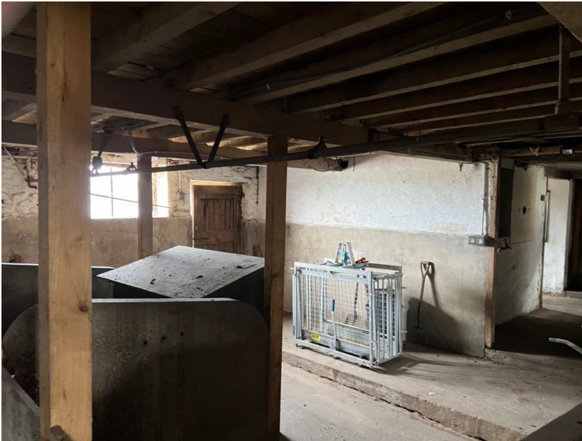
Photo 36 - Internal main barn – mid section
