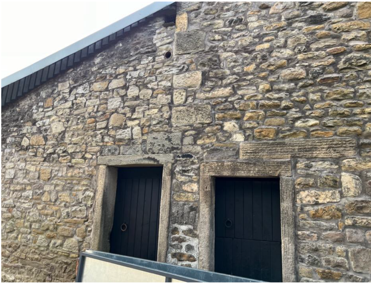
Photo 11 - North West Elevation
