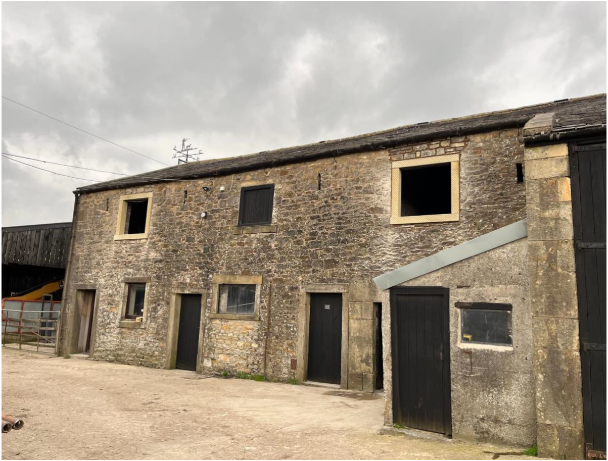
Photo 1 - South West Elevation
