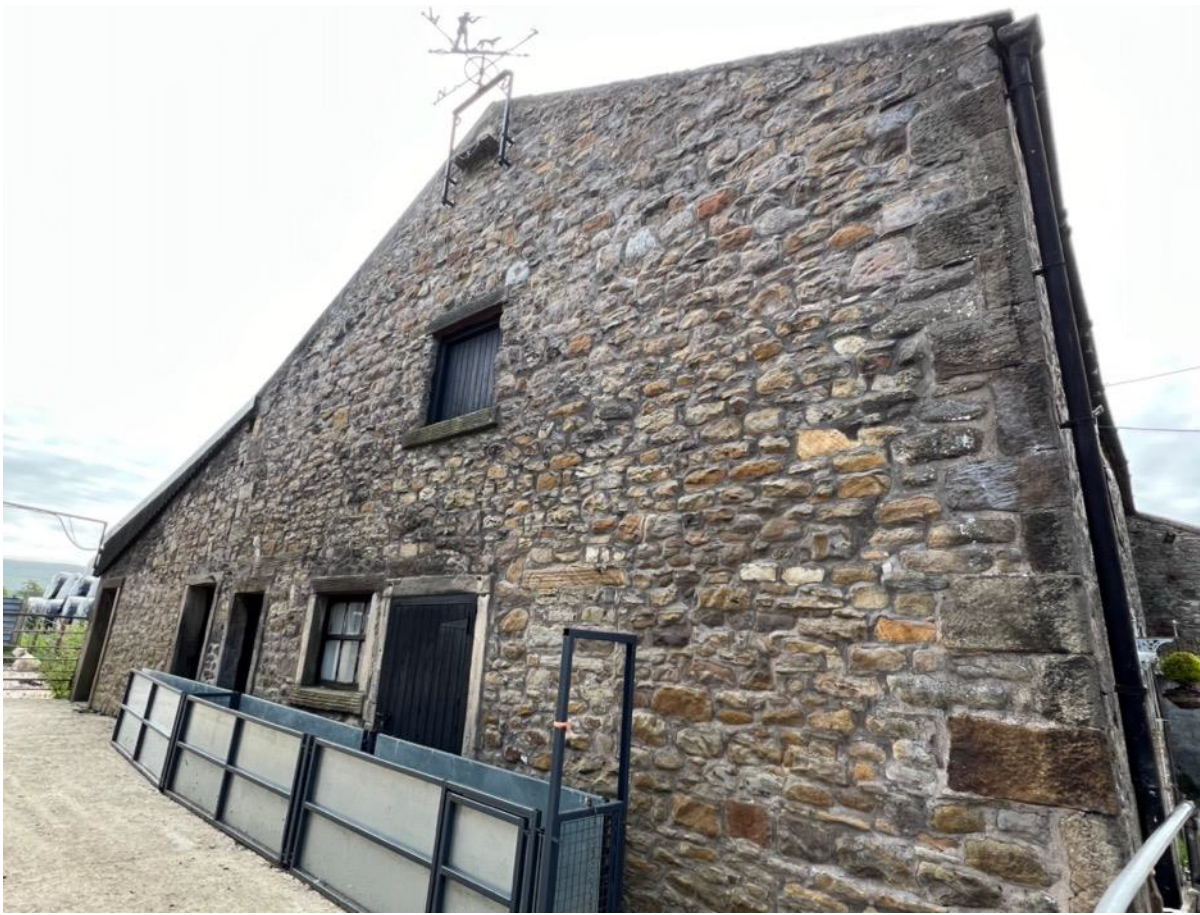
Photo 9 – North West Elevation
