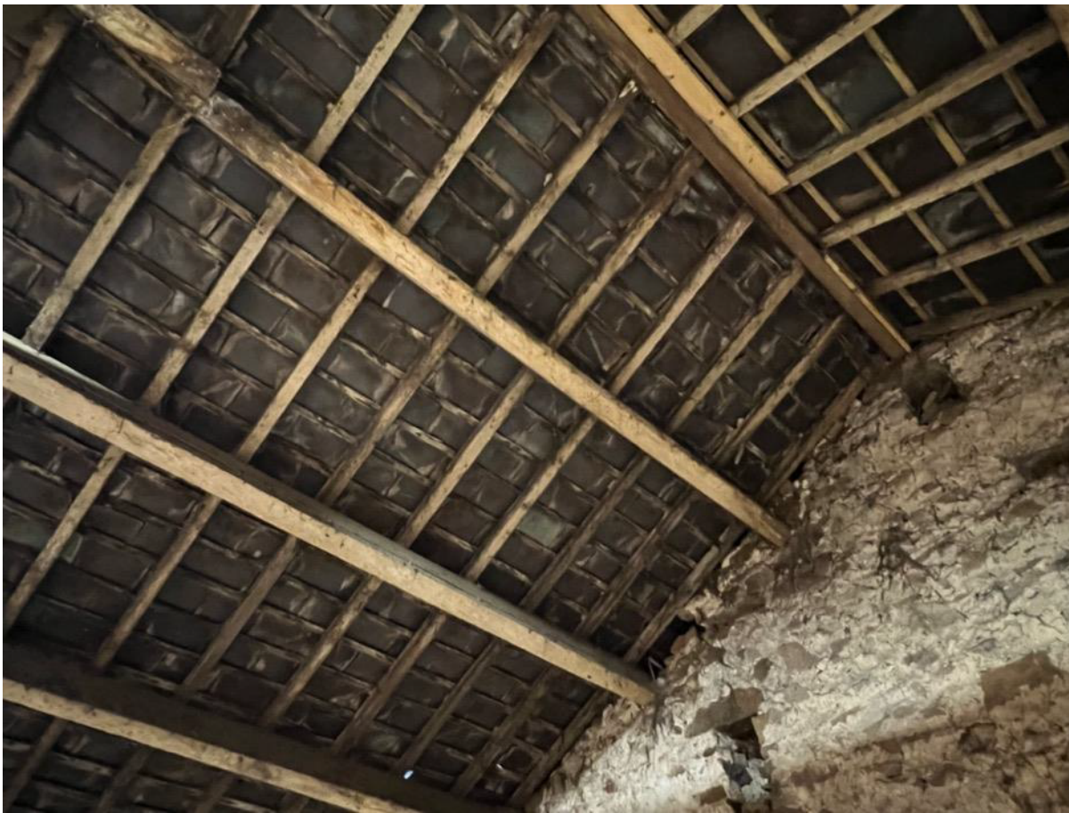
Photo 29 - Internal main barn – roof
