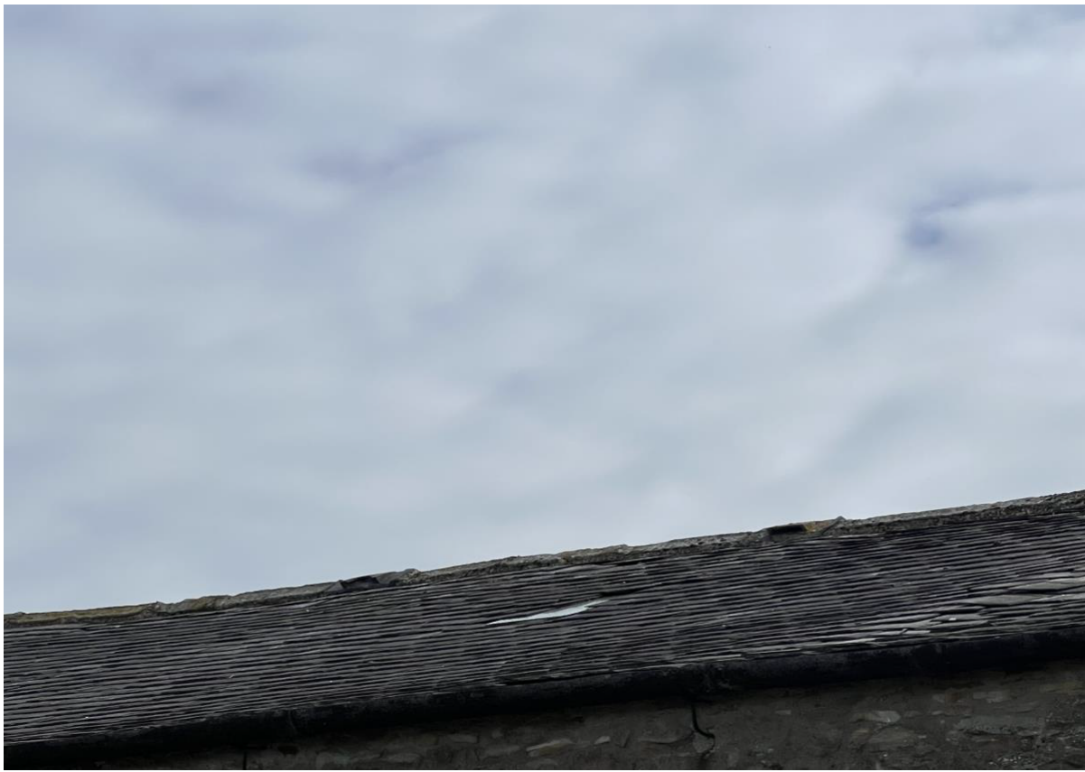
Photo 3 - Roof South West
