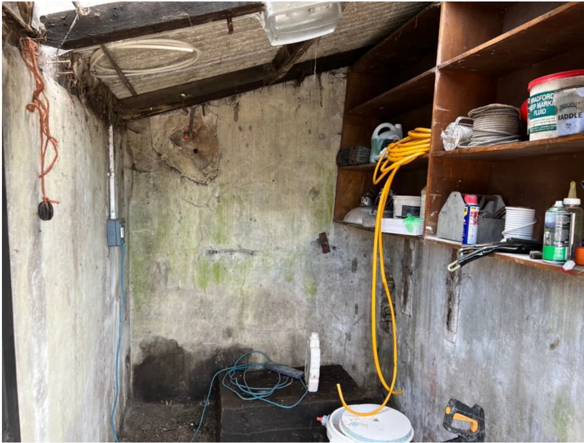
Photo 44 – Lean to on south west elevation - internal
