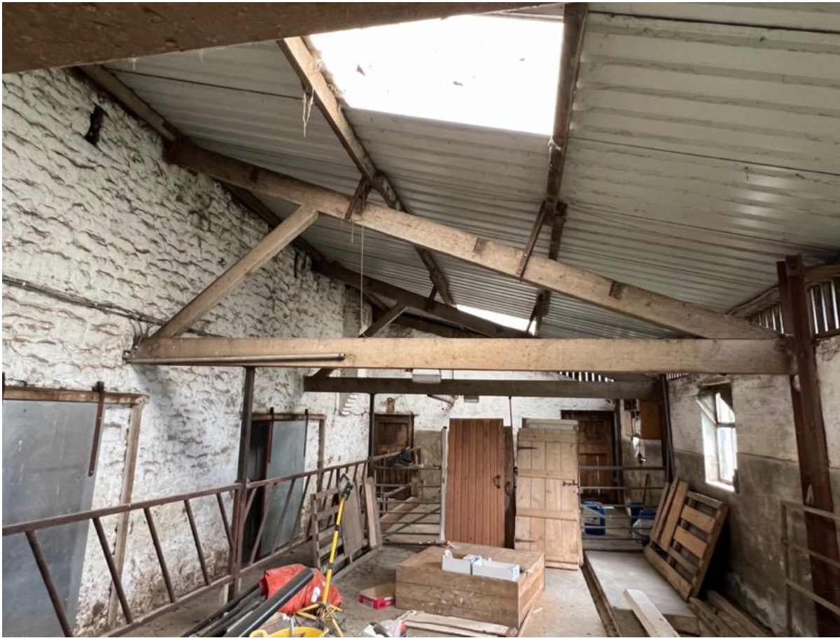
Photo 22 - Internal to rear single storey section
