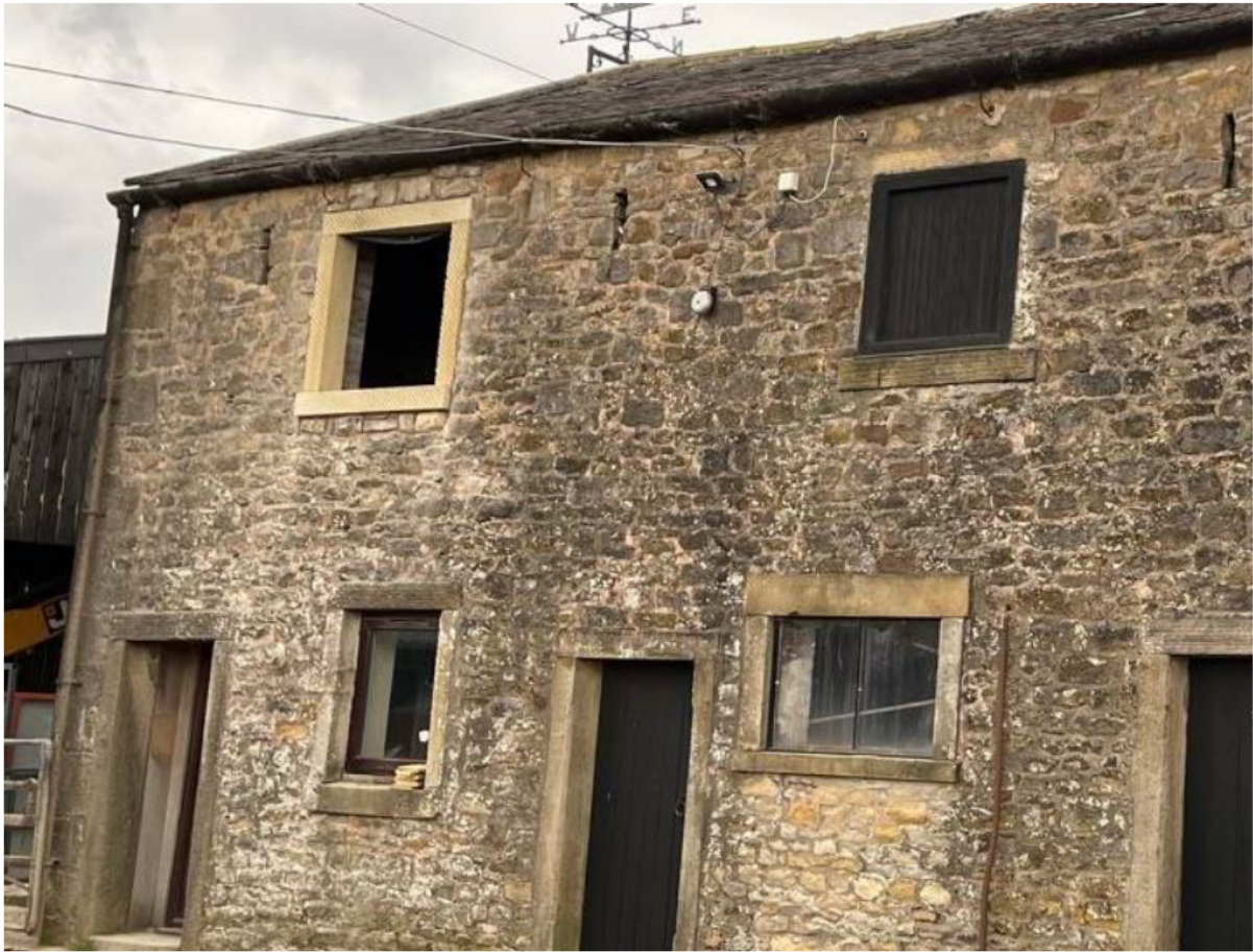
Photo 8 – South West Elevation
