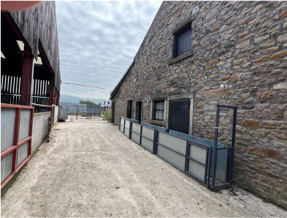
Photo 10 – North West Elevation
