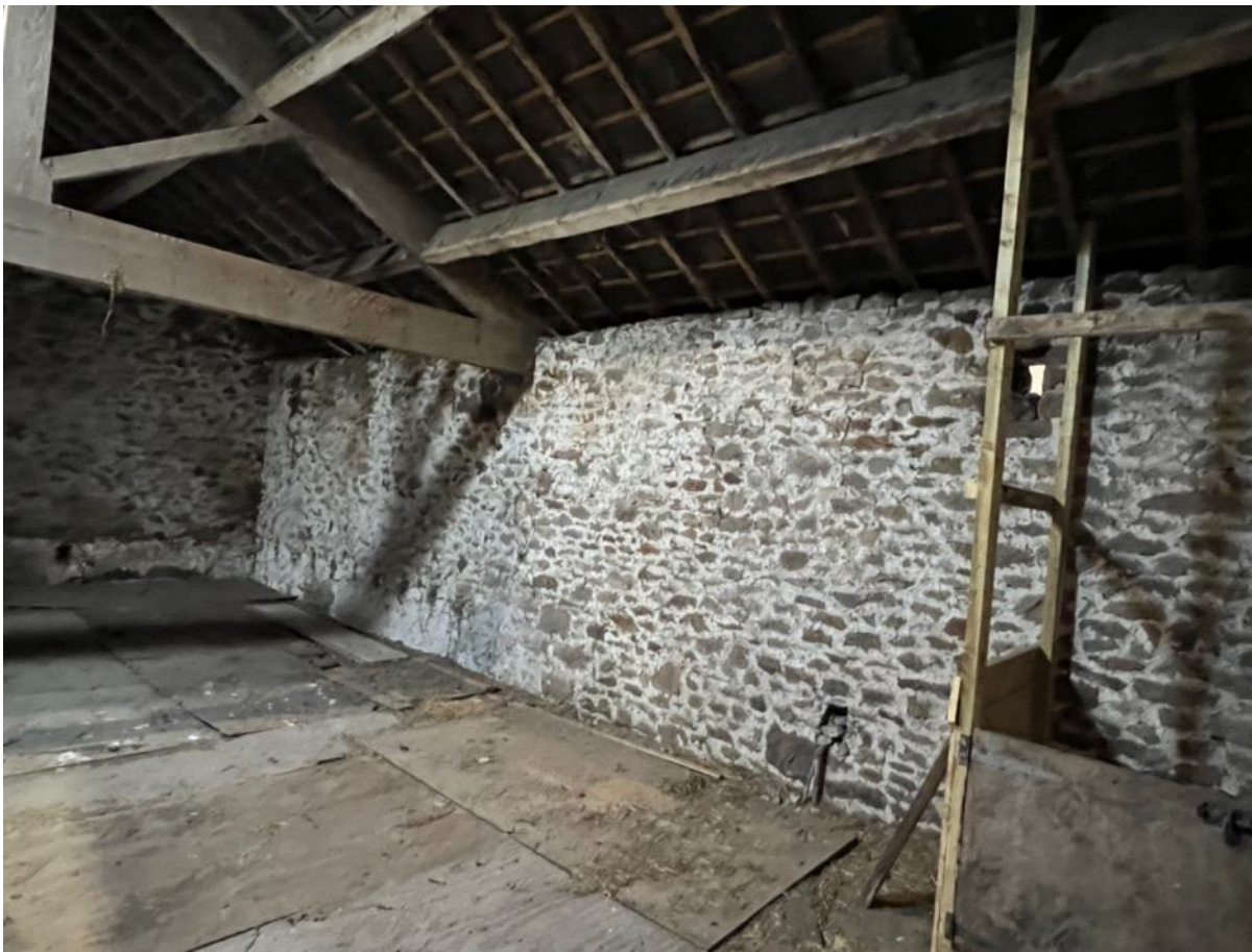
Photo 33 - Internal main barn – south west end
