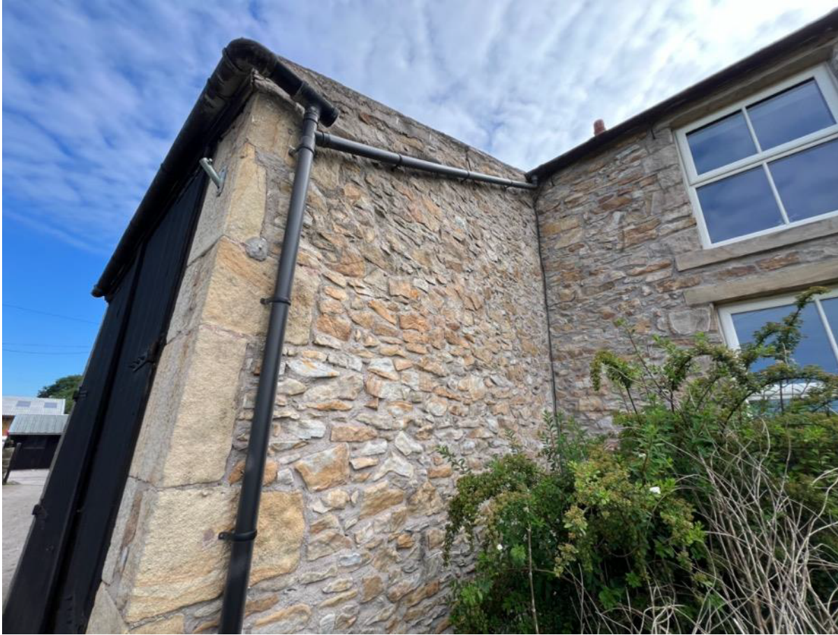
Photo 14 - South East Elevation – outrigger wall adjacent to house
