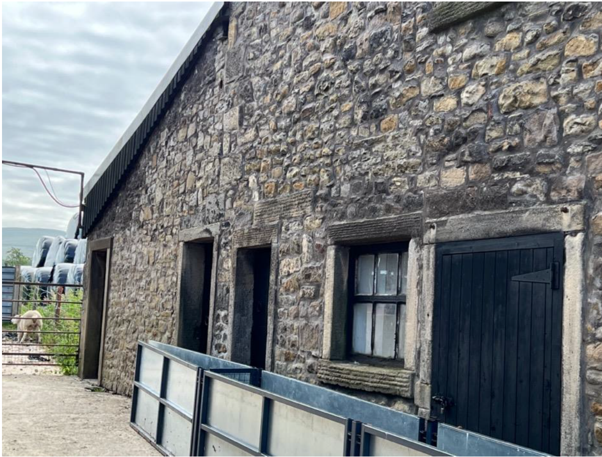
Photo 12 - North West Elevation
