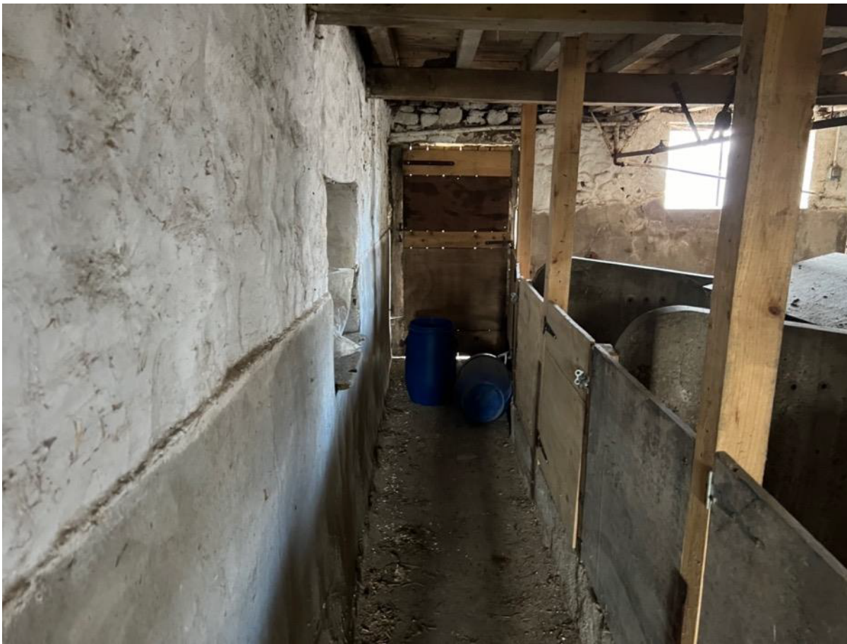
Photo 37 - Internal main barn – mid section
