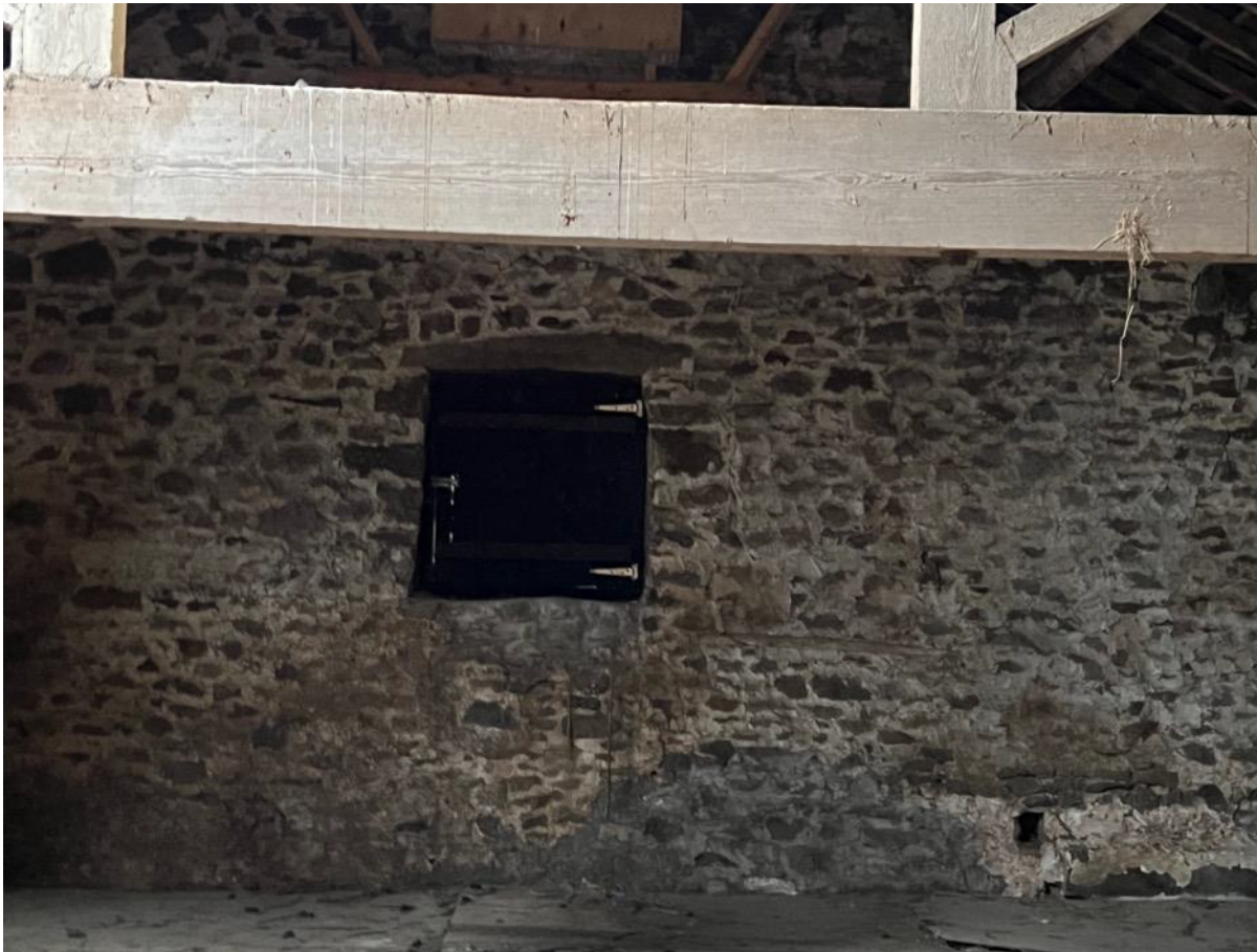
Photo 34 - Internal main barn – south west end – truss timber
