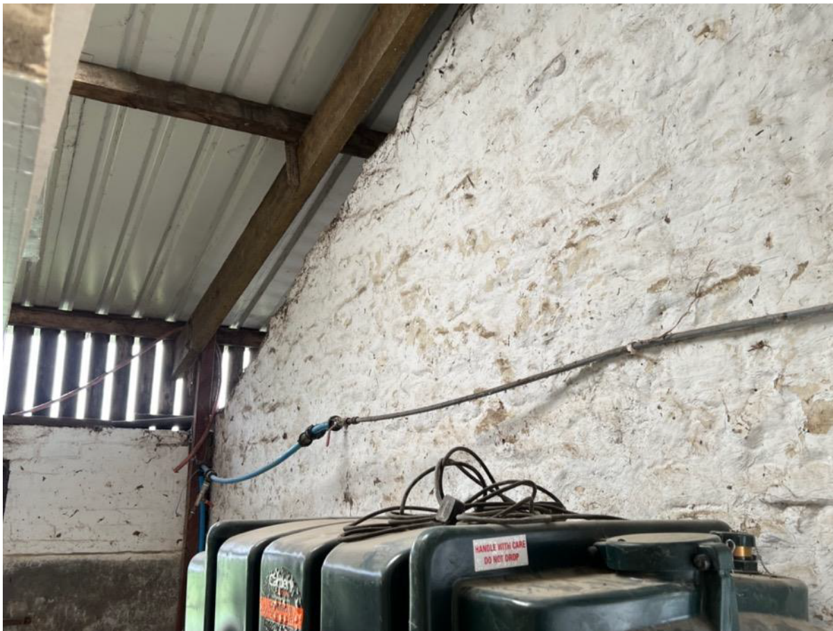
Photo 18 – Internal to rear single storey section
