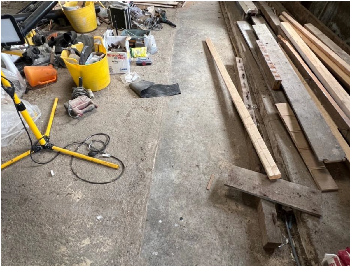
Photo 23 - Internal to rear single storey section - floor
