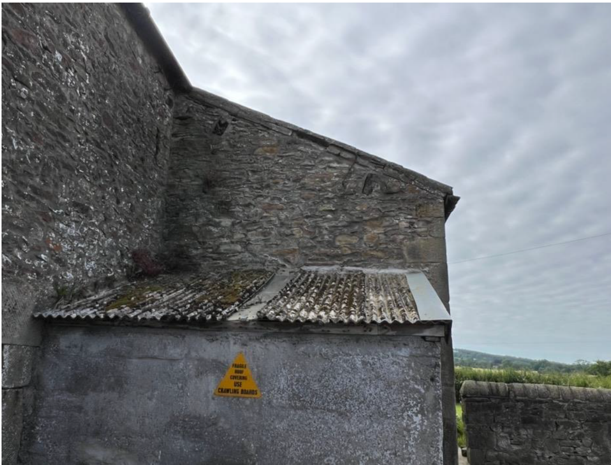
Photo 13 – Lean to on South West Elevation
