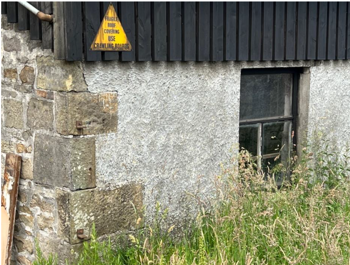
Photo 16 - North East Elevation at corner with south east elevation
