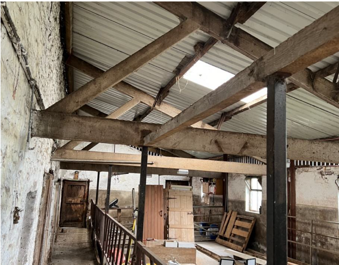
Photo 19 - Internal to rear single storey section
