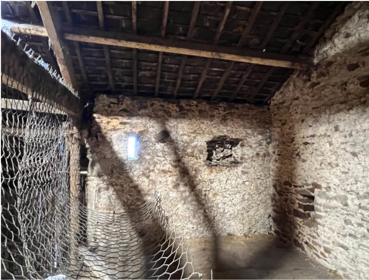
Photo 30 - Internal main barn – south east end
