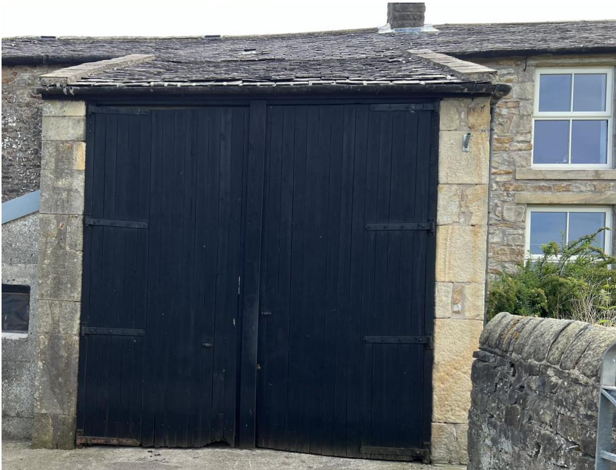
Photo 5 – South West Elevation
