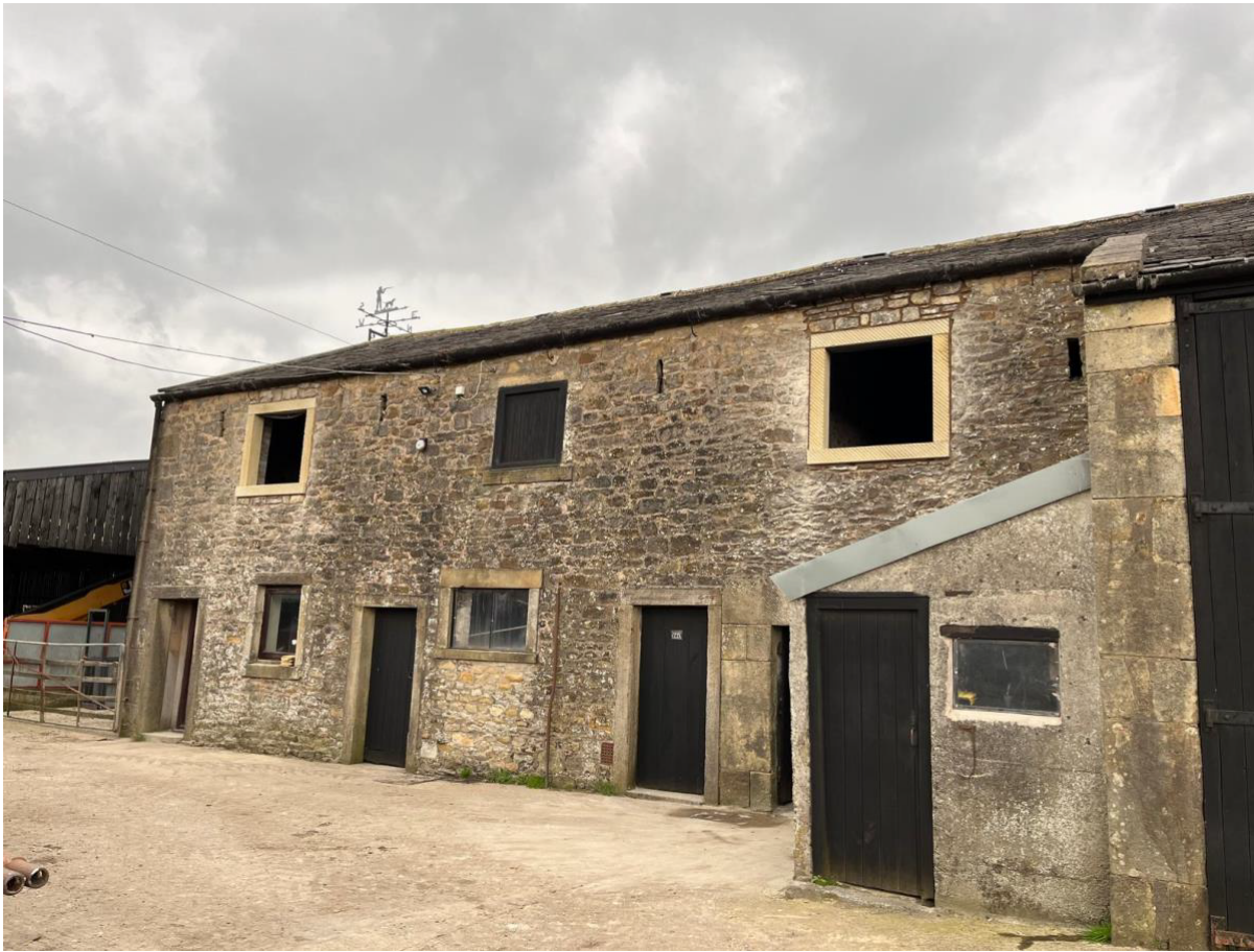
Photo 6 – South West Elevation
