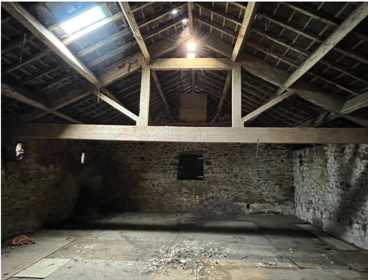
Photo 31 - Internal main barn – south west end
