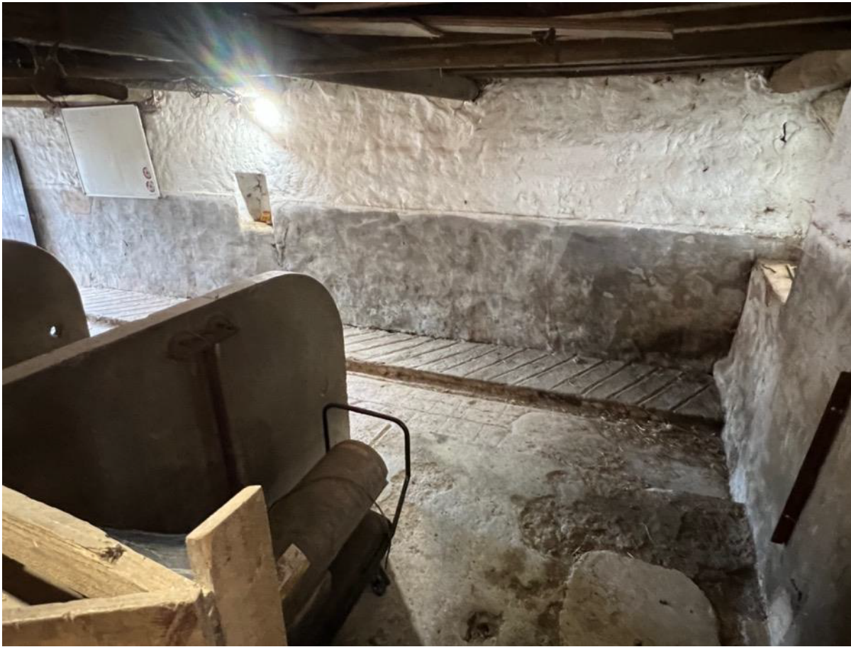
Photo 26 - Internal main barn – south east end
