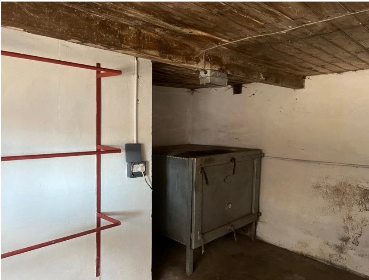
Photo 40 - Internal main barn – north west end
