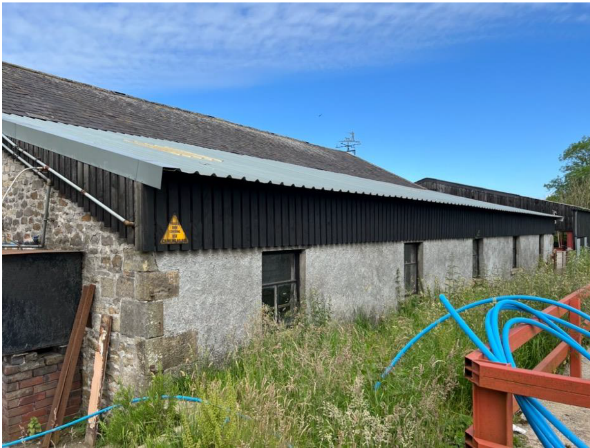
Photo 15 - North East Elevation with south east elevation
