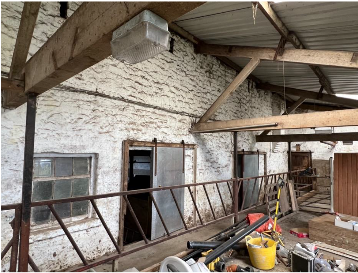
Photo 21 - Internal to rear single storey section
