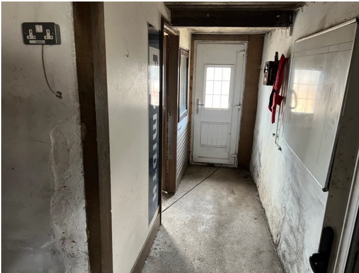
Photo 41 - Internal main barn – north west end
