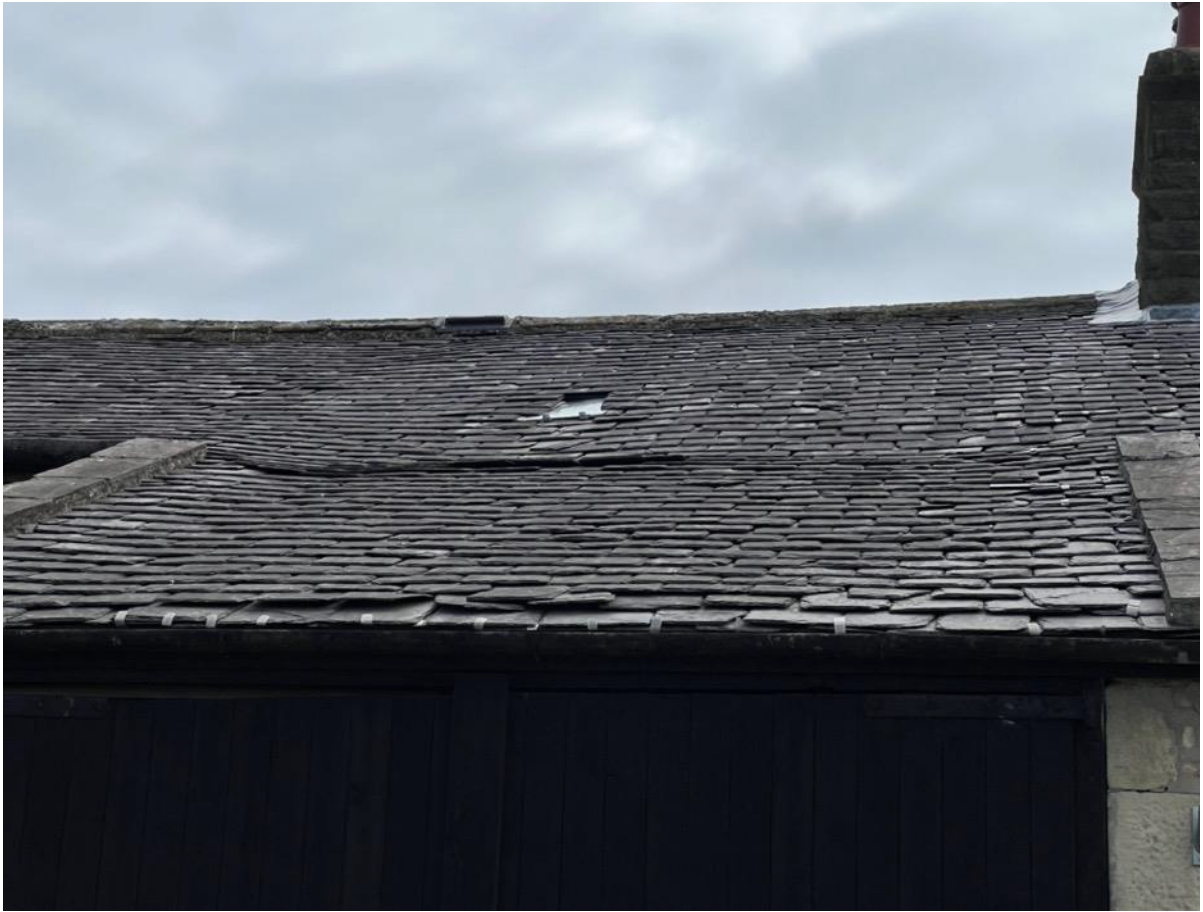
Photo 2 – Roof South West
