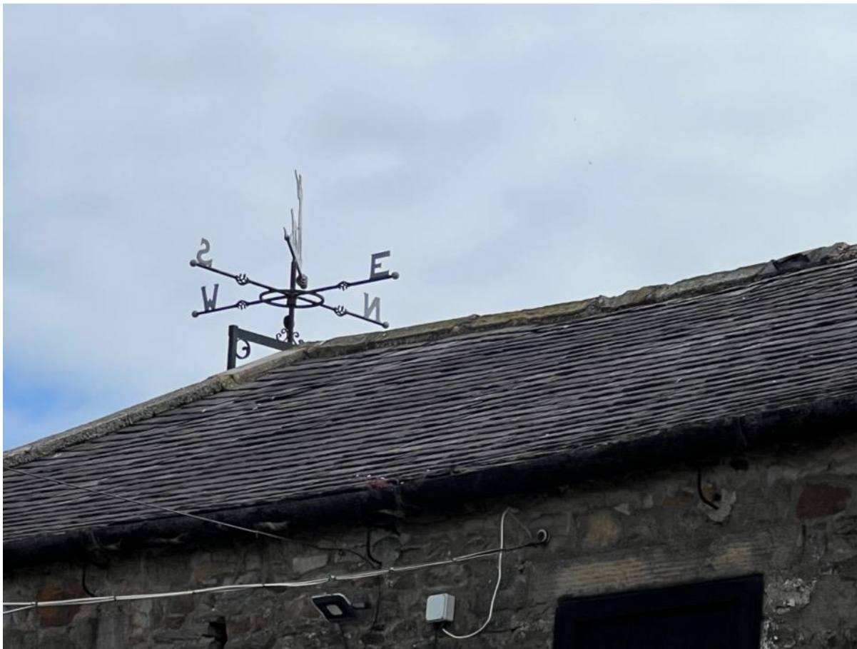
Photo 4 – Roof South West
