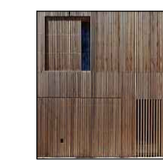
Louvered timber cladding over windows
