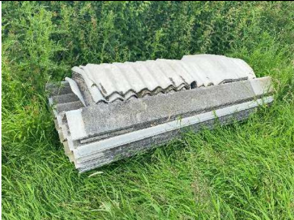
P11: Roof sheeting material used in the construction of the barn building proven to be devoid of asbestos through laboratory testing
