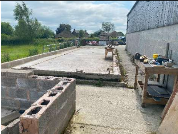
P7: View along the southern side of the barn building
