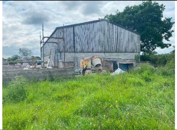
P8: View of the eastern side/gable end of the barn building
