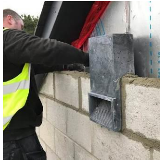
Green and Blue Bat Block/Brick in situ
